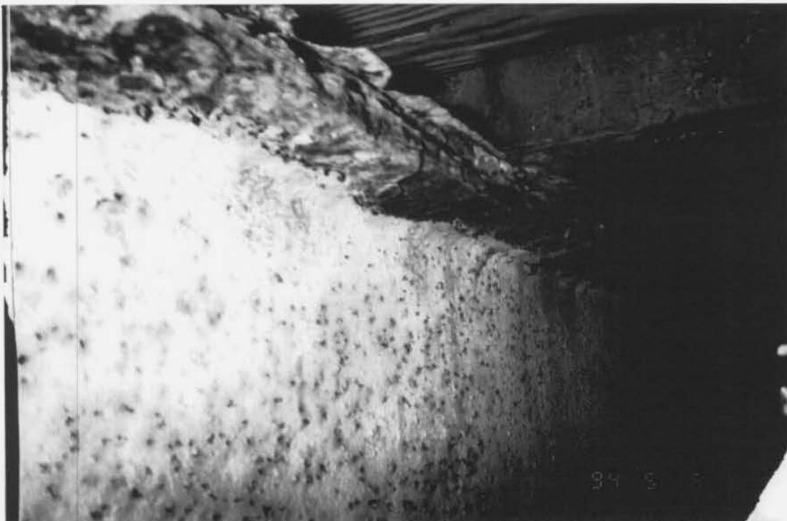
CORROSION IN FLOOR BEAM - TOP FLANGE
