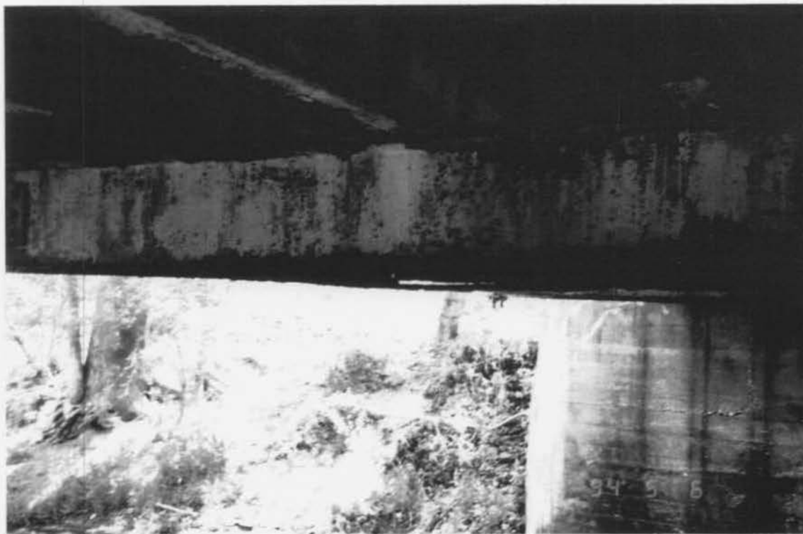
FLOOR BEAM BENT #3 - SEPARATION OF COVER PLATE
