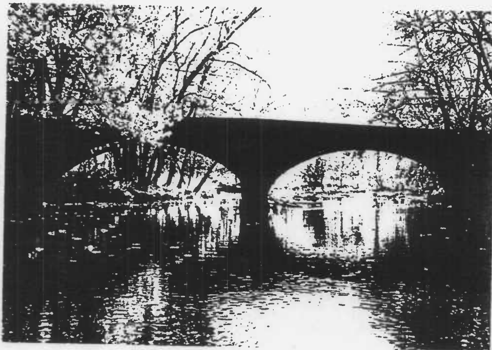
2. WEST ELEVATION (LOOKING EAST)
