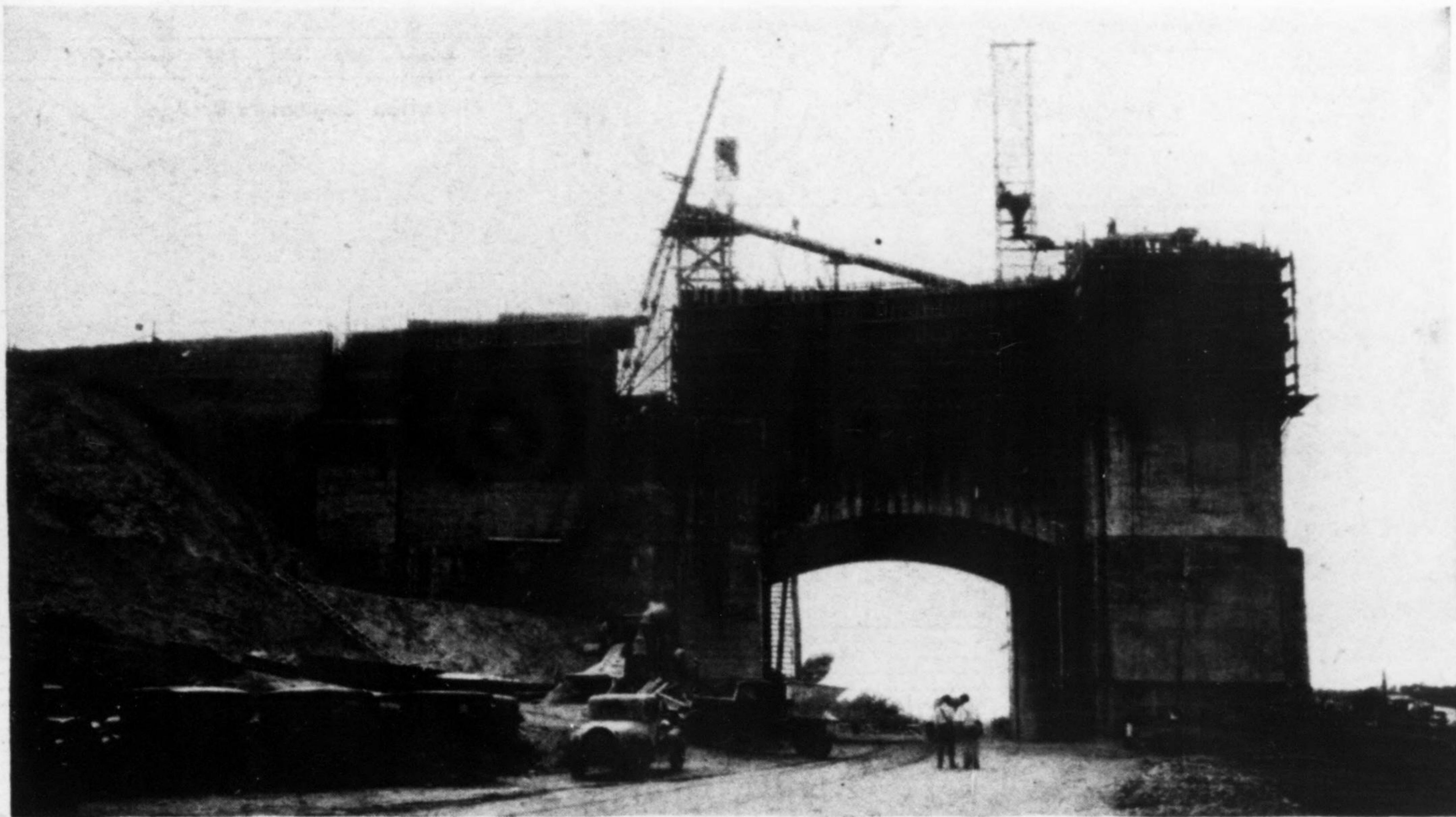
FIG. 1—CONCRETING the South Sagamore abutment with the plant units typical of the job—small tip-over-body trucks, paving mixers and a crawler crane to hoist the bottom-dump buckets. The elevator tower was required for the high pylons. Note how crane is set on an embankment to increase its reach.
