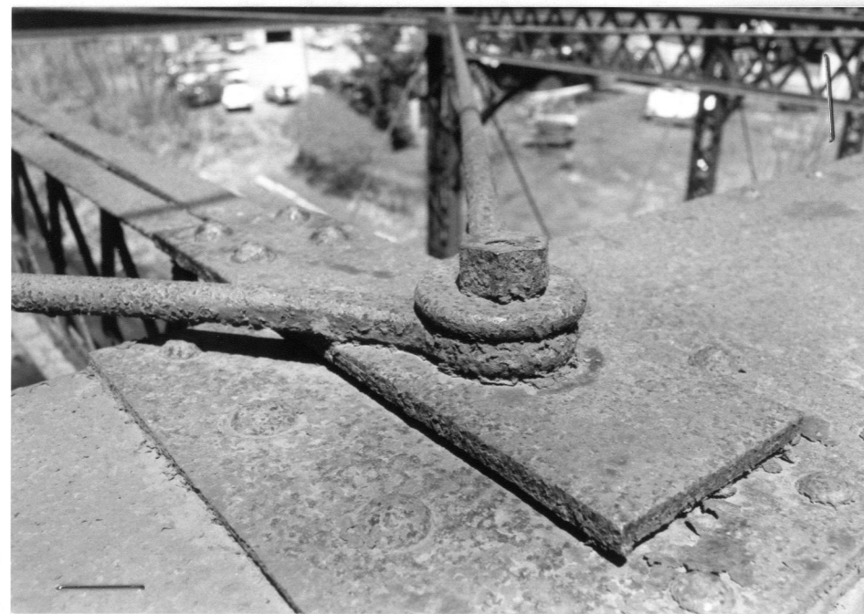
UPPER LATERAL BRACES CONNECTION TO SE UPPER CHORD AT 2ND UPPER PANEL POINT, FROM S (5-4-88)
