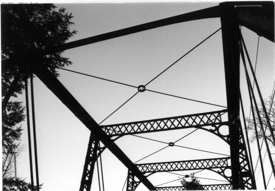
UPPER CHORDS LATERAL BRACING, AND TENSION RODS, IN 3 SOUTHWESTERN PANELS, FROM SW (4-25-85)
