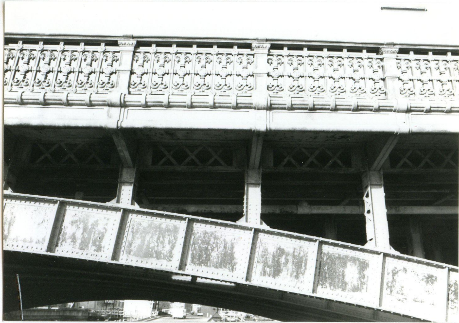
WESTERN MOST ARCH, SOUTHERN FACE, FROM S
