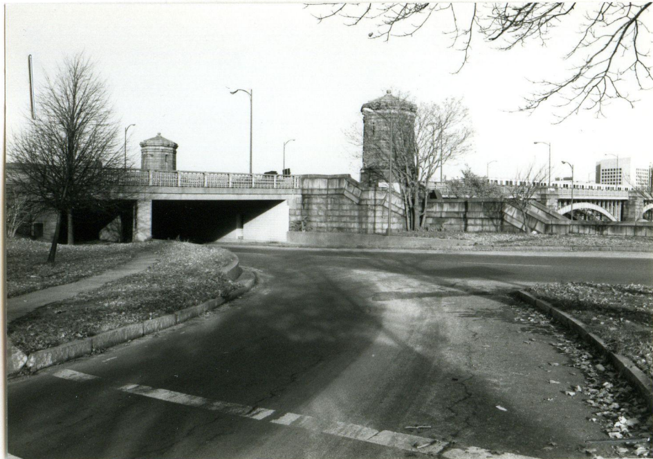
WESTERN END, FROM SW
