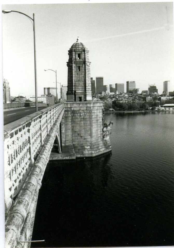
S TOWER ON PIER 6, FROM W
