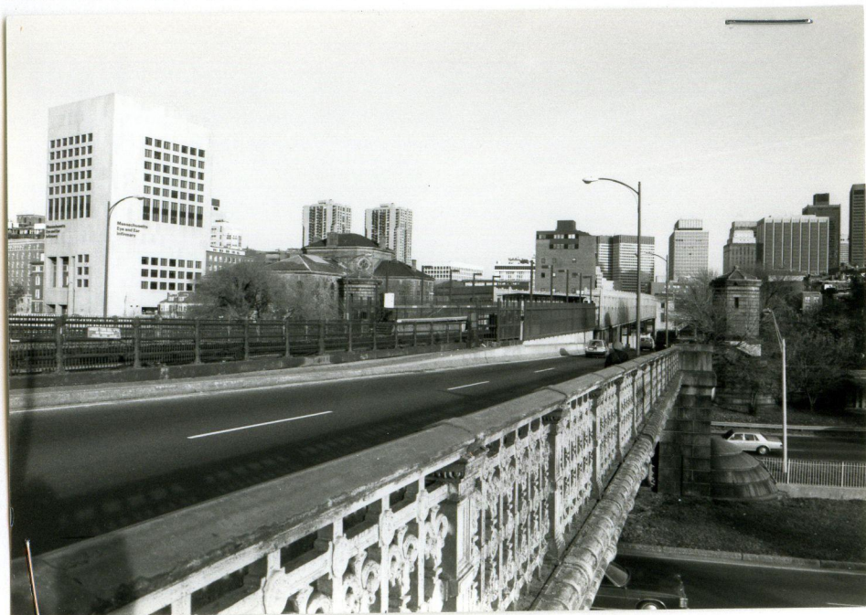
EASTERN END OF BRIDGE, LOOKING E. FROM NEAR PIER 2
