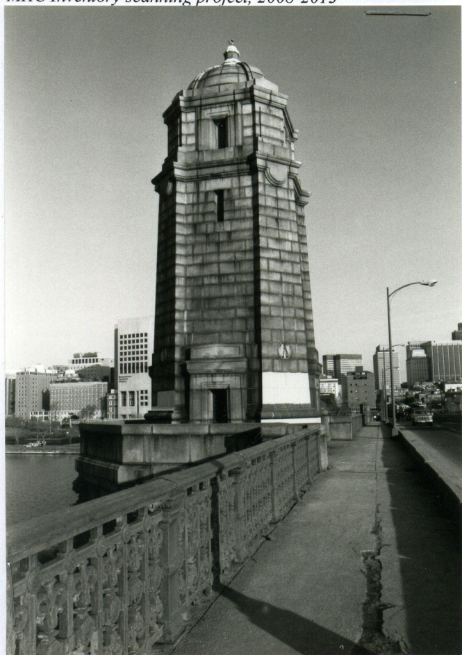
N TOWER, PIER 5, FROM W
