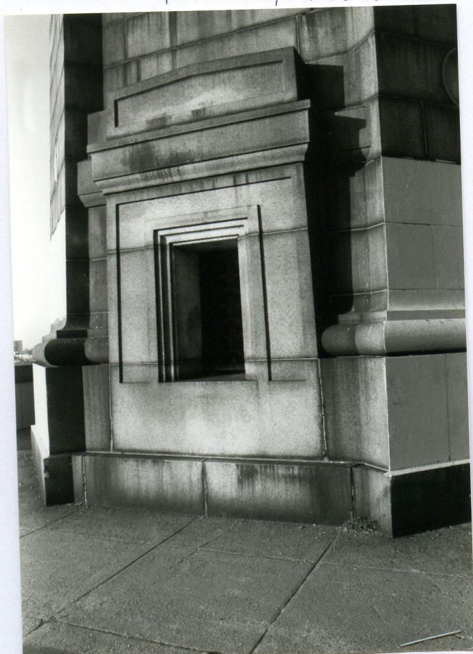
N TOWER, PIER 5, S WINDOW, FROM SE
