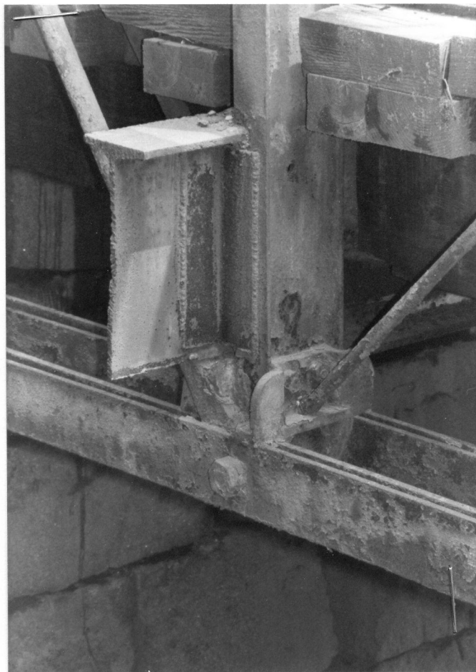
ALL: WESTERN TRUSS, INTERMEDIATE LOWER PANEL POINT (3/6/1986)
