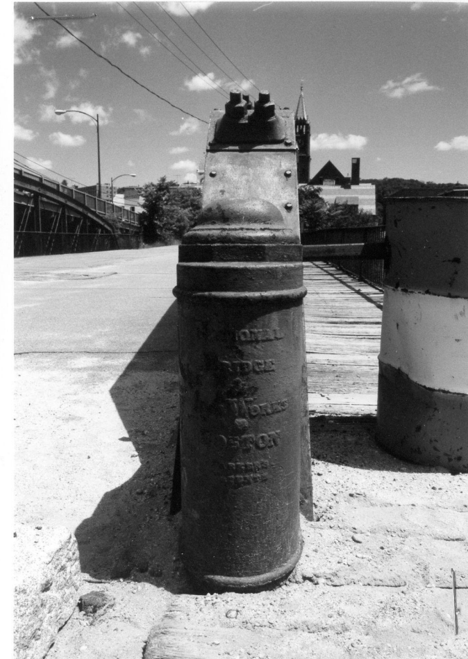
BOLLARD/PLAQUE ABOVE SKEWBACK, 3 END OF E TRUSS 6/22/1984
