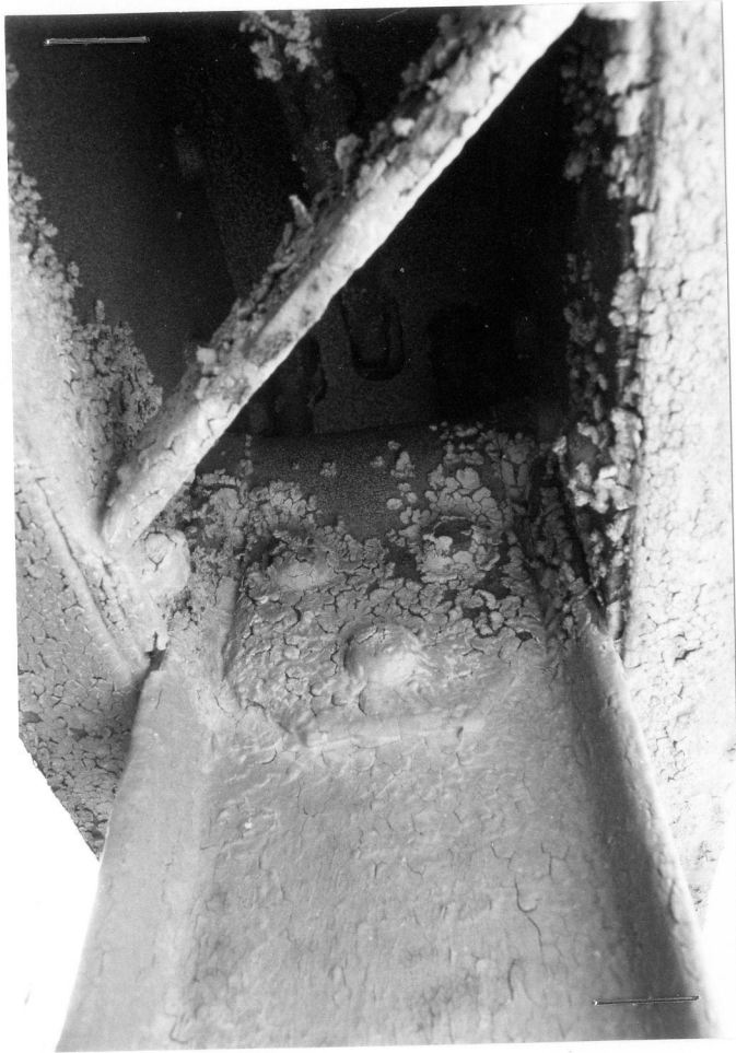
PATENTED COMPRESSION MEMBER, LOOKING UP INSIDE UPPER CHORD 6/22/1984
