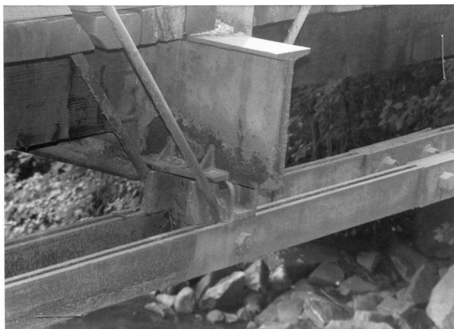
ALL: WESTERN TRUSS, INTERMEDIATE LOWER PANEL POINT (3/6/1986)
