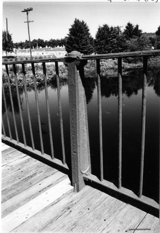
N TRUSS, UPPER CHORD INTERMEDIATE PANEL POINT CASTING (7-11-85)
