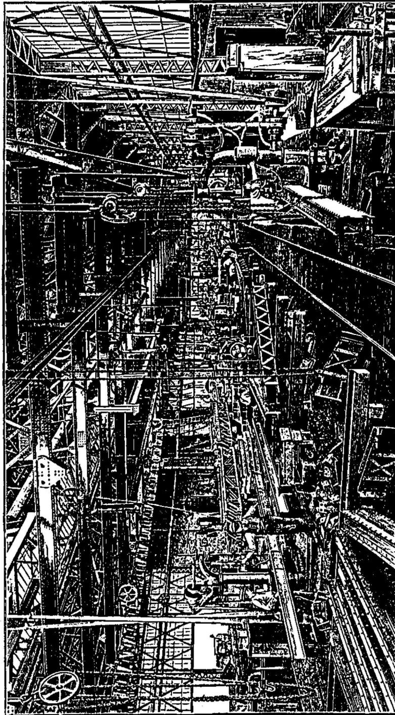
A well-appointed bridge shop of the 1890s. The 80-by-400-foot building—itsself presumably a product of the firm's works—was entirely of iron and glass with no wood used. The capacity was 1,000 tons of finished work per month. (Berlin Iron Bridge Company, East Berlin, Connecticut)
