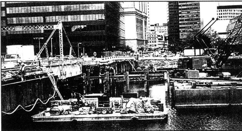
*The Summer Street Bridge was kept open to both pedestrian and vehicular traffic during renovation, all of which was staged from barges.*
