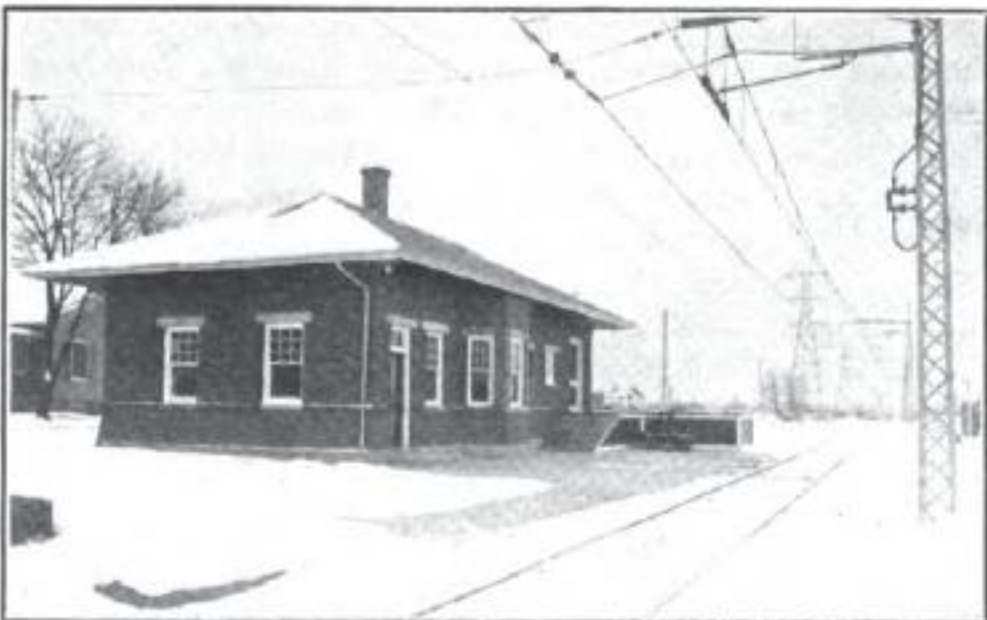
MICHIGAN 2400-VOLT LINE—STANDARD BRICK AND WOODEN WAITING STATIONS
