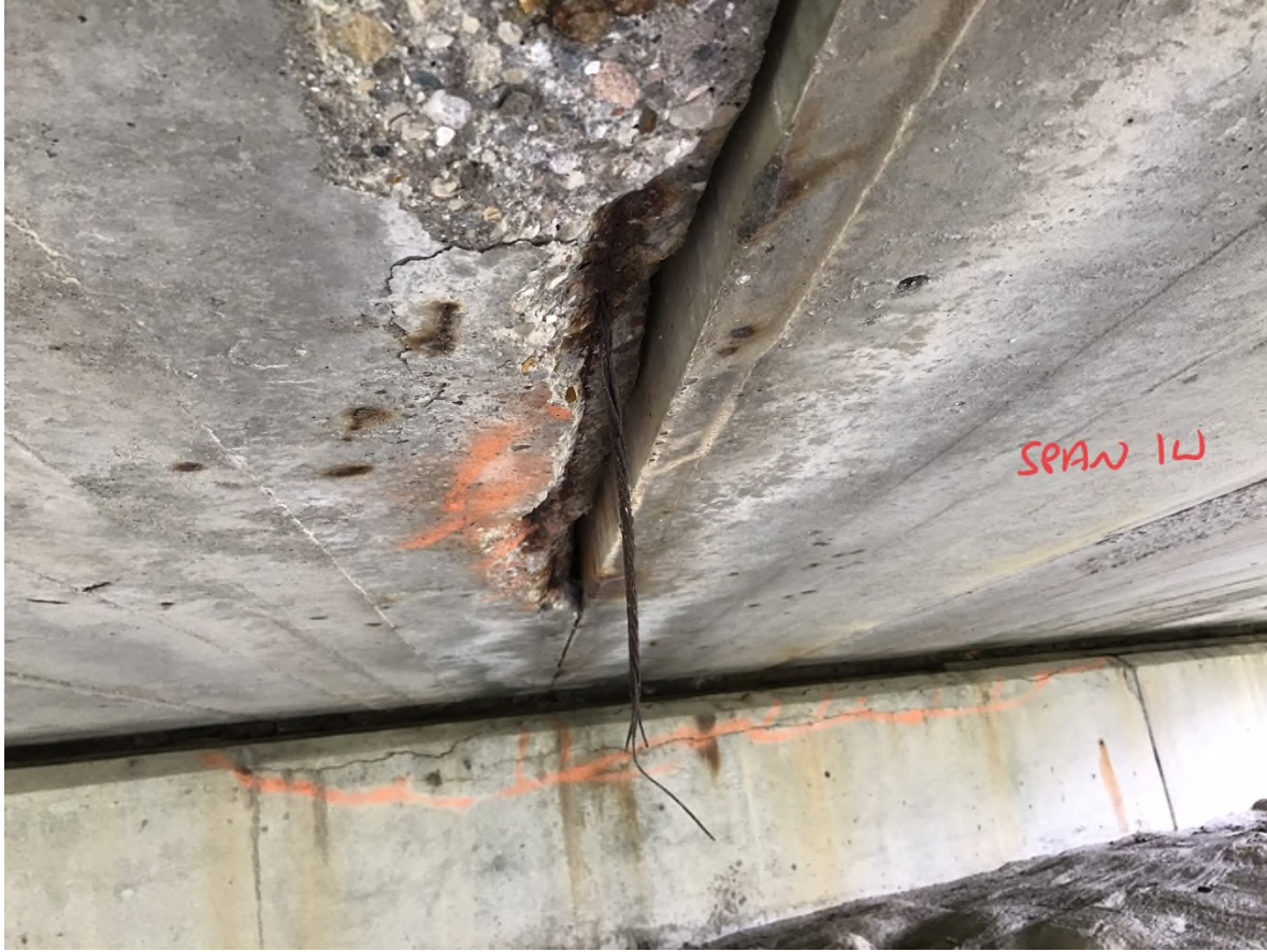
Photo 4—Detail of the underside of the bridge showing a broken and exposed beam reinforcing strand.
