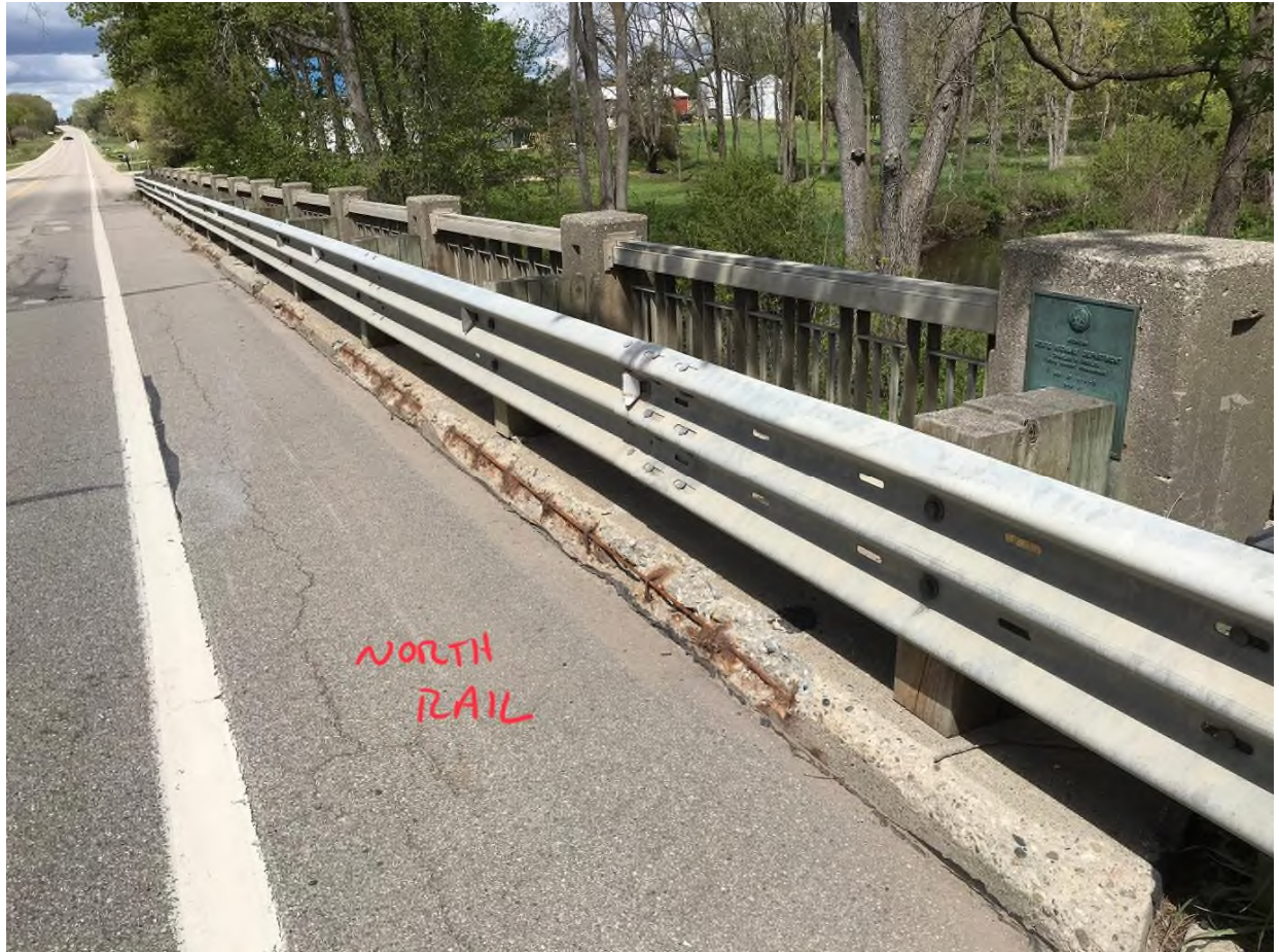
Photo 5—North railing and spalled brush block.
