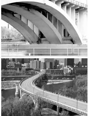
Feature 1. Melan-system reinforced-concrete arches. The Melan system, patented in 1894, uses steel Ibeams bent approximately to the shape of the arch axis and laid in a parallel series near the undersurface of the arch. The Third Avenue Bridge has seven large Melan arches, including two barrel arches and five three-rib arches, including the example in this photograph. It is considered to be the last major reinforced-concrete bridge constructed in the Twin Cities using the Melan system.
