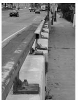
Figure 4. Looking north at the east vehicular railing on the north approach. Settlement has led to shifting of the barrier both vertically and laterally.
