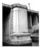
Feature 3. Classical Revival aesthetic treatment. A gateway structure, the Third Avenue Bridge received a Classical Revival aesthetic treatment. Classical elements include piers and the projecting pedestrian bays, which were restored or reconstructed in the 1979-80 deck-replacement project, and the 1939 ornamental railing.
