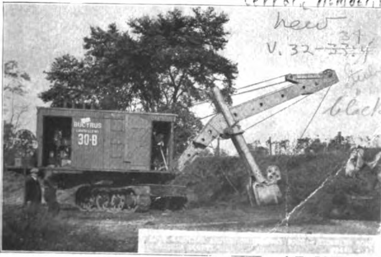
On Highway Work, Widening Roadway in Waukesha County, Wis.
