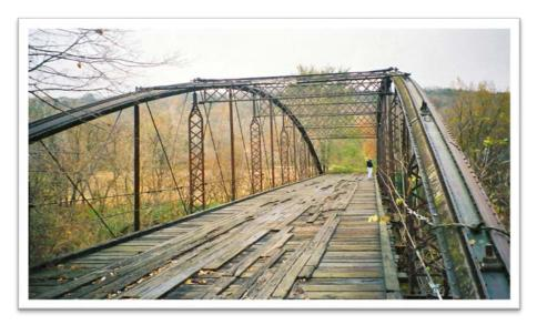
The Kern (Yaeger) Bridge is a single-span, wrought-iron, bowstring arch through truss resting on limestone abutments. Until February 6, 2020, the bridge was located in Blue Earth County connecting Mankato and South Bend Townships spanning the Le Sueur River. It was constructed by John Mahowald and the Wrought Iron Bridge Company in 1873.
