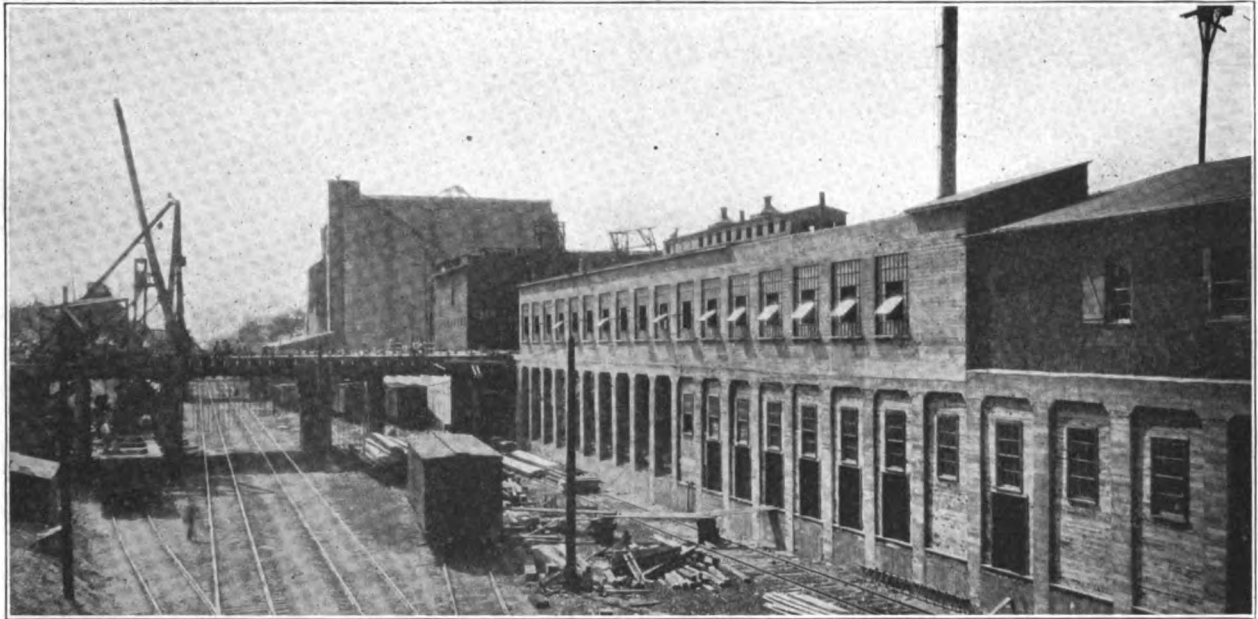
C. M. & St. P. Ry. Track Depression In Minneapolis, Fig. 6—Grand Ave. Bridge Under Construction; Concrete Underpinning of Plant of Western Crucible Steel Castings Co.
