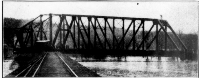
The Draw Span in the Open Position
