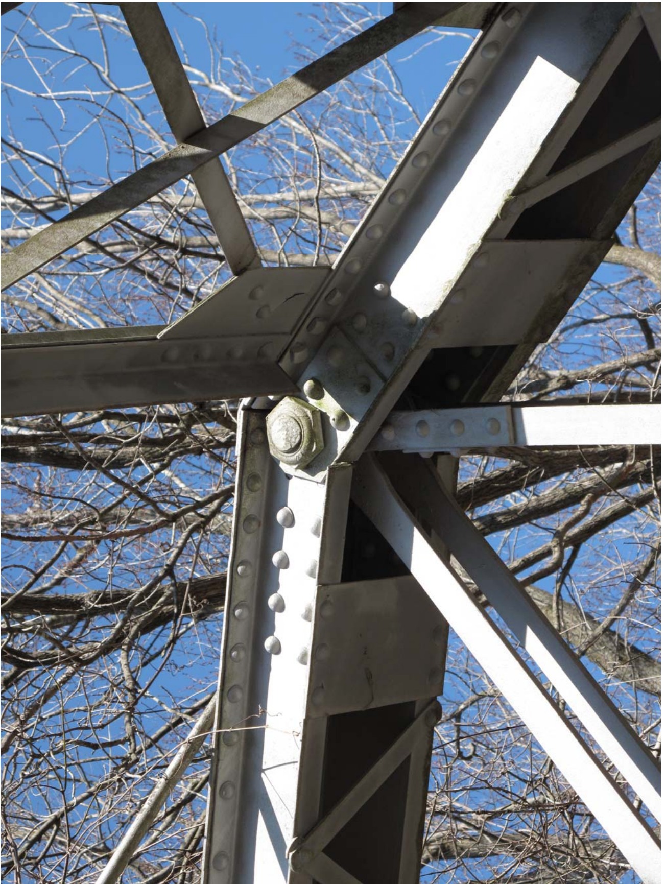
#14 of 40. Bridge W0304. Upper hip vertical pin connection. View to north.
