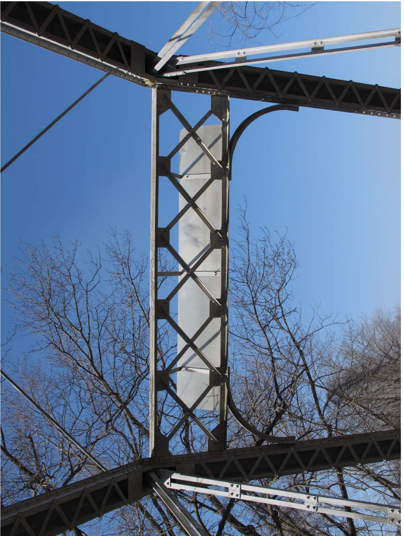
#13 of 40. Bridge W0304. West portal bracing. View to west.
