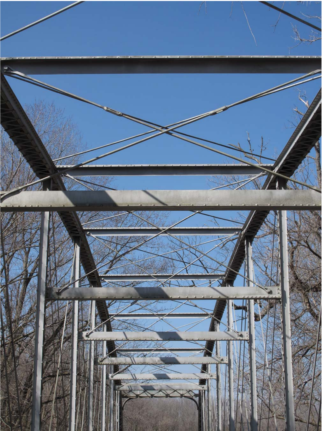
#10 of 40. Bridge W0304. Sway bracing. View to west.
