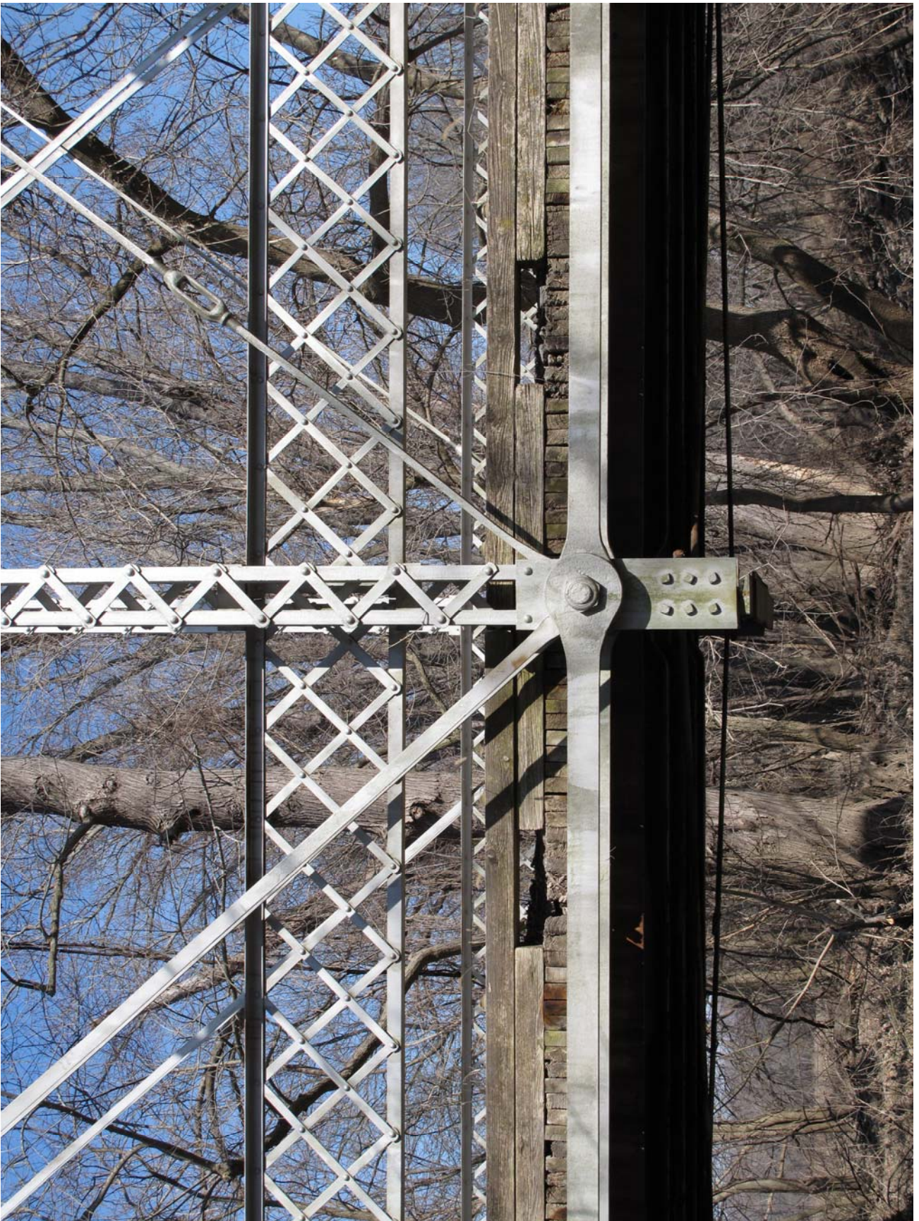
#35 of 40. Bridge W0304. Lower pin connection. View to north.
