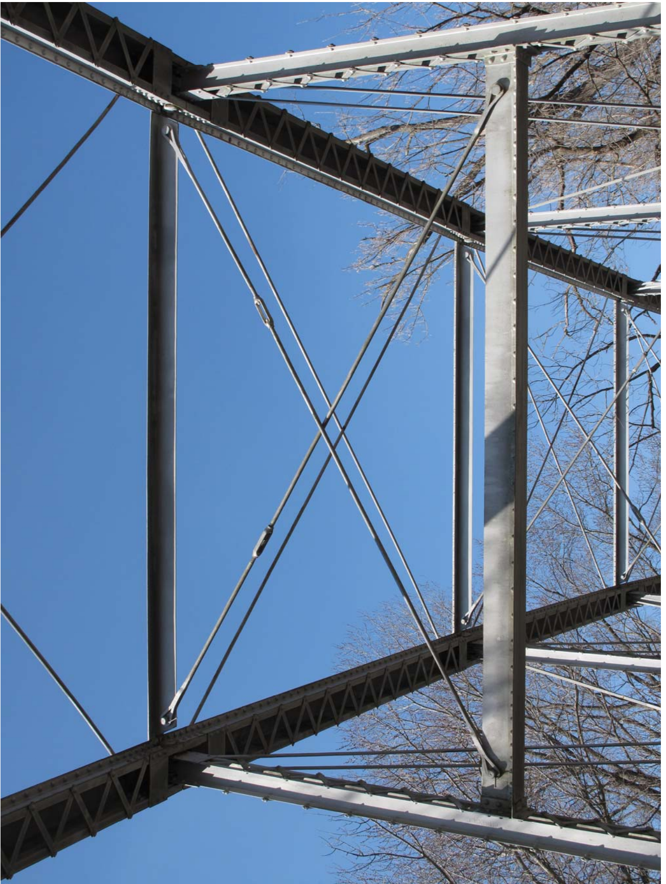
#12 of 40. Bridge W0304. Sway bracing detail. View to west.
