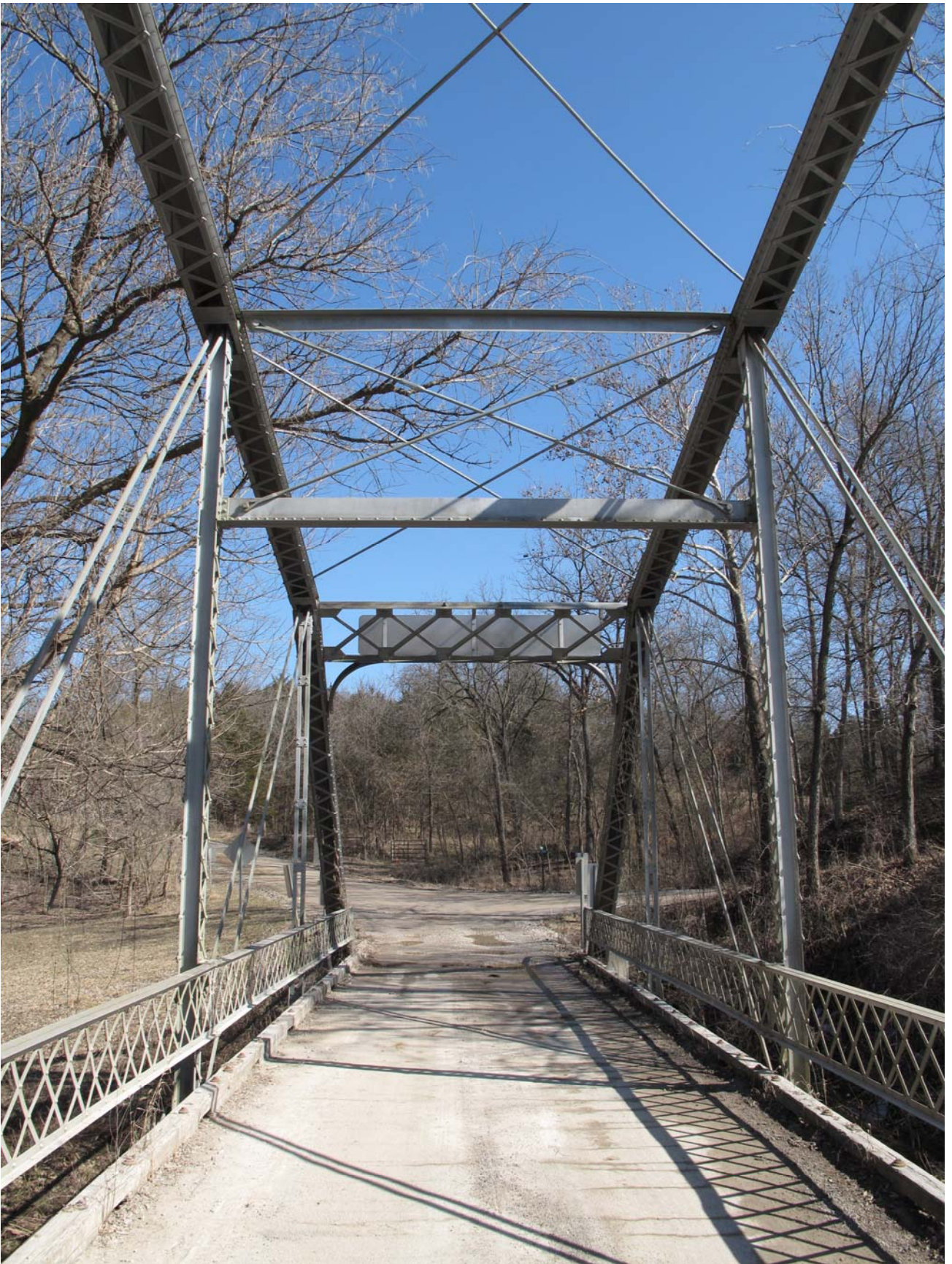
#28 of 40. Bridge W0304. Sway bracing. View to east.
