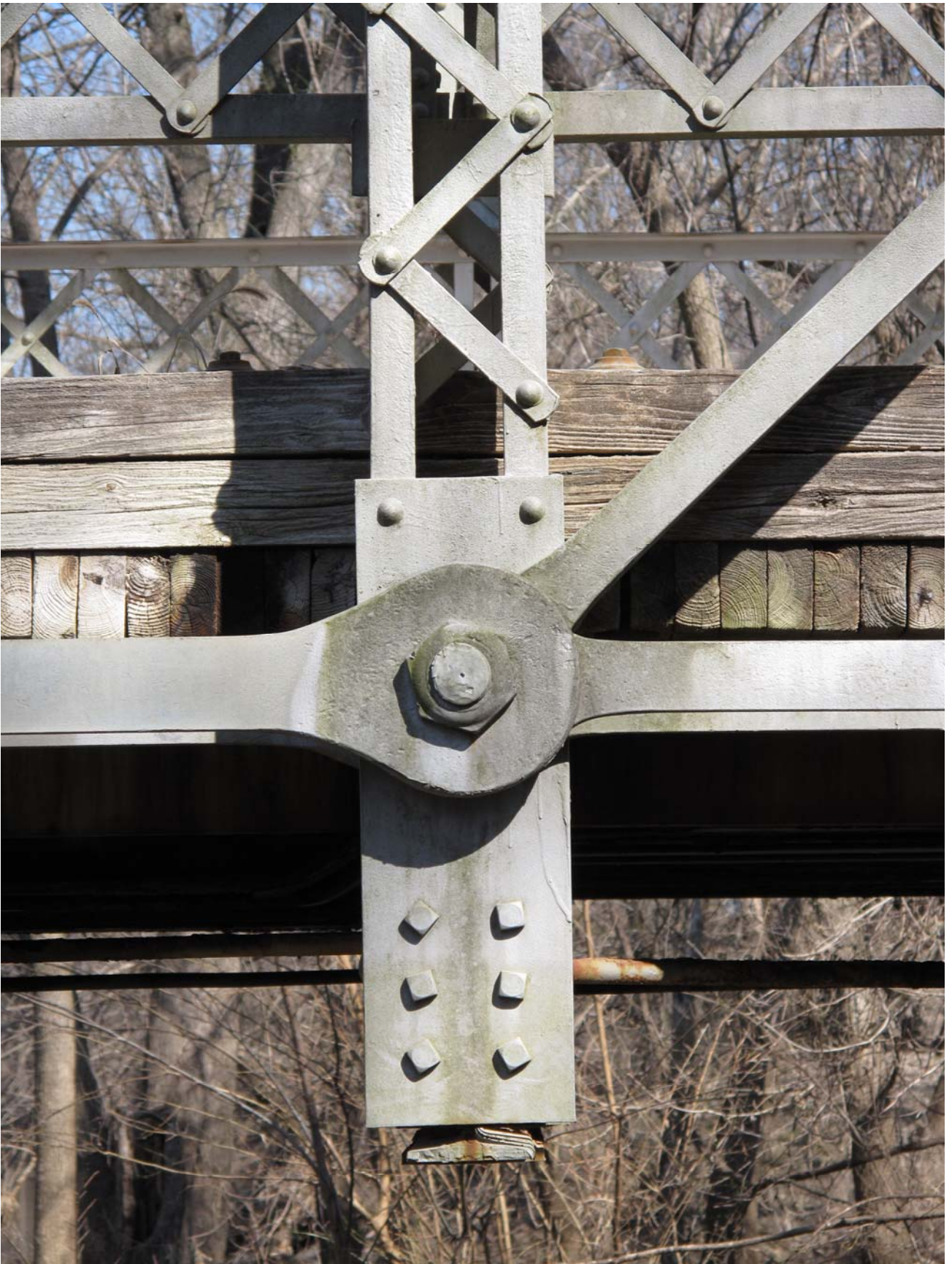
#36 of 40. Bridge W0304. Pin connection detail. View to north.
