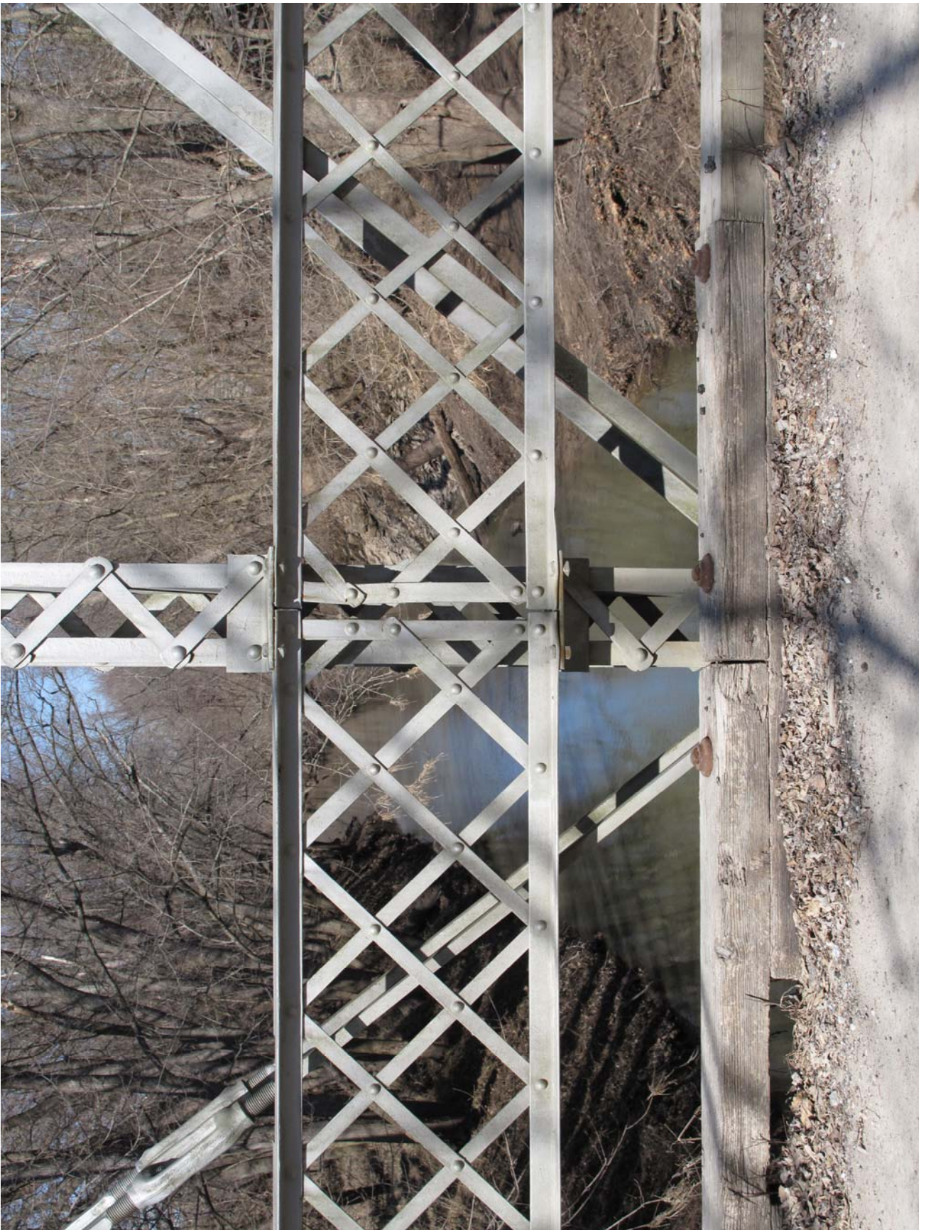
#18 of 40. Bridge W0304. Lattice guardrail. View to north.
