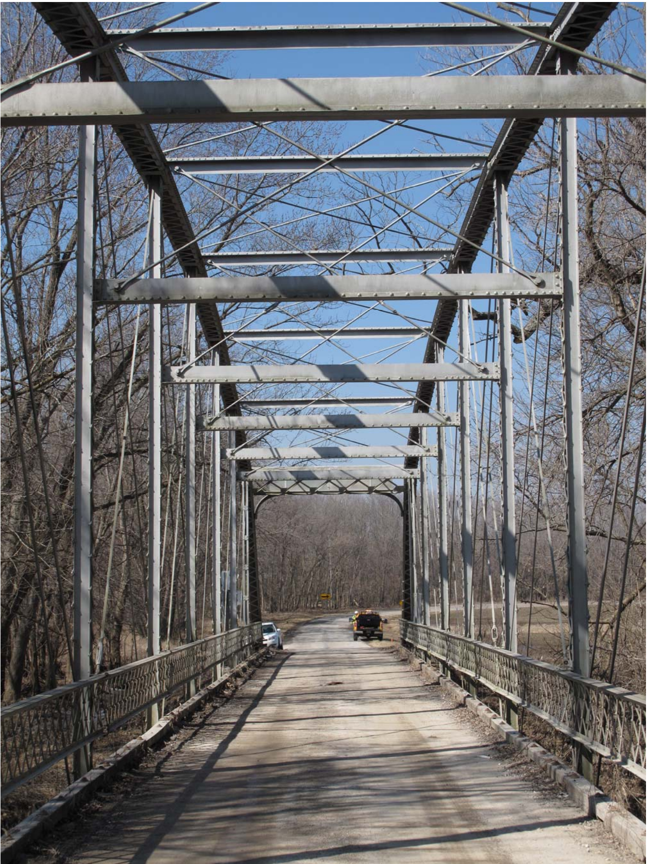
#11 of 40. Bridge W0304. Sway bracing. View to west.
