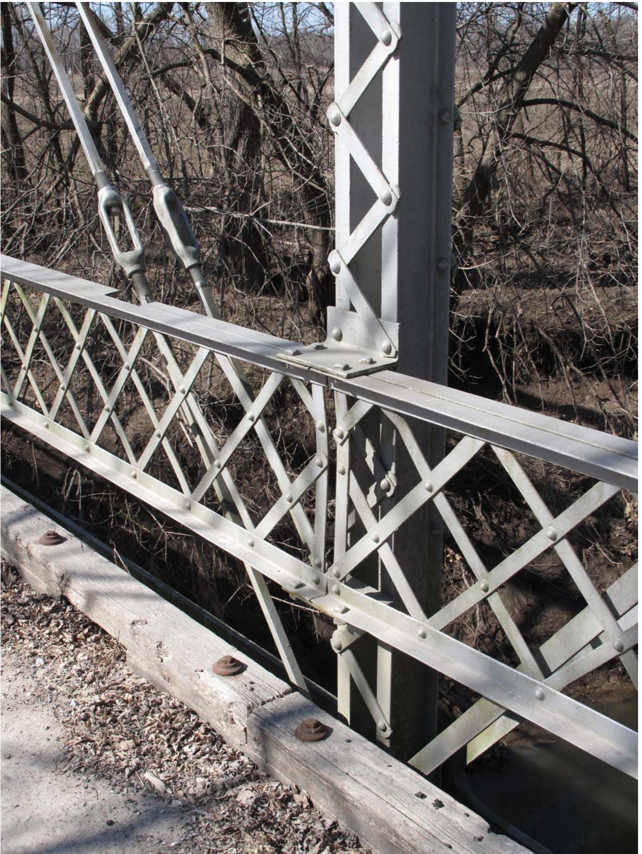
#17 of 40. Bridge W0304. Lattice guardrail. View to northwest.
