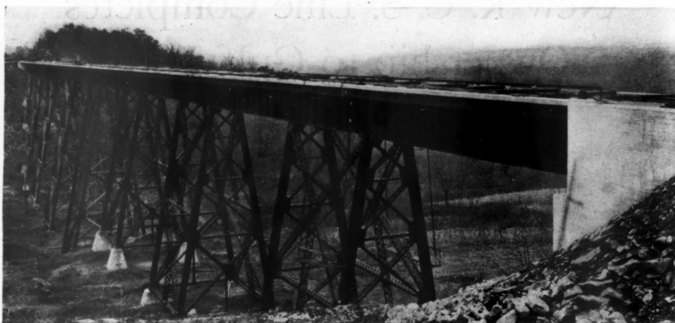
A View of the Steel Viaduct on Mile 14 Complete Except for Handrails, Ballast and Track
