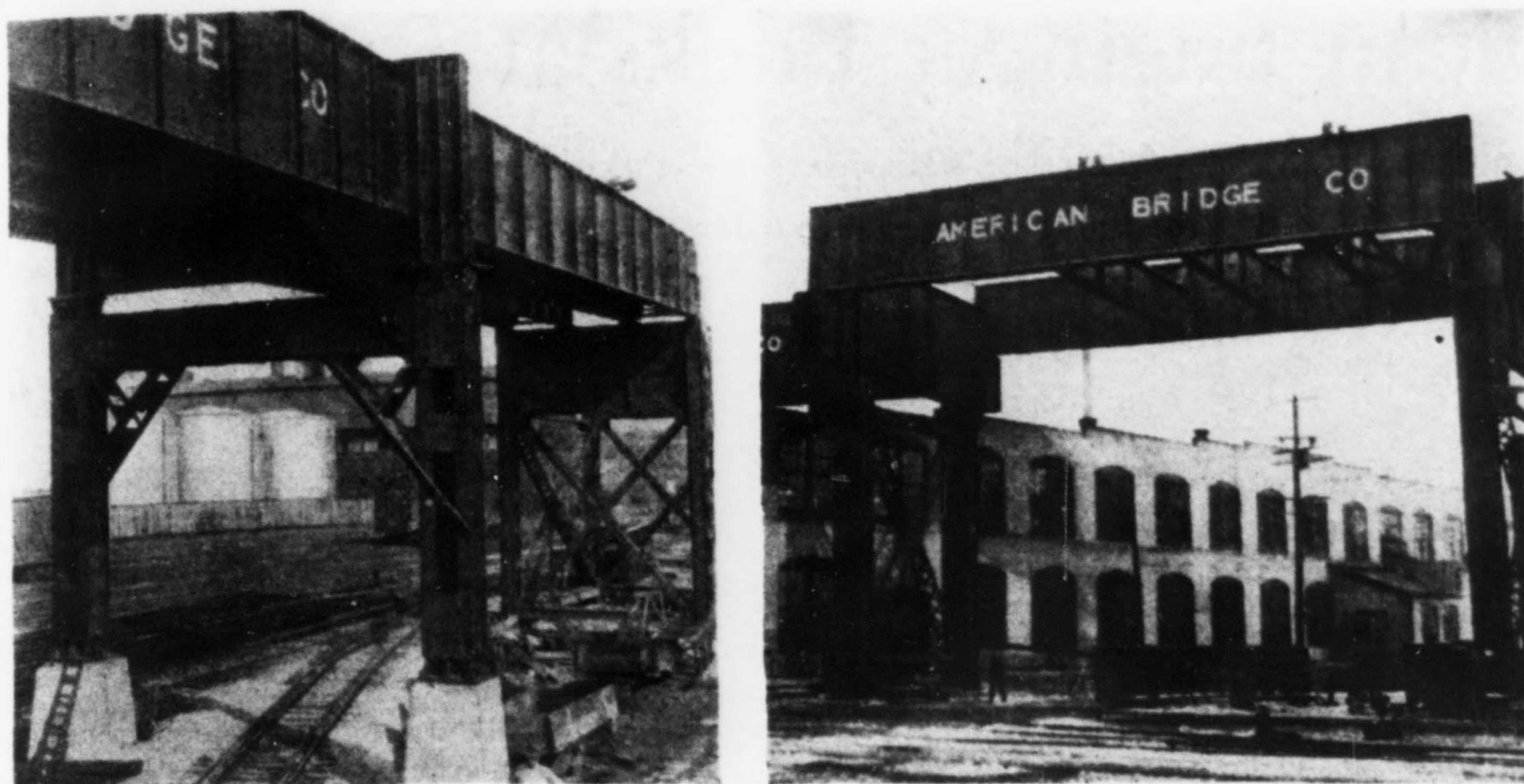
FIG. 5—PIN-CONNECTED VIADUCT BENTS Note cantilever ends of cross-girders.
