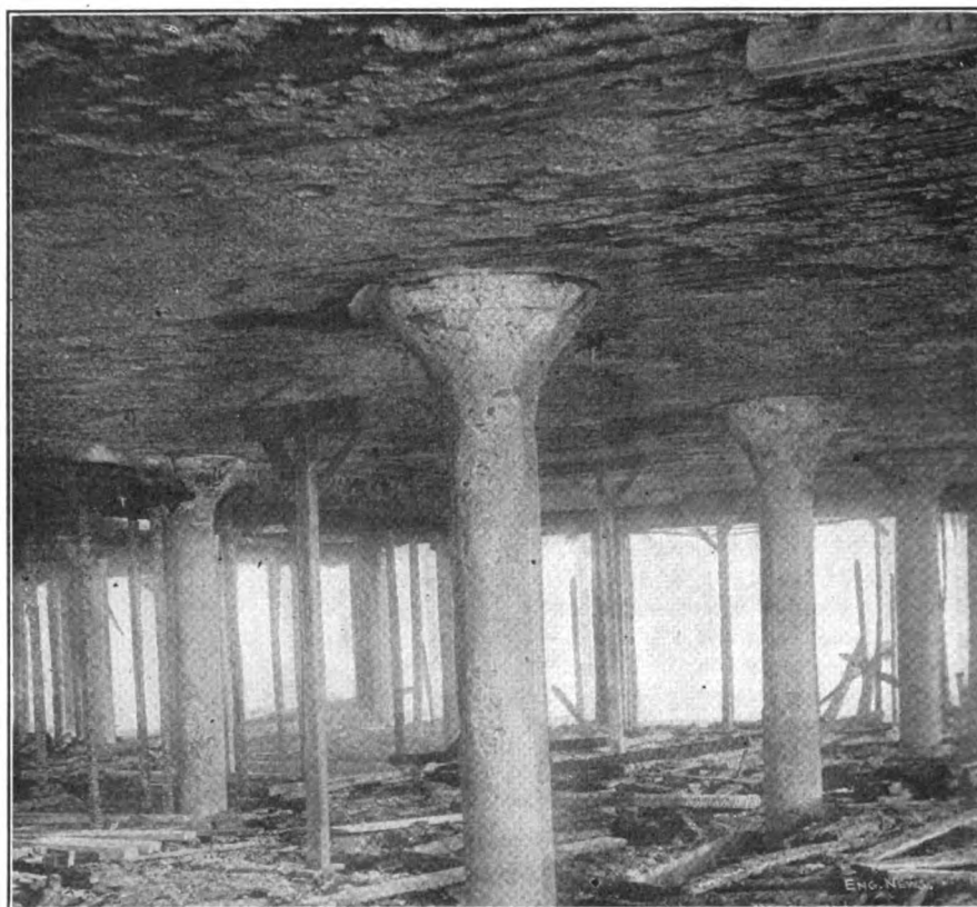
A FLOOR OF A CONCRETE BUILDING AFTER A FIRE WHICH BURNED OUT ALL OF THE FALSEWORK
