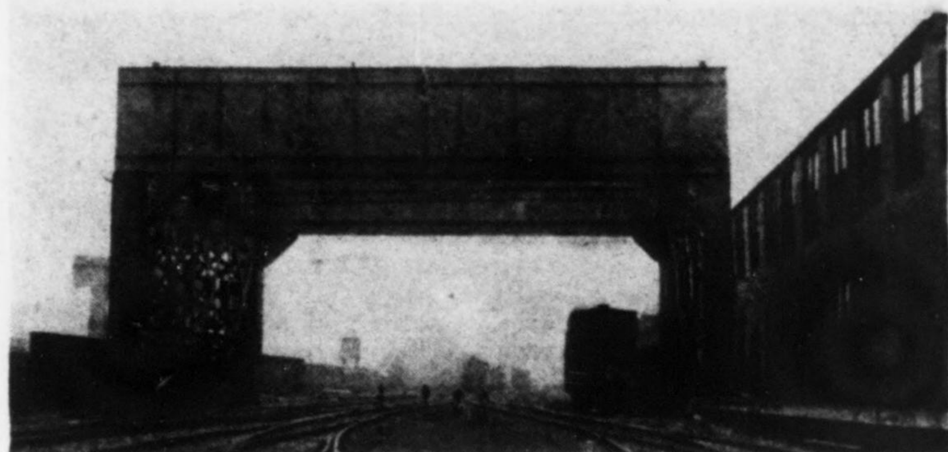
FIG. 6—SPECIAL VIADUCT CONSTRUCTION Above—Bent at left has farther column braced longitudinally and bent at right is braced laterally; the next bent is skewed and two A-frames carry the cross-girder. Below—Two bents form square tower, across which the track stringers run diagonally.
