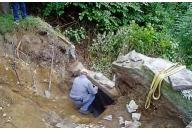
prevent washout were added to the backfill as it was put back and compacted behind the retaining wall after the realignment work of the stones was finished.
