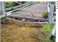
At he same time, settled threshold stones across the east side of the bridge entrance were re-leveled, even with the wooden planks of the roadbed of the bridge.
