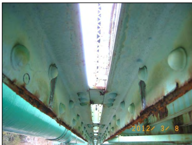
Photo 32: Span 1 Left Truss - L6L7 at tie plate #3, underside: Section loss <12-0184>
