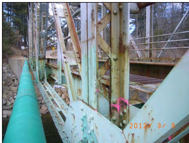
Photo 35: Span 2 Left Truss - U4L4 at L4: Section loss <12-0333>
