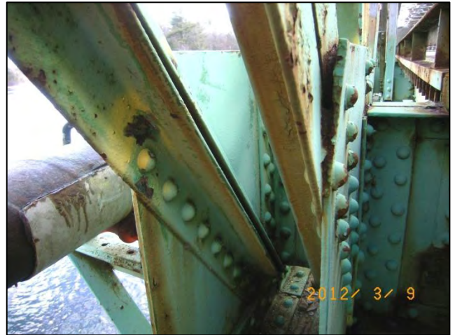
Photo 50: Span 2 Right Truss - L6U7 at L6: Section loss. <12-0445>
