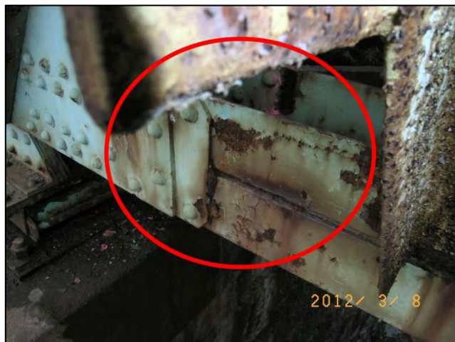
Photo 21: Span 1 Right Truss - L0L1 at L0, from Right: Section loss <12-0202a>
