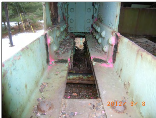
Photo 22: Span 1 Right Truss - L0L1 at L0, looking into L0: Section loss <12-0203>
