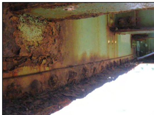
Figure 13: Floorbeam deterioration (from 2011 NHDOT (Draft) Inspection Report, Image No, D077-62)
