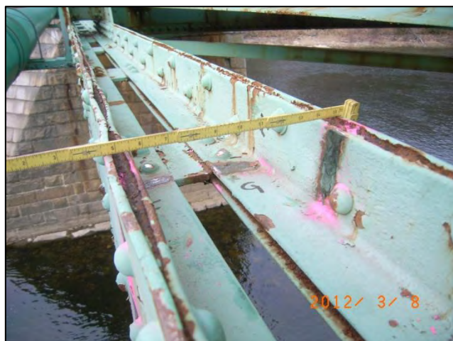
Photo 31: Span 1 Left Truss - L6L7 at tie plate #3 (mid-panel): Section loss <12-0182>
