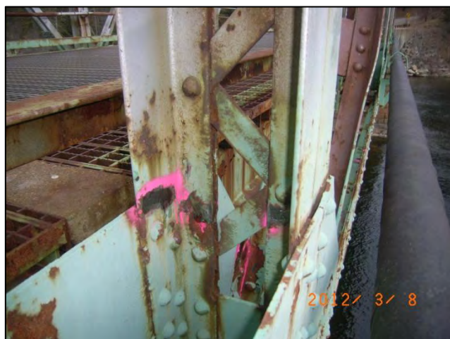
Photo 33: Span 1 Right Truss - U3L3 at L3: Section loss <12-0227>
