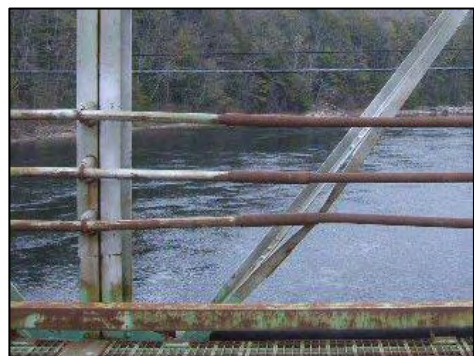
Figure 8: Truss member impact damage
