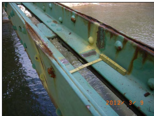
Photo 26: Span 2 Right Truss - L3L4 between tie plates #2 & #3: Section loss <12-0413>
