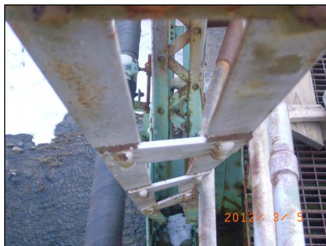
Photo 16: Span 1 Right Truss – L3U4: Impact damage in lower half, looking toward L3 <12-0048>
