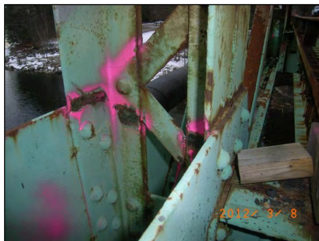
Photo 38: Span 1 Right Truss – U6L6 at L6: Section loss <12-0267>
