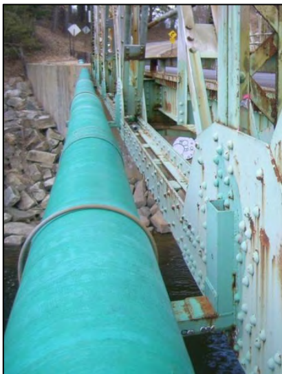
Figure 11: Utility brackets welded to gusset plates (Left side shown, Right side similar)
