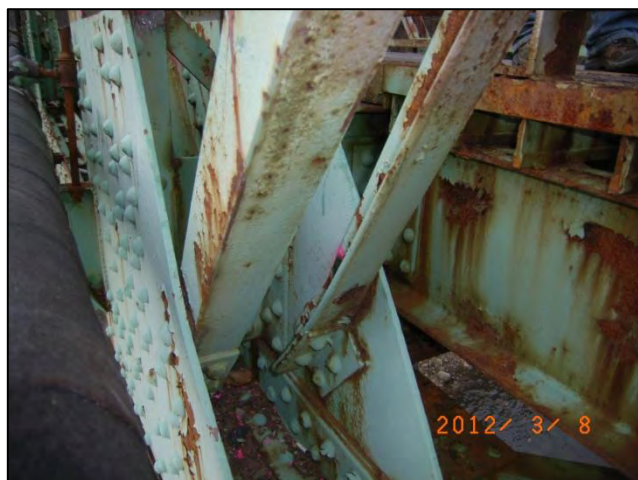
Photo 43: Span 1 Right Truss - L3U4 at L3: Section loss <12-0230>
