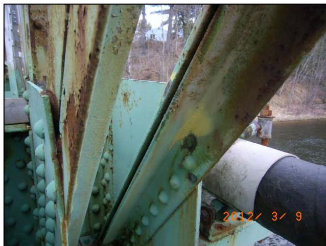
Photo 41: Span 2 Right Truss - U2L3 at L3: Section loss <12-0406>
