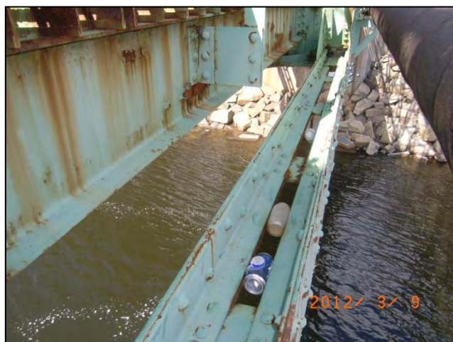
Photo 27: Span 2 Right Truss - L4L5 looking toward panel point L5: Section loss <12-0423>
