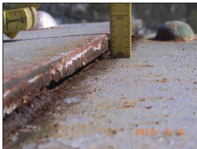
Photo 4: Span 2 Right Truss at U7: Pack rust at top chord and bracing gusset plate. <12-0105>
