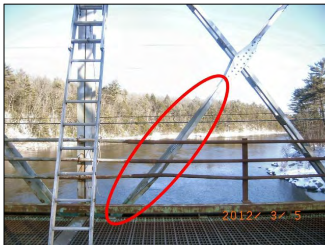
Photo 17: Span 1 Right Truss – U4L5: Impact damage <12-0053a>
