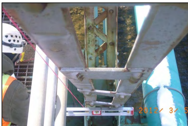
Figure 5: Documentation of impact damage
