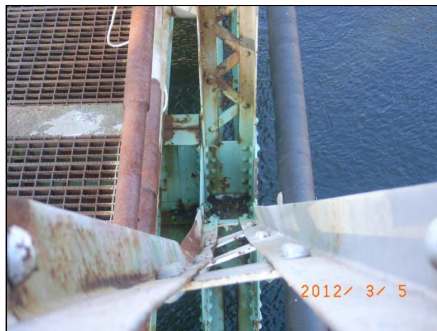
Photo 18: Span 1 Right Truss – U4L5: Impact damage, looking toward L5 <12-0055>
