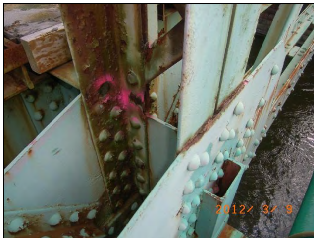
Photo 36: Span 2 Left Truss - U4L4 at L4: Section loss <12-0334>
