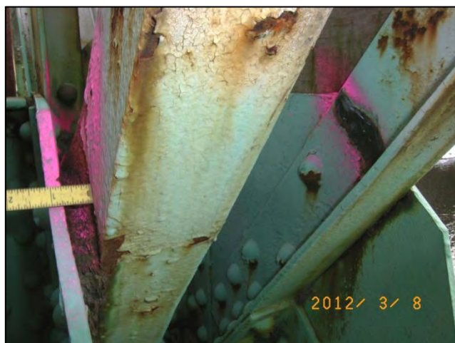
Photo 45: Span 1 Left Truss - L5U6 at L5: Section loss <12-0166>
