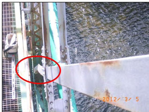
Photo 14: Span 1 Left Truss – L5U6: Impact damage looking back from U6 <12-0032a>
