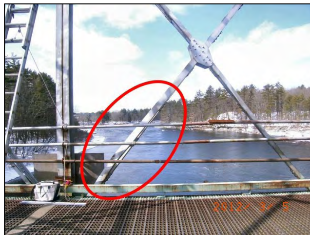
Photo 12: Span 1 Left Truss - L5U6: Impact damage <12-0030>
