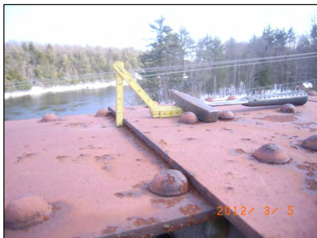
Photo 1: Span 1 Right Truss at U1: Pack rust at top chord and bracing gusset plate <12-0042>
