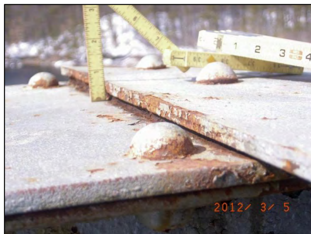
Photo 2: Span 1 Left Truss at U6: Pack rust at top chord and bracing gusset plate <12-0033>
