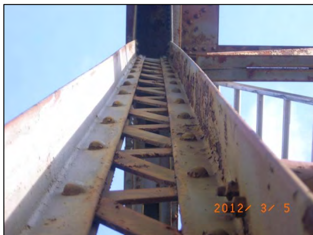
Photo 7: Span 1 Left Truss at U2L2 (Begin side looking up): Impact damage: axial rotation <12-0008>
