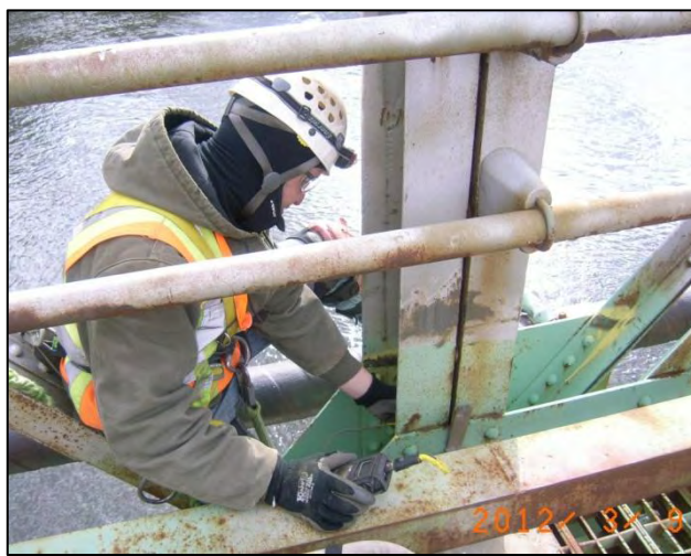
Figure 6: Measuring section loss on a truss vertical
