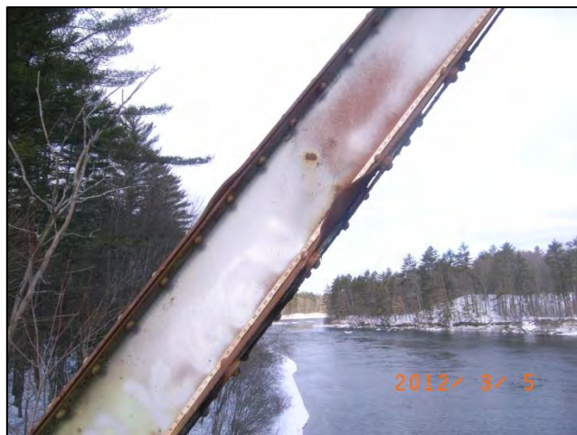
Photo 5: Span 1 Left Truss at L0U1: Localized impact damage <12-0003>
