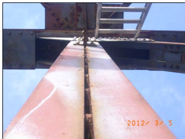
Photo 8: Span 1 Left Truss at U2L2 (Right side looking up): Impact damage: axial rotation <12-0009>
