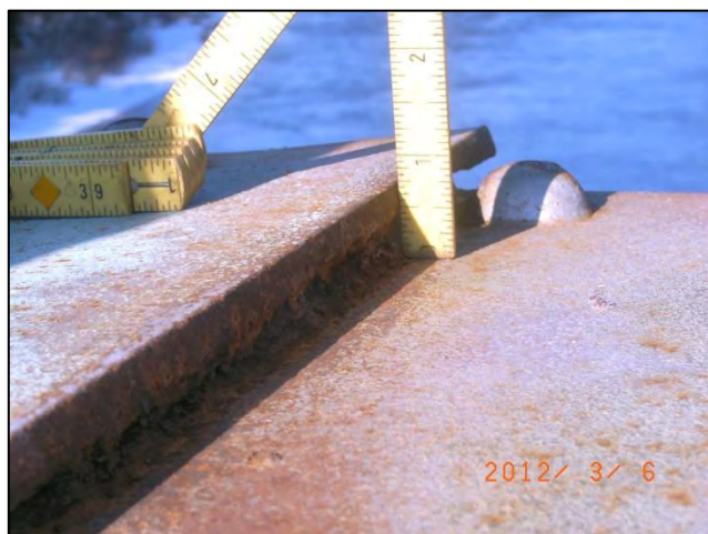
Photo 3: Span 2 Left Truss at U1: Pack rust at top chord and bracing gusset plate. <12-0066a>
