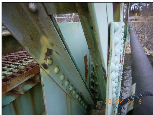
Photo 39: Span 2 Right Truss - U1L2 at L2: Section loss <12-0396>
