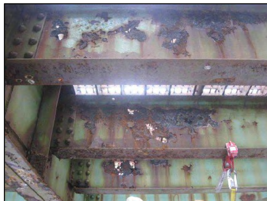
Figure 12: Stringer deterioration (from 2011 NHDOT (Draft) Inspection Report, Image No, D077-28)
