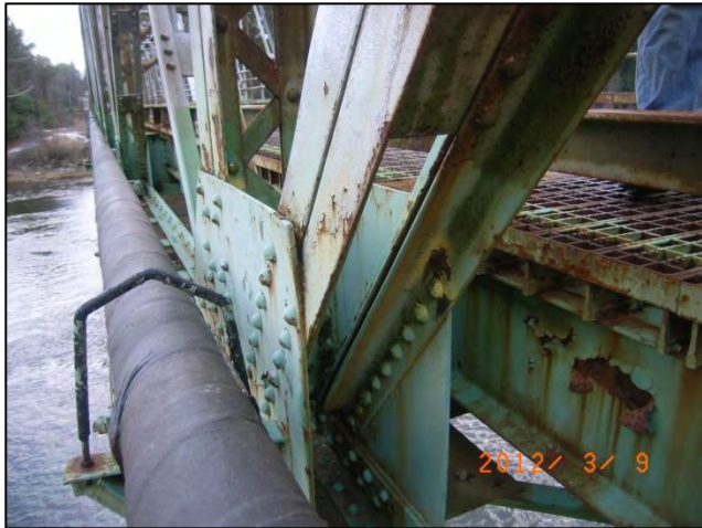
Photo 49: Span 2 Right Truss – L6U7 at L6: Section loss. <12-0443>
