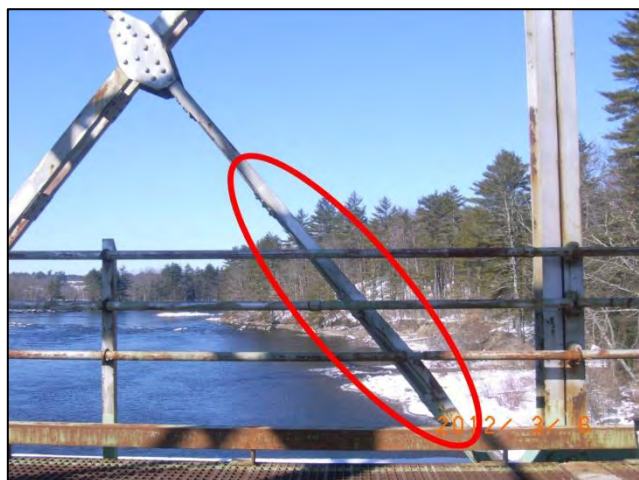
Photo 19: Span 2 Left Truss - U5L6: Impact damage. <12-0071a>
