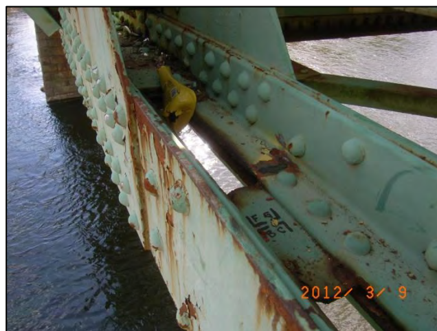
Photo 28: Span 2 Right Truss - L4L5 looking back at panel point L4: Section loss <12-0424>
