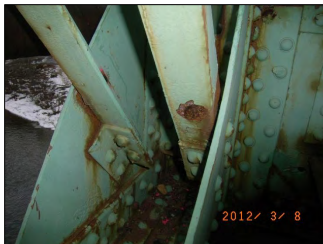
Photo 44: Span 1 Right Truss - L3U4 at L3: Section loss <12-0232>
