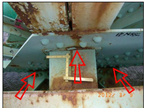
Figure 10: Typical pitting lines, from top
