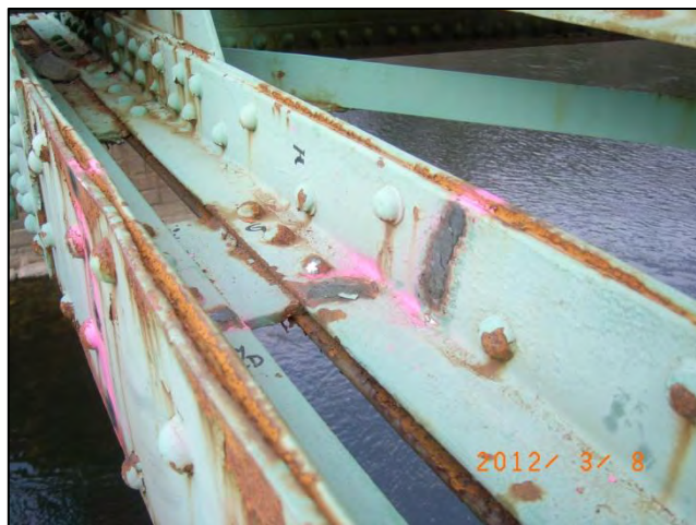
Photo 29: Span 1 Left Truss - L5L6 at tie plate #5 (near L6): Section loss <12-0169>
