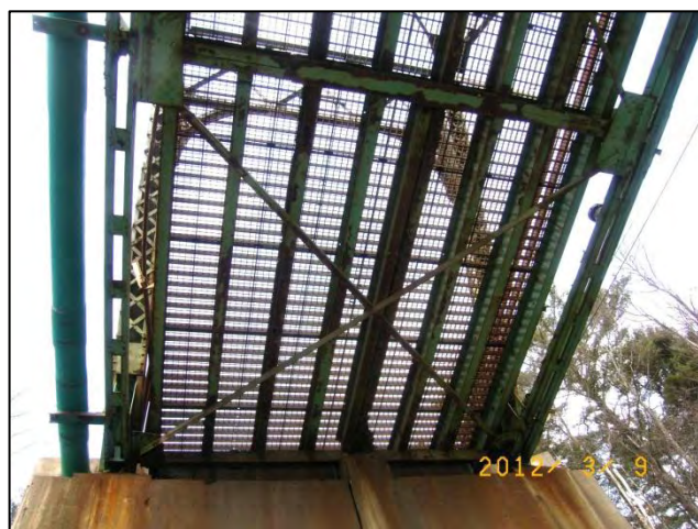
Figure 4: Typical floor framing - Span 2 Panel 9
