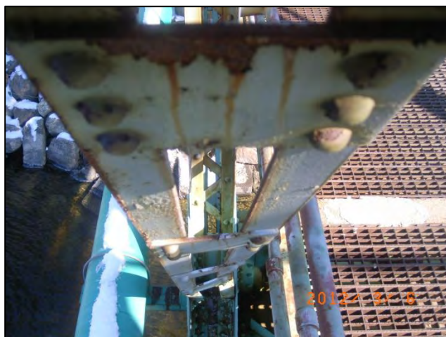
Photo 20: Span 2 Left Truss - U5L6: Impact damage, looking toward L6. <12-0072>
