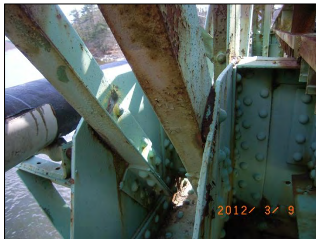
Photo 48: Span 2 Right Truss - L5U6 at L5: Section loss. <12-0432>
