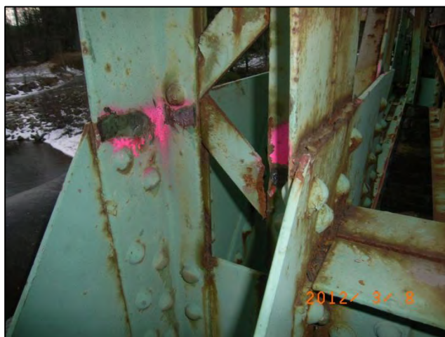
Photo 34: Span 1 Right Truss - U3L3 at L3: Section loss <12-0229>
