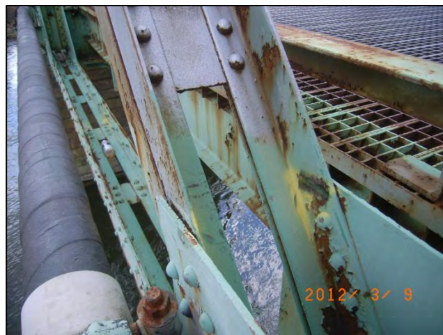
Photo 42: Span 2 Right Truss - U2L3 at L3: Section loss <12-0407>
