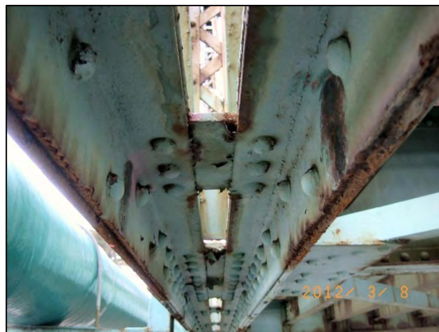
Photo 30: Span 1 Left Truss - L5L6 at tie plate #5, underside: Section loss <12-0172a>
