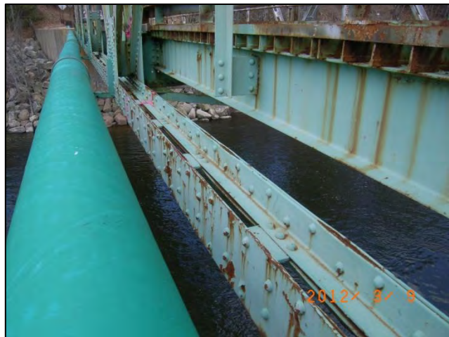
Photo 23: Span 2 Left Truss - L2L3 looking from L2: Section loss <12-0314>
