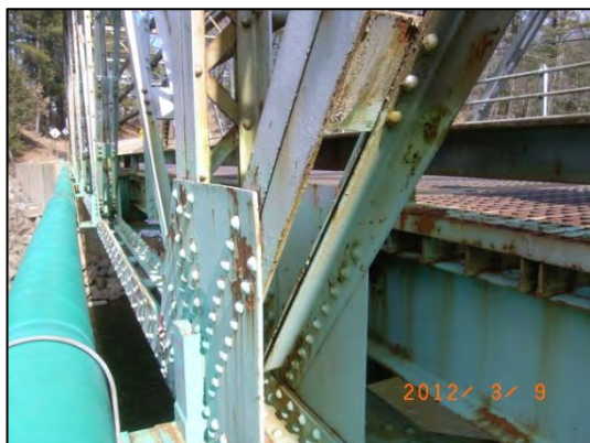
Figure 9: Typical lower chord gusset plate conditions (Span 2 Left Truss at L3).
