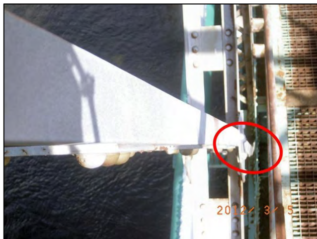
Photo 11: Span 1 Left Truss at U5L6: Impact damage in lower half, looking from U5 <12-0024a>
