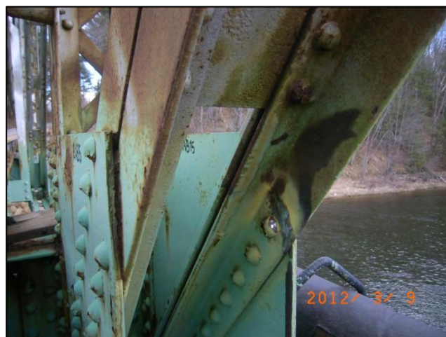
Photo 40: Span 2 Right Truss - U1L2 at L2: Section loss <12-0397>
