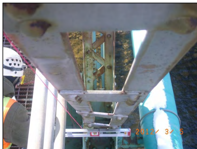
Photo 10: Span 1 Left Truss - L1U2: Impact damage. <12-0019>
