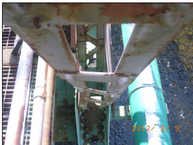
Photo 13: Span 1 Left Truss – L5U6: Impact damage in lower half of member <12-0031>
