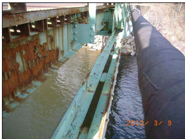
Photo 25: Span 2 Right Truss - L3L4 looking toward panel point L4: Section loss <12-0413>
