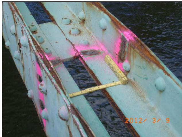
Photo 24: Span 2 Left Truss - L2L3 at 5 th tie plate: Section loss <12-0315>
