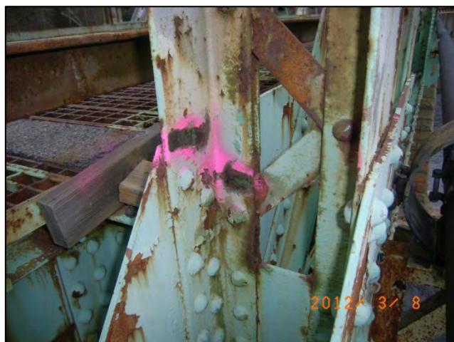
Photo 37: Span 1 Right Truss – U6L6 at L6: Section loss <12-0264>
