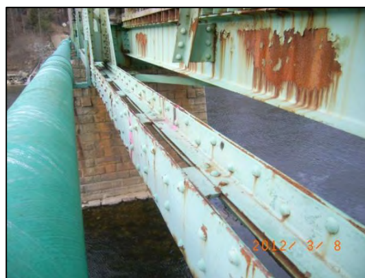
Figure 10: Typical truss bottom chord
