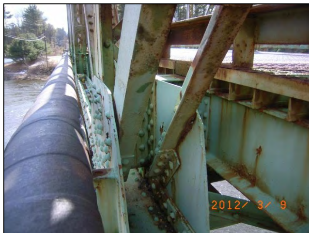
Photo 47: Span 2 Right Truss - L5U6 at L5: Section loss. <12-0431>
