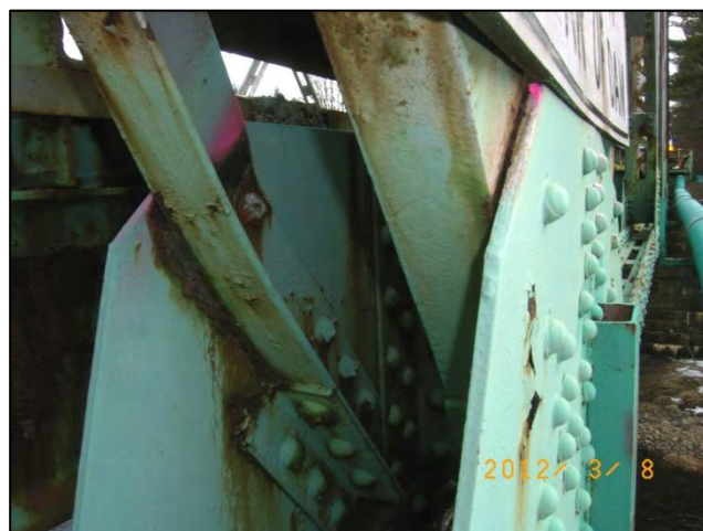
Photo 46: Span 1 Left Truss - L5U6 at L5: Section loss <12-0167>
