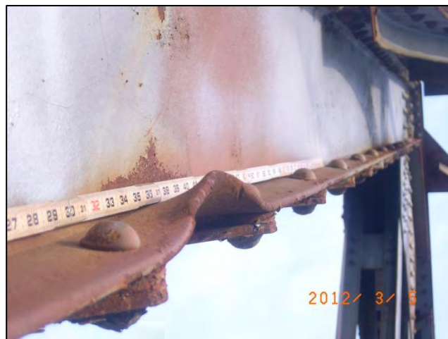
Photo 6: Span 1 Left Truss at L0U1: Localized impact damage <12-0004>
