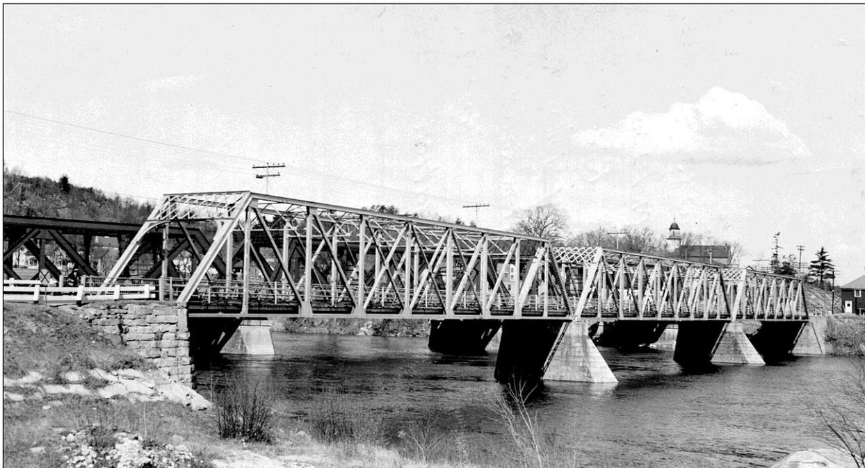
FIGURE 20: Hooksett Village Bridge, shown April 13, 1942. The American Bridge Company built an exact duplicate replacement span to replace the one destroyed in the flood (at left) using the original shop drawings they had retained in their files (NHHD Bridge Inventory Card). Demolished and replaced with pedestrian bridge, 2017.
