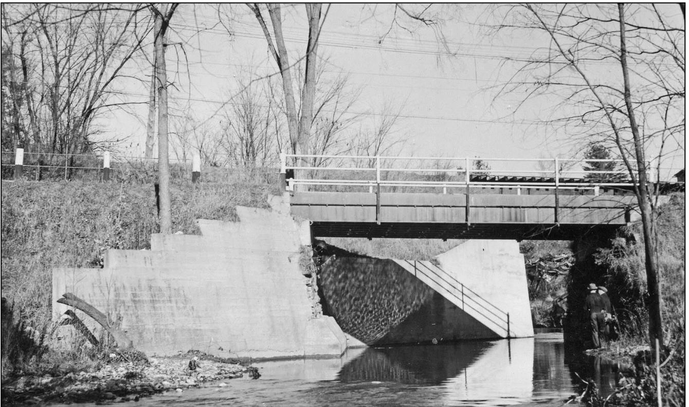
FIGURE 14: Claremont 106/120, NH 12/103 over Red River Brook. Designed by John Storrs and built by C. E. Walbridge, Plymouth NH in 1908. Replaced in 1997. This was a 30' span I-beam stringer bridge with a reinforced concrete slab deck. Photo November 19, 1940 (NHHD Bridge Inventory Card).
