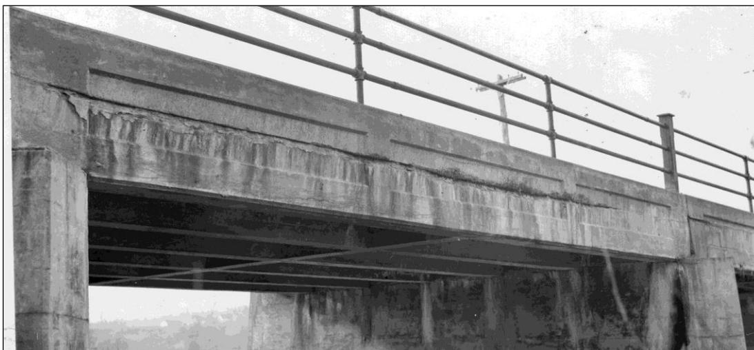
FIGURE 62: Elm Street Bridge, Newport (1916). Underside, showing concrete encased I-beams. Bridge replaced in 1985. Photo November 19, 1940 (NHHD Bridge Inventory Card).
