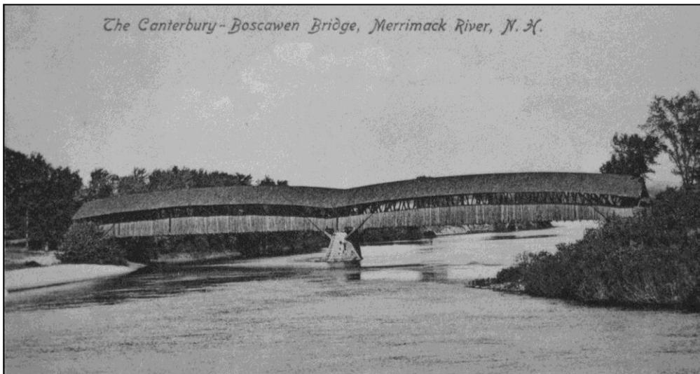
FIGURE 4: Boscawen-Canterbury Covered Bridge over Merrimack River, built in 1857 with unusual arched truss "humpback" design thought at the time to be only one of its type in the US. Storrs inspected the bridge in October 1906 and recommended its replacement with a steel truss bridge. He was paid \$30 for his inspection and report, \$15 by each town. Postcard photo before 1907 (Canterbury Historical Society).
