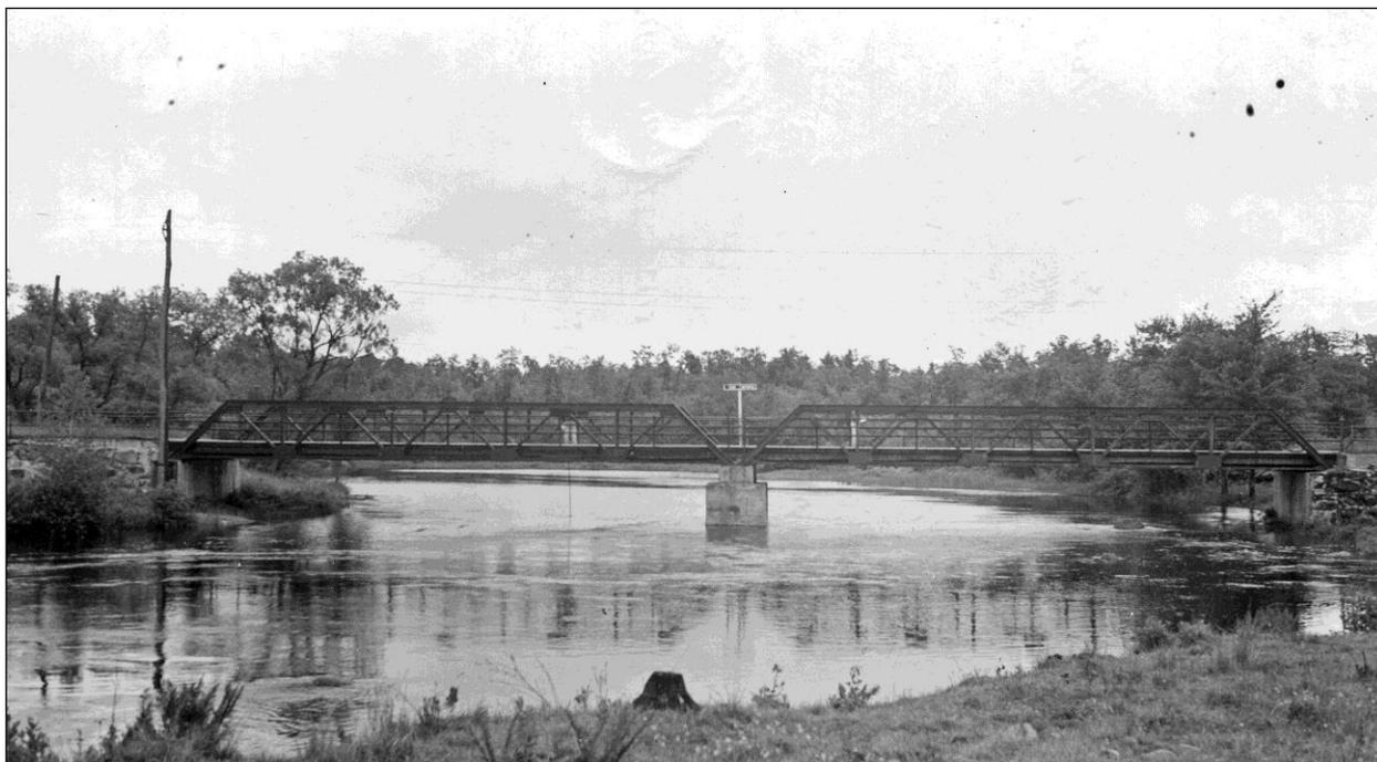
FIGURE 23: Tilton-Northfield 128/158 (now 109/062), a two span Warren pony truss carrying NH 140 over Winnepesaukee River. Designed by John Storrs and built by Canton Bridge Co. in 1910. Replaced in 1968. Each truss measured 67'-7" between bearings. Photo June 17, 1942 (NHHD Bridge Inventory Card).
