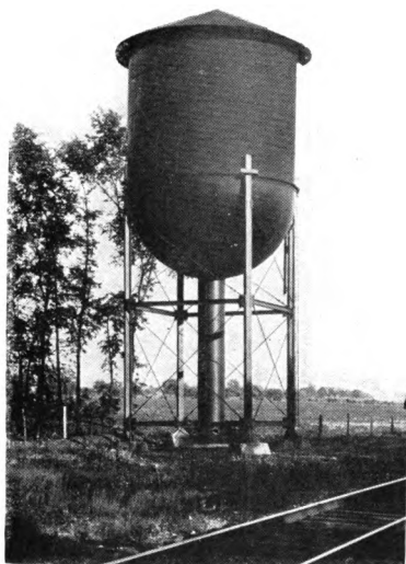
WATER TOWER FOR L. V. R. R. Capacity 100,000 Gals., Height 23 Ft. 6 inches to Bottom of Tank Erected at Reider, N. J., in 1911
