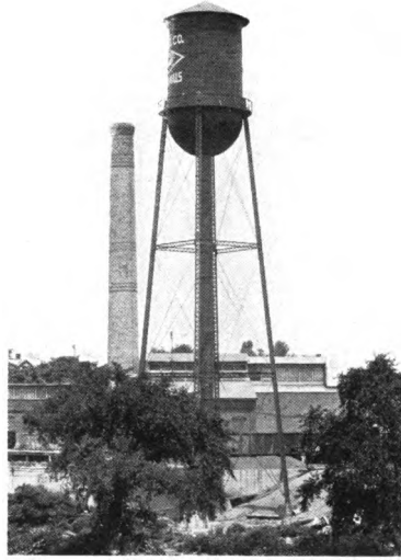
WATER TOWER FOR THE HAEMMERSCHLAG MFG. CO. Capacity 100,000 Gals., Height 100 Ft. to Tank Bottom Erected at Garfield, N. J., in 1911
