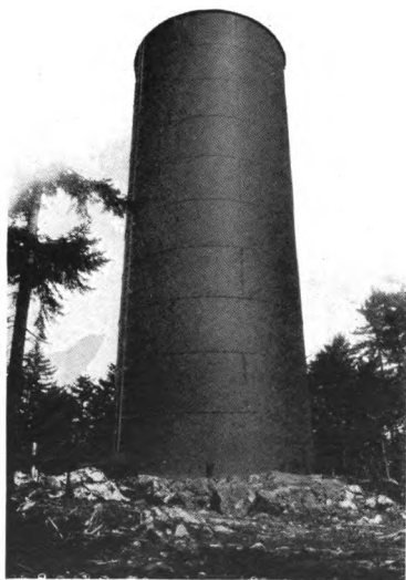
STAND-PIPE FOR TOWN OF NORTH HAVEN Diam. 25 Ft., Height 67 Ft. Capacity 246,000 Gals. Erected at North Haven, Me., in 1911
