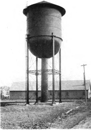
WATER TOWER FOR P. R. R. Capacity 35,000 Gals., Height 22 Ft. to Tank Bottom Erected at Penns Grove, N. J., in 1910
