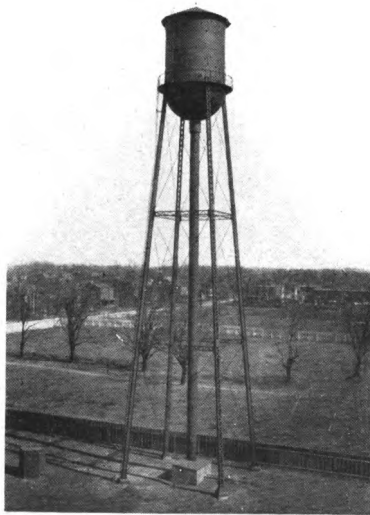
WATER TOWER FOR E. H. FITLER & CO. Capacity 50,000 Gals., Height 100 Ft. to Bottom of Tank Erected at Philadelphia, Pa., in 1914
