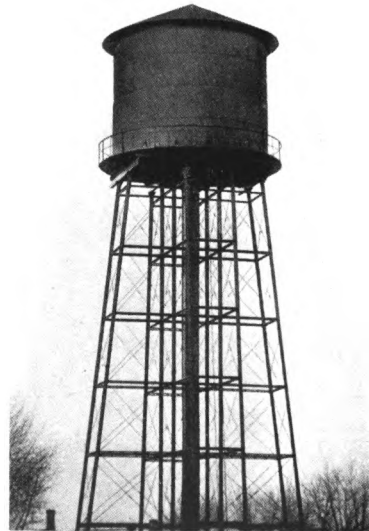
WATER TOWER FOR TOWN OF DENTON Capacity 65,000 Gals., Height 75 Ft. to Bottom of Tank Erected at Denton, Md., in 1911
