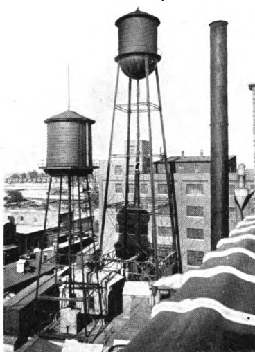
WATER TOWER FOR ARMSTRONG CORK CO. Capacity 60,000 Gals., Height 110 Ft. to Bottom of Tank Erected at Camden, N. J. in 1912
