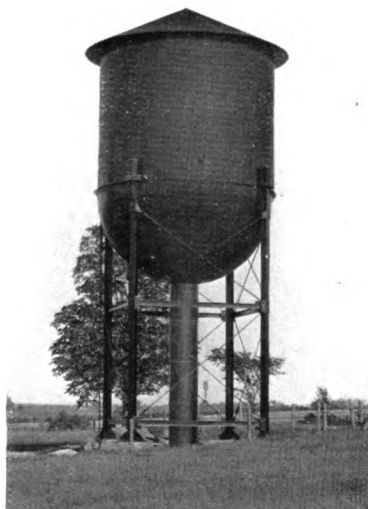
WATER TOWER FOR L. V. R. R. Capacity 100,000 Gals., Height 22 Ft. to Bottom of Tank Erected at West Manchester, N. Y., in 1911
