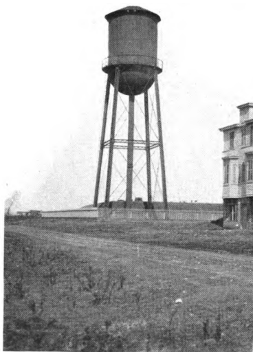
WATER TOWER FOR BOROUGH OF LODI Capacity 50,000 Gals., Height 46 Ft. to Bottom of Tank Erected at Lodi, N. J., in 1910
