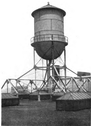
10,000 GAL. GRAVITY TANK & 4-7,500 PRESSURE TANKS Erected for Varick Realty Co., at New York, N. Y.
