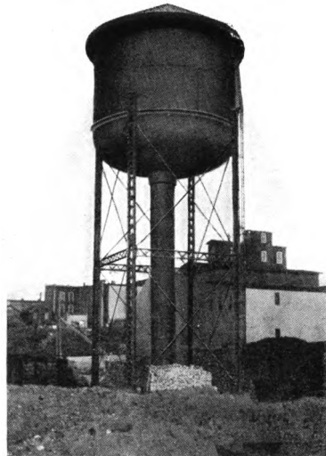
WATER TOWER FOR BORDEN CONDENSED MILK CO. Capacity 40,000 Gals., Height 30 Ft. to Tank Bottom Built 1908
