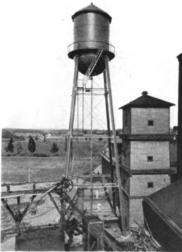
WATER TOWER FOR WATER WORKS AT PLEASANT PLAINS, STATEN ISLAND, N. Y. Capacity 40,000 Gals., Height 75 Ft. to Bottom of Tank Erected in 1900
