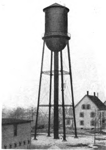
WATER TOWER FOR LOWELL FERTILIZER CO. Capacity 75,000 Gals., Height 75 Ft. to Bottom of Tank Erected at Lowell, Mass., in 1909
