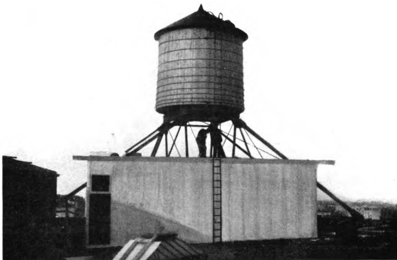
10,000 GAL. GRAVITY TANK AND 7500 GAL. PRESSURE TANK Erected for Earnest Gabler and Bros., in New York, N. Y.
