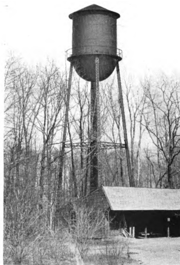
WATER TOWER FOR NASSAU COUNTRY CLUB Capacity 45,000 Gals., Height 60 Ft. to Bottom of Tank Erected at Glen Cove, L. I., in 1911
