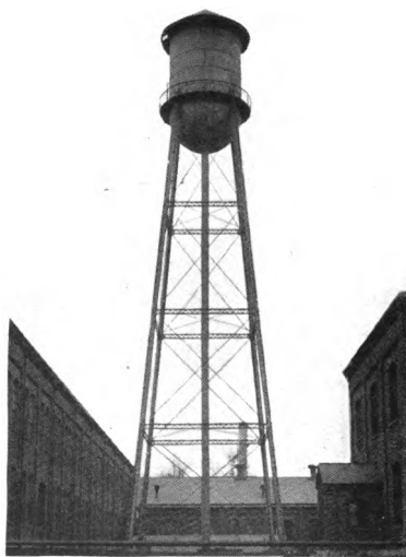
WATER TOWER FOR U. S. ARSENAL Capacity 75,000 Gals., Height 120 Ft. to Bottom of Tank Erected at Frankford, Pa., in 1905
