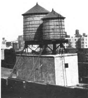
10,000 GAL. GRAVITY TANK 3500 GAL. STAND-PIPE TANK AND 7,500 GAL. PRESSURE TANK Erected for the Folsom Estate Agency in New York, N. Y.
