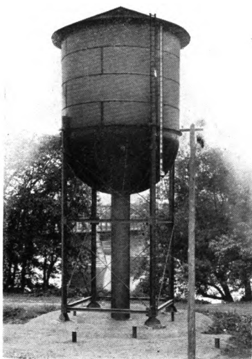
WATER TOWER FOR L. V. R. R. Capacity 100,000 Gals., Height 28 Ft. to Bottom of Tank Erected at Tunkhannock, Pa., in 1910
