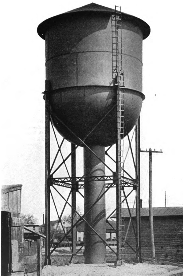
WATER TOWER, FOR P. R. R. Capacity 35,000 Gals., Height 22 Ft. to Bottom of Tank Erected at Elmer, N. J., in 1911
