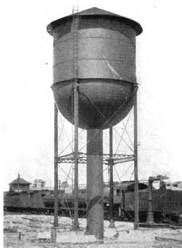
WATER TOWER FOR P. R. R. Capacity 50,000 Gals., Height 24 Ft. to Bottom of Tank Erected at Northumberland, Pa., in 1911
