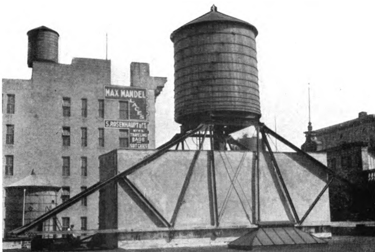
12,000 GAL. GRAVITY TANK AND 9,000 GALLON PRESSURE TANK Erected for Estate of Andrew Alexander, in New York, N. Y.
