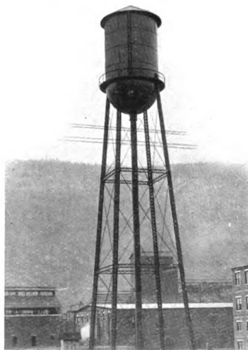
WATER TOWER FOR NEW JERSEY ZINC CO. Capacity 100,000 Gals., Height 100 Ft. to Bottom of Tank Erected at Palmerton, Pa., in 1911
