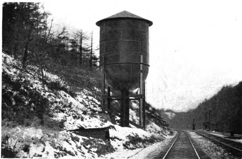
WATER TOWER FOR L. V. R. R. Capacity 70,000 Gals., Height 19 Ft. to Bottom of Tank Erected at Hinkles, Pa., in 1911
