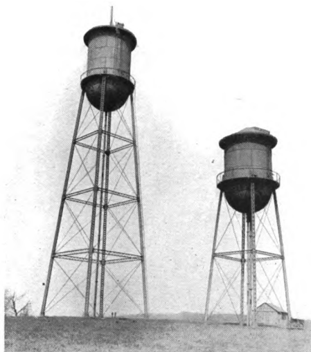
WATER TOWERS FOR THE ATLAS PORTLAND CEMENT CO. Capacity 100,000 Gals., Height 100 Ft. to Bottom of Tank Capacity 40,000 Gals., Height 58 Ft. to Bottom of Tank Erected at Northampton, Pa. in 1907
