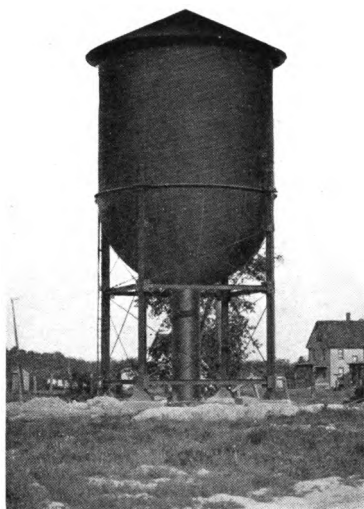
WATER TOWER FOR L. V. R. R. Capacity 100,000 Gals., Height 16 Ft. to Bottom of Tank Erected at East Manchester, N. Y., in 1911
