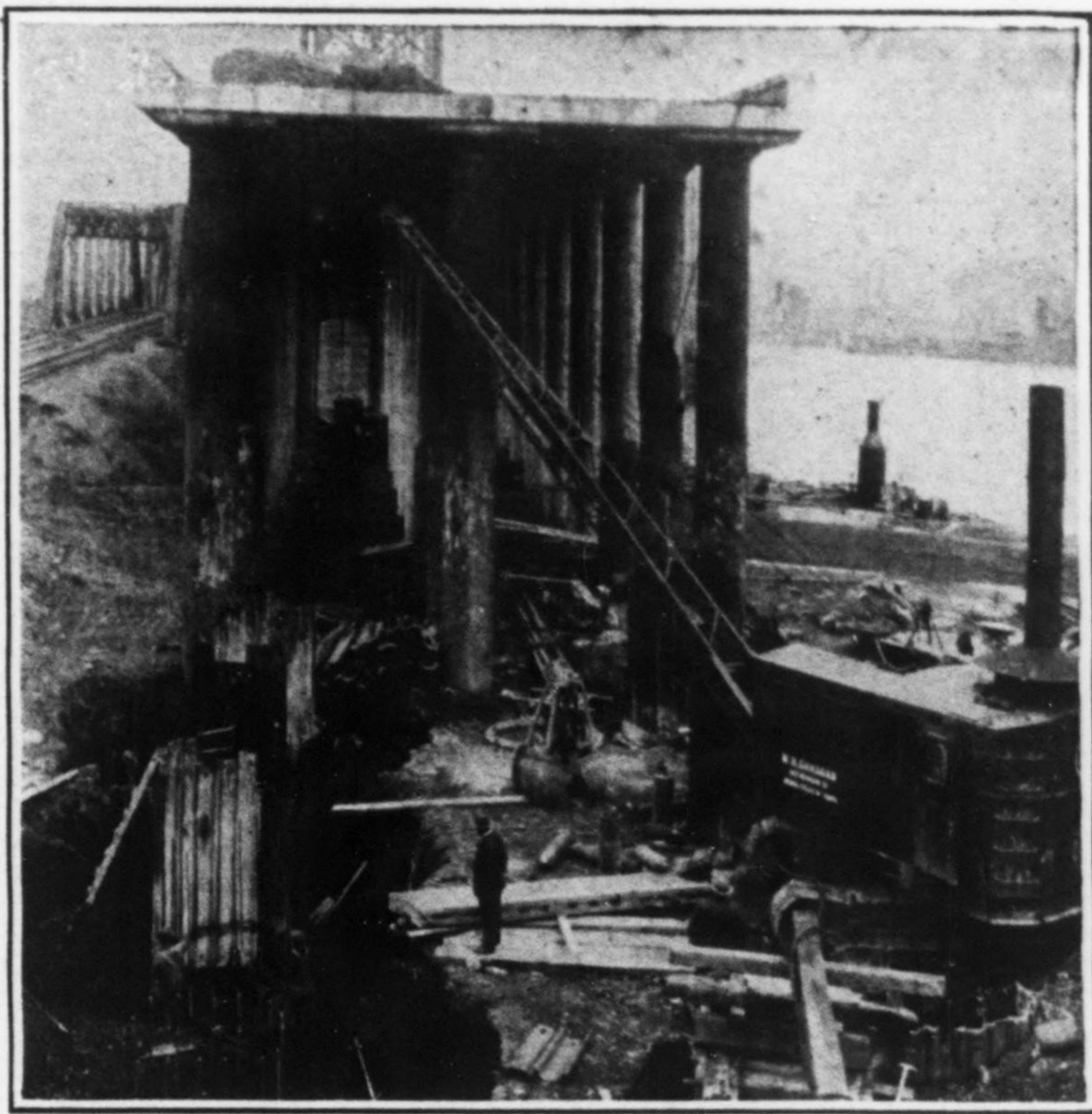
FIG. 3—CIRCULAR PIER CAISSONS AT WEST END OF VIADUCT
