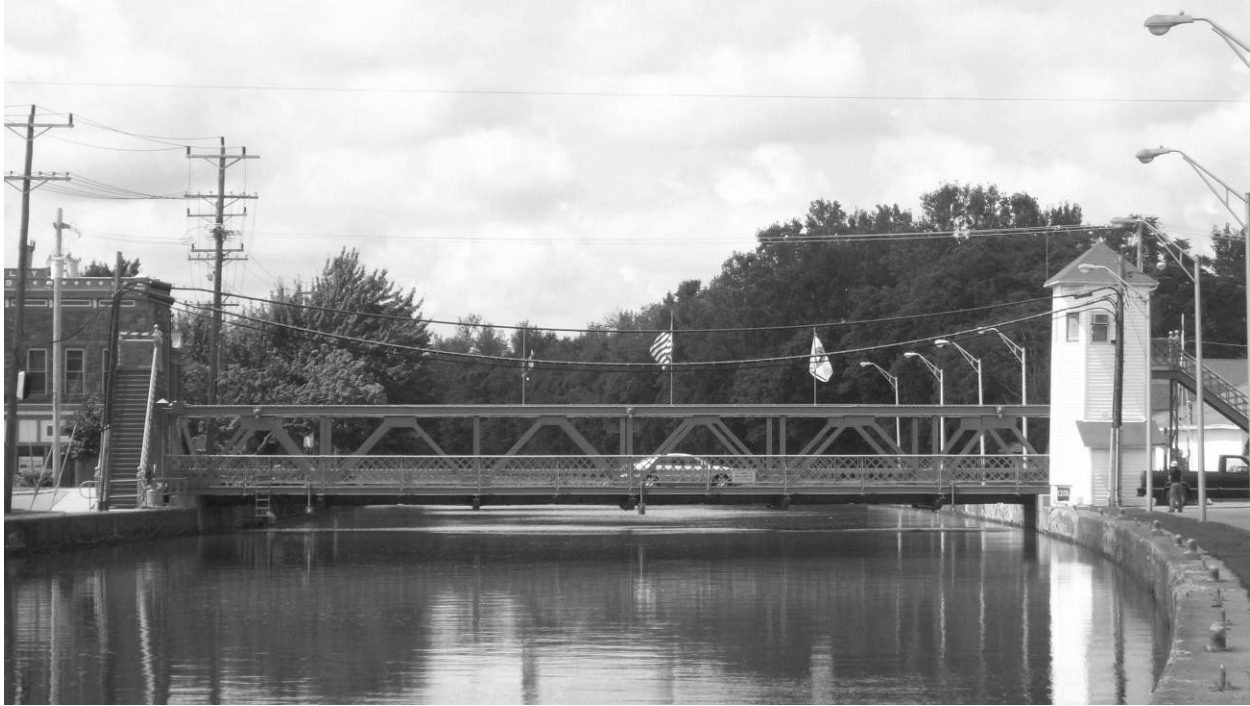
Image 1: Main Street Lift Bridge elevation with control tower at right. Field photograph taken by HAER recording team, summer 2009.
