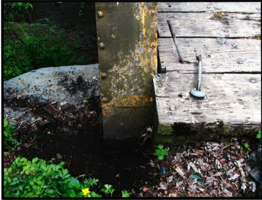
Northwest Bridge Seat
