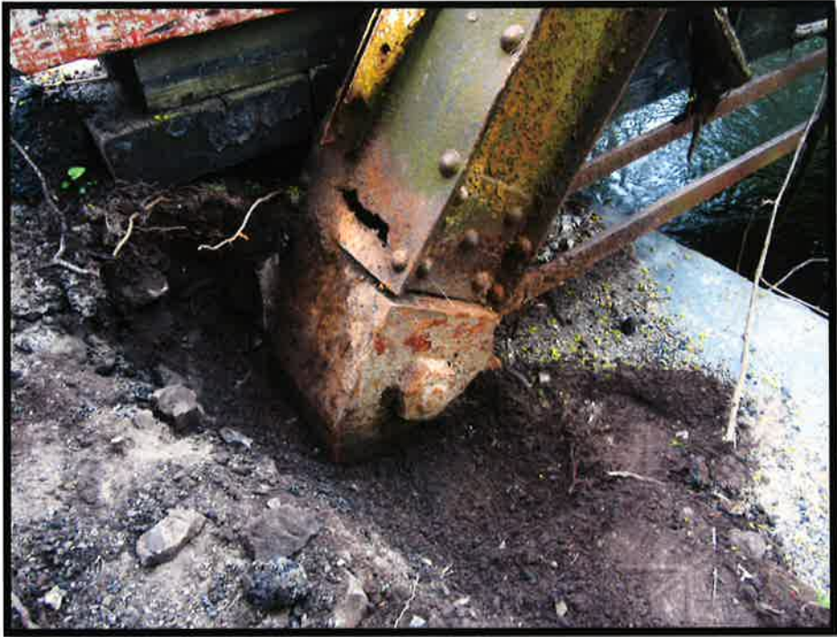
Northeast bridge seat
