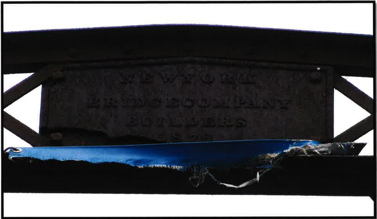
Bridge Plaque East End
