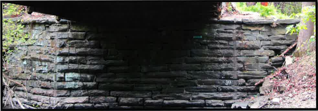
East abutment taken from west abutment
