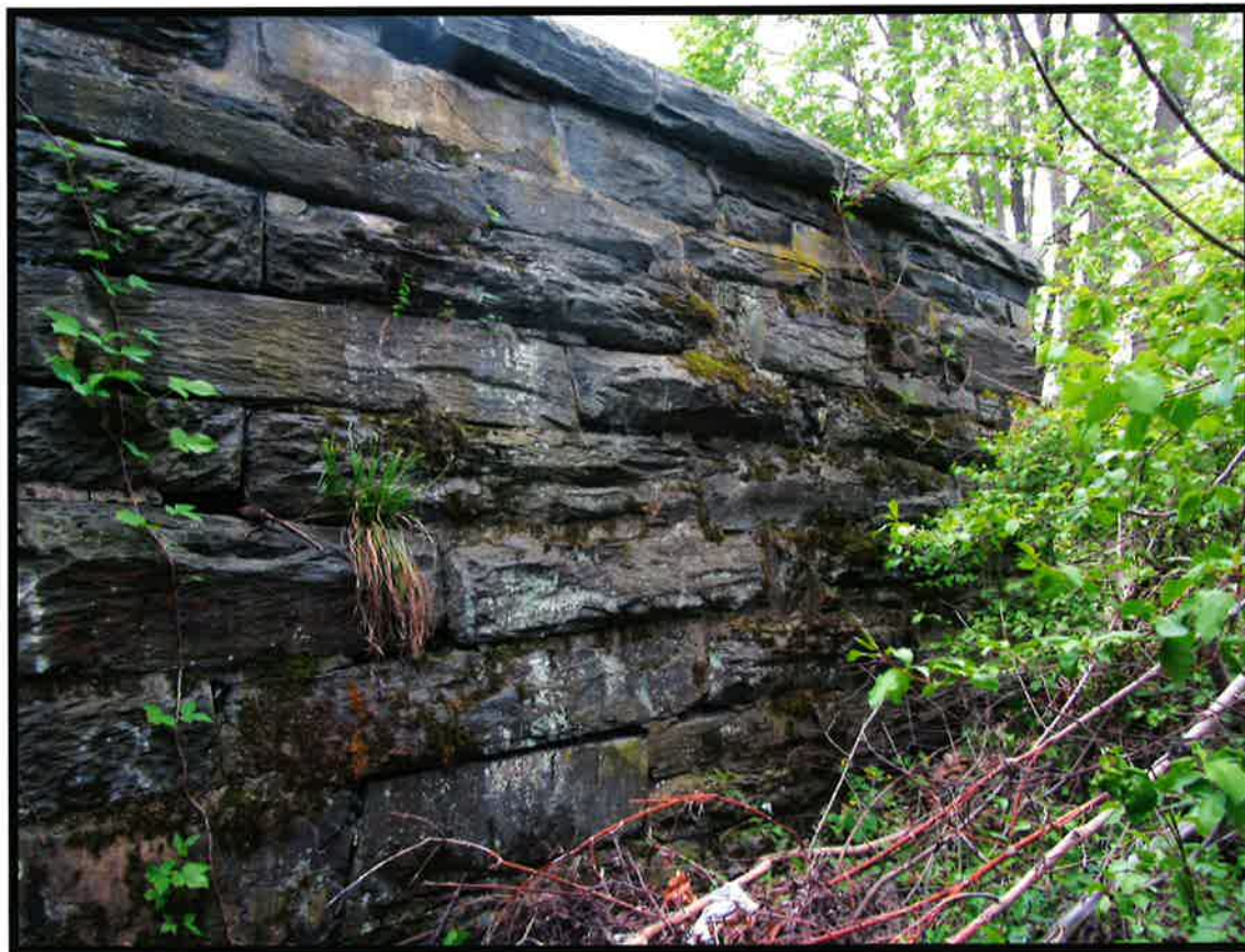
North wing wall of westerly abutment
