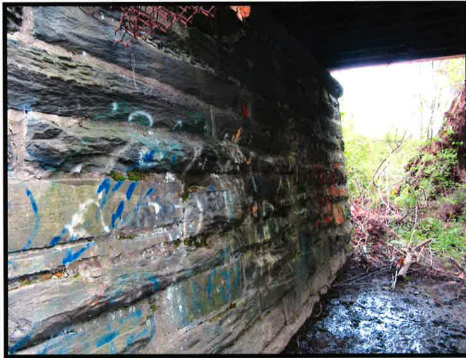
Face of west abutment showing pointed stonework
