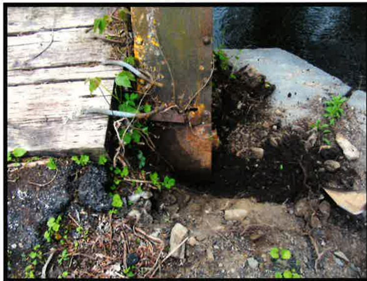
Southwest bridge seat end and side views
