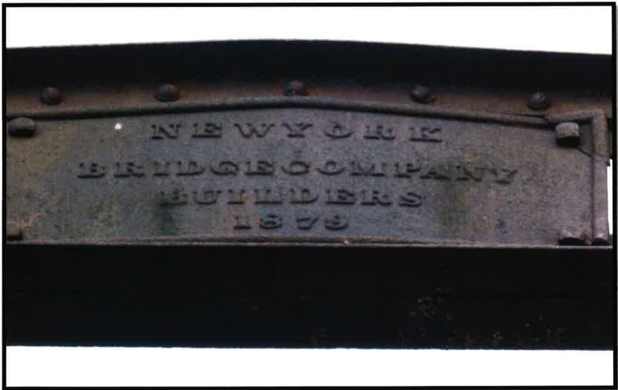
Bridge Plaque West End
