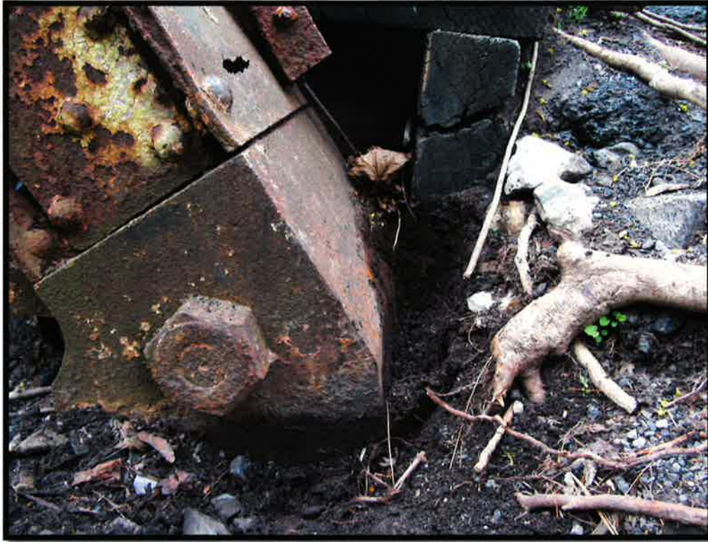
Southeast bridge seat end and side views
