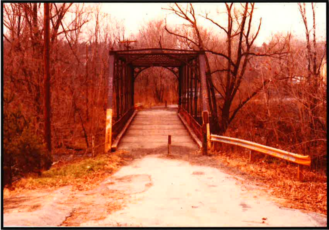
East Portal 1978 NYSDOT
