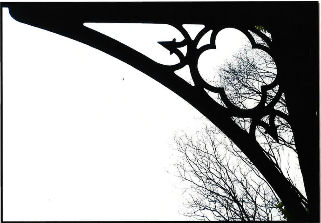
Cast Iron Tracery - Bolted to Cross Truss and Inclined End Post.
