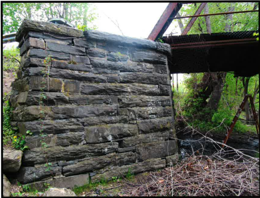
Southerly Wing wall, showing good line of face of abutment
