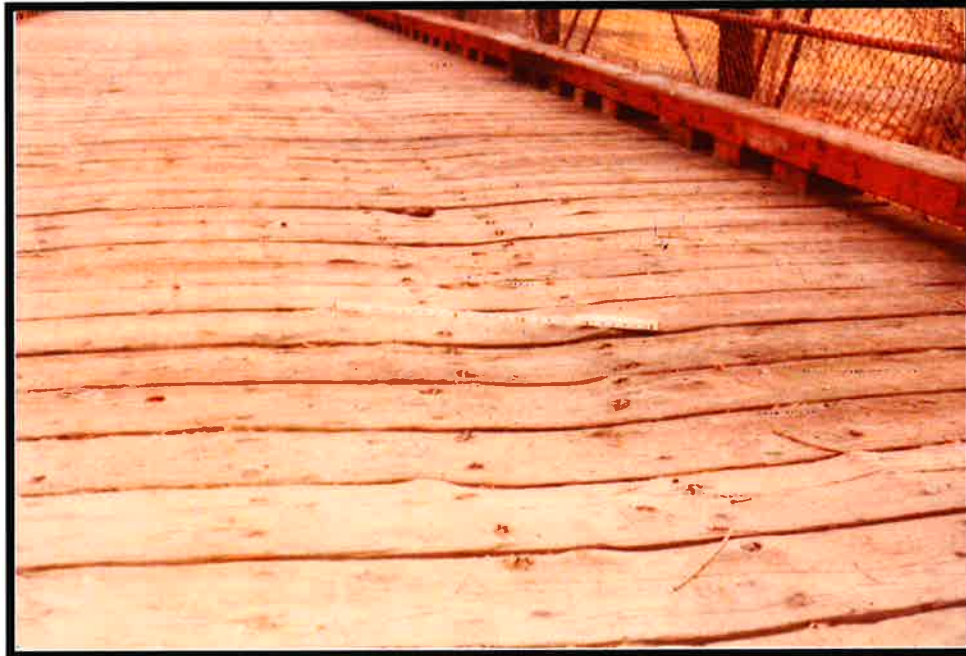
Deck and Curb 1978 NYSDOT
