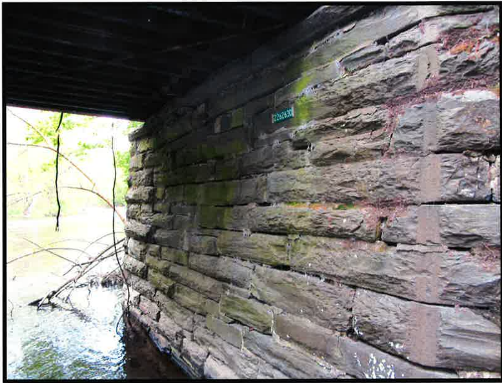
Face of easterly wing wall, excellent condition
