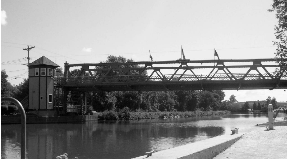
Image 1: Park Avenue Lift Bridge in raised position. Field photograph taken by HAER recording team, summer 2009.
