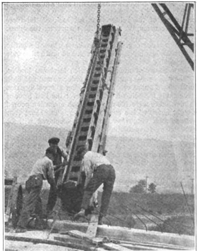
FIG. 7. BALUSTRADE FORM UNITS BEING PLACED
