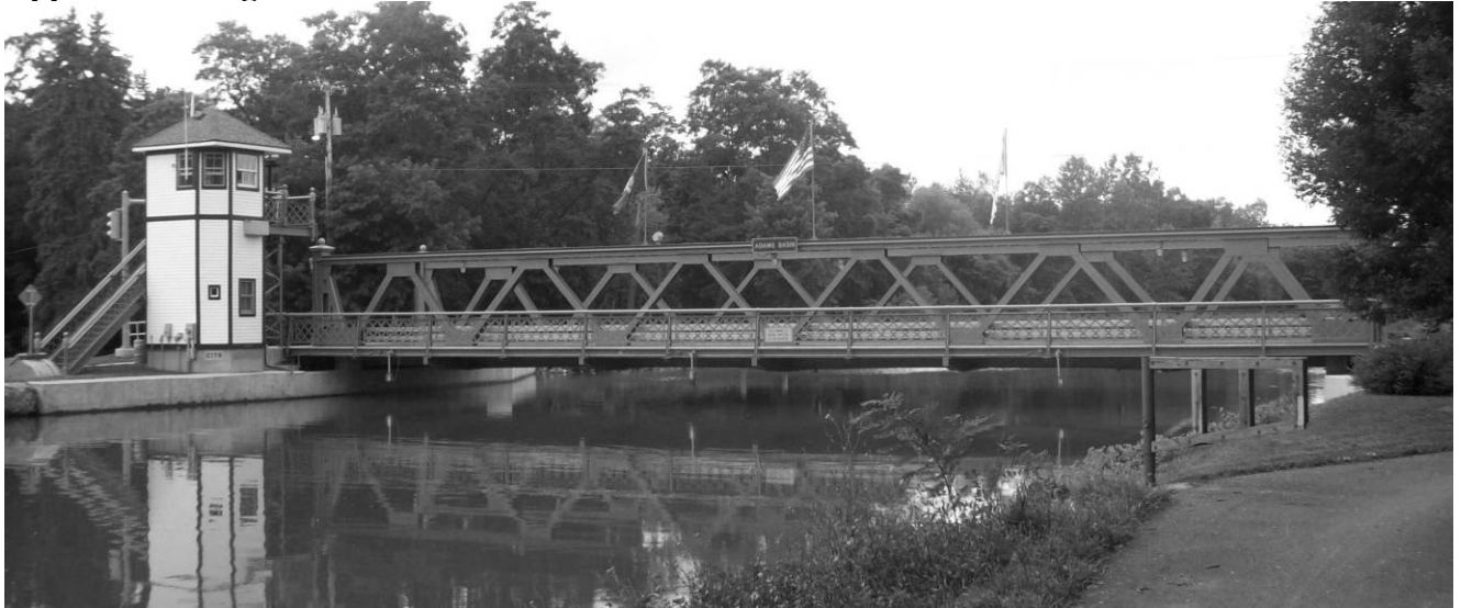
Image 1: Overview of Washington Street Bridge with control tower at left. Field photograph taken by HAER recording team, summer 2009.
