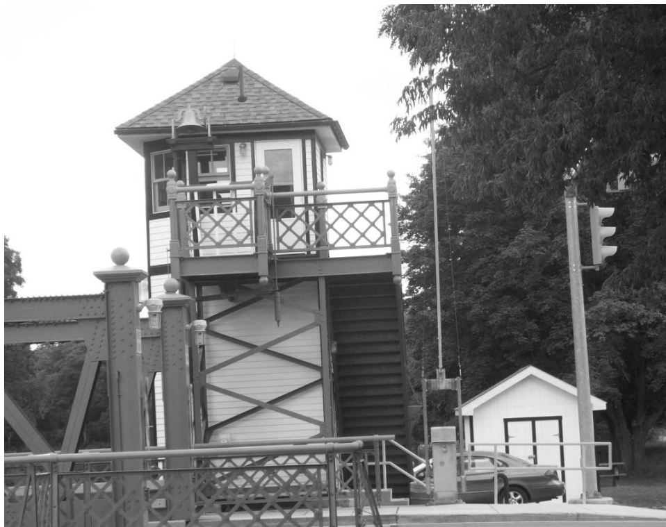
Image 2: Control tower with historic bell and storage shed at rear. Field photograph taken by HAER recording team, summer 2009.
