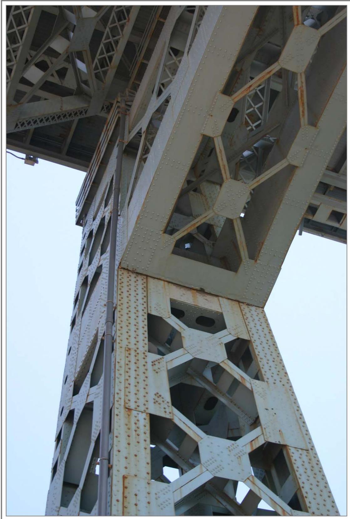
Photo V-20. Detail of truss connection beneath Kosciuszko Bridge
