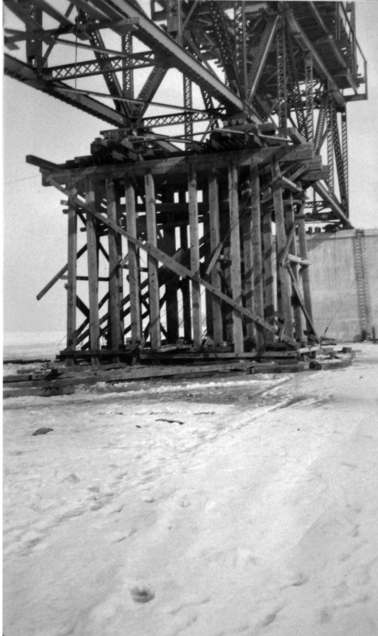
Figure 26. "Close-up view of ice for temporary bent of 12-inch x 12-inch square timbers, Span 5," February 18, 1929. Image shows the use of ice to support falsework for some of the truss spans. Image courtesy Penfield Homestead Museum.
