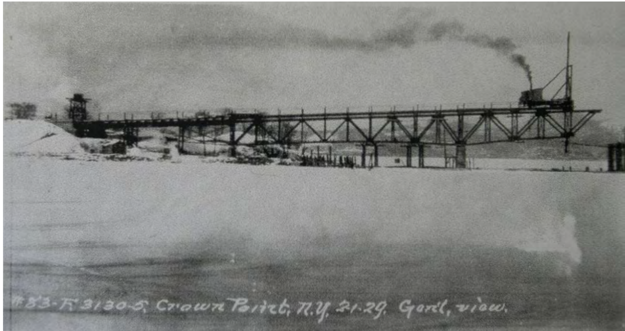
Figure 23. February 2, 1929. "Gen'l View." (LCBC Photo #83, F3130-5, Crown Point, N.Y). View of Spans 1-4 and Span 5 under construction. Image courtesy Moriah Historical Society.
