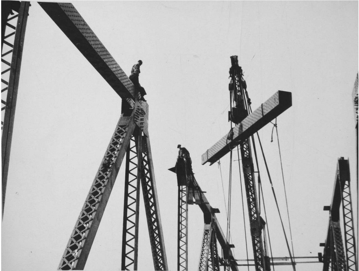
Figure 37. Workers waiting for a section of the top chord to be lifted into place on Span 7, mid-June, 1929. Image courtesy Vermont State Archives.
