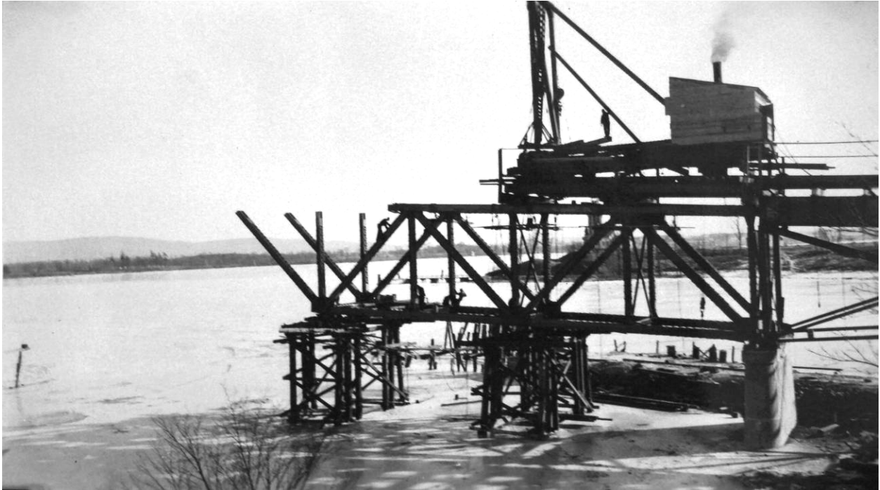
Figure 21. "Second bent falsework and second panel nearly in place" January 15, 1929. View of Span 4 from Fort St. Frederic. Image courtesy Penfield Homestead Museum.
