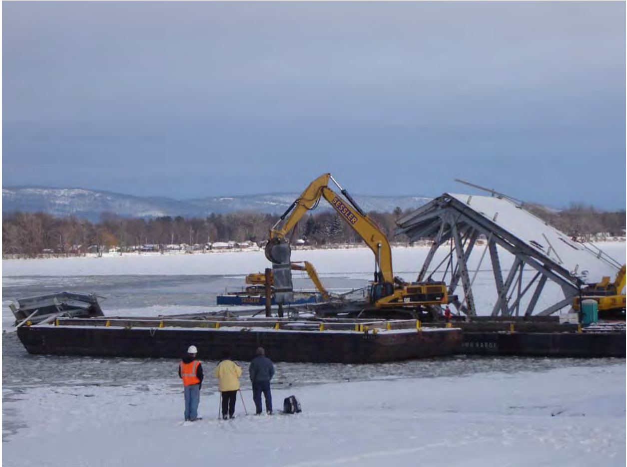
Figure 76. View of backhoe piling salvaged bridge members onto a barge on the New York end of the bridge. The barge will be unloaded at a scrap yard in Port Henry. Photograph by New York State Department of Transportation.
