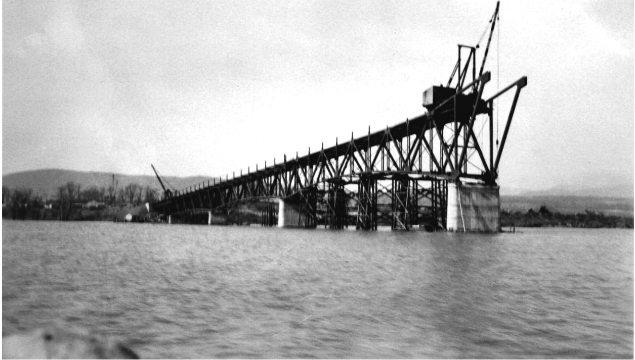
Figure 30. "Bridge from water looking westerly," April 9, 1929. View shows a completed Span 6 and early work on Span 7. Image courtesy Penfield Homestead Museum.
