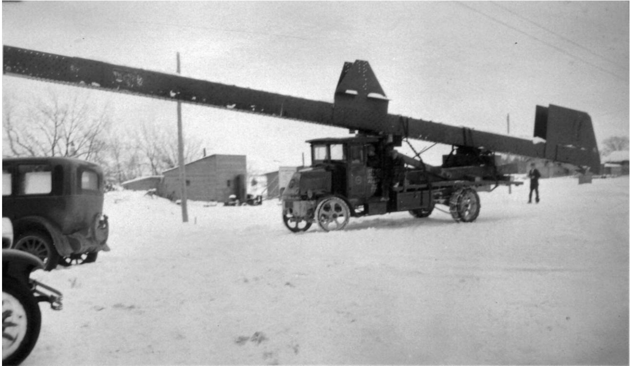
Figure 25. "Trucking L8-10, Weight 14-tons 1780 lbs, this with the timber carriage estimated at approximately 1-ton makes a 16-ton load on a 5-ton Mack truck," February 12, 1929. Image courtesy Penfield Homestead Museum.
