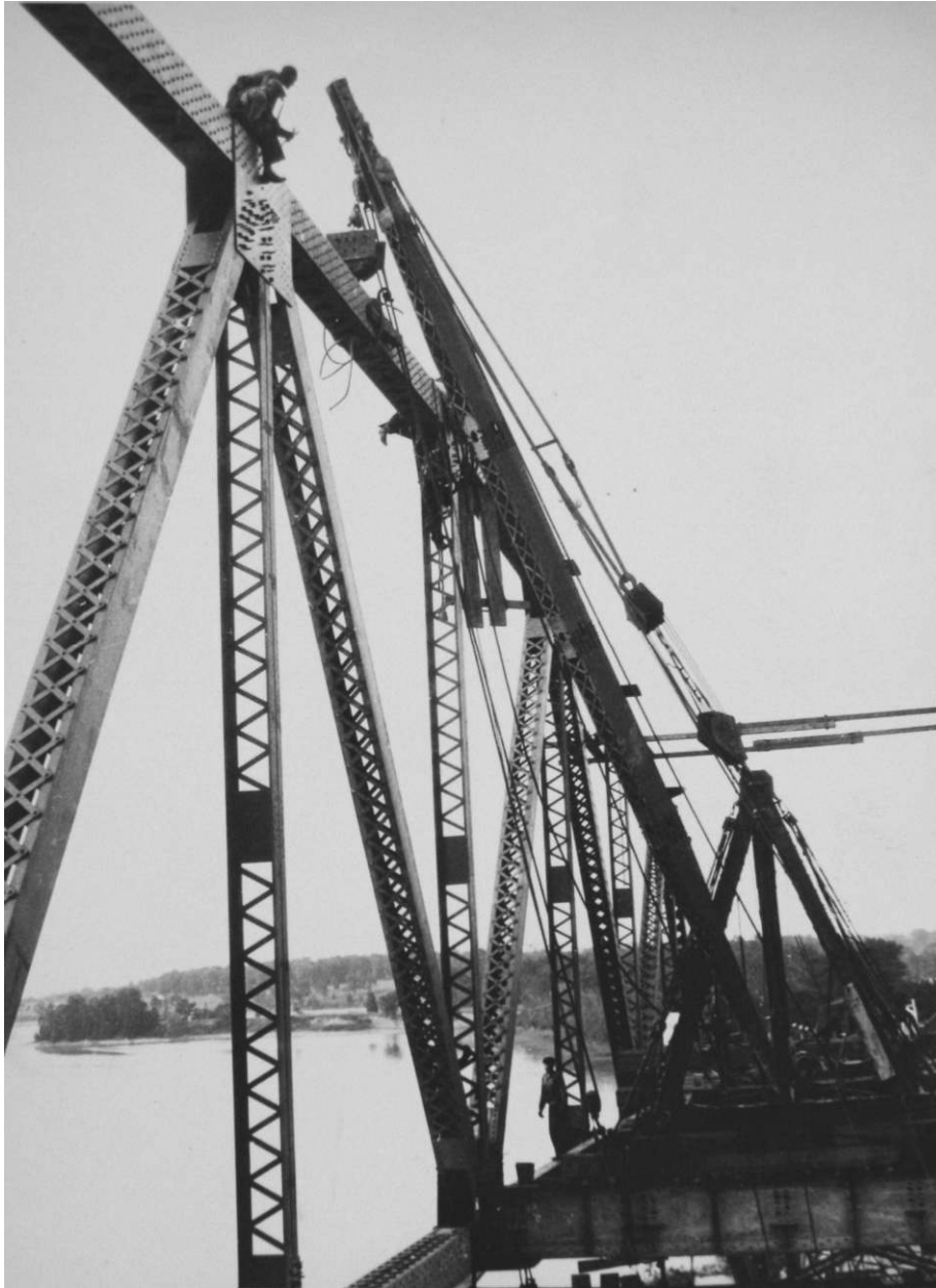
Figure 38. Workers joining the top chord on Span 7, mid-June, 1929. Image courtesy Vermont State Archives.
