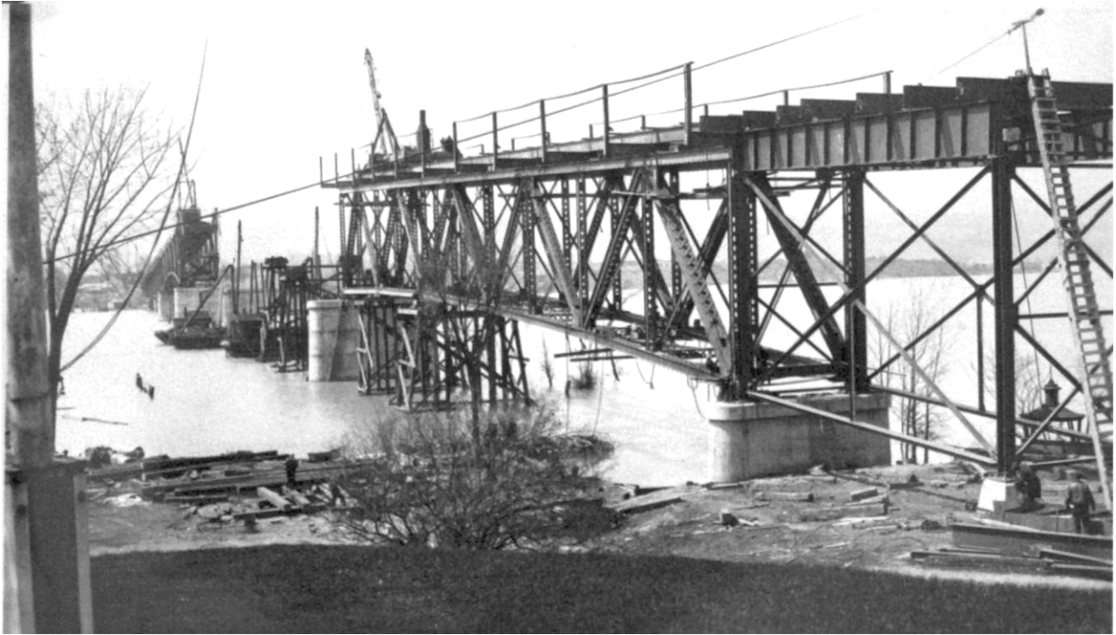
Figure 36. "Bridge from Barnes lawn," May 1, 1929. View shows the completed Span 9, with Spans 7 and 8 still to be built. Image courtesy Penfield Homestead Museum.
