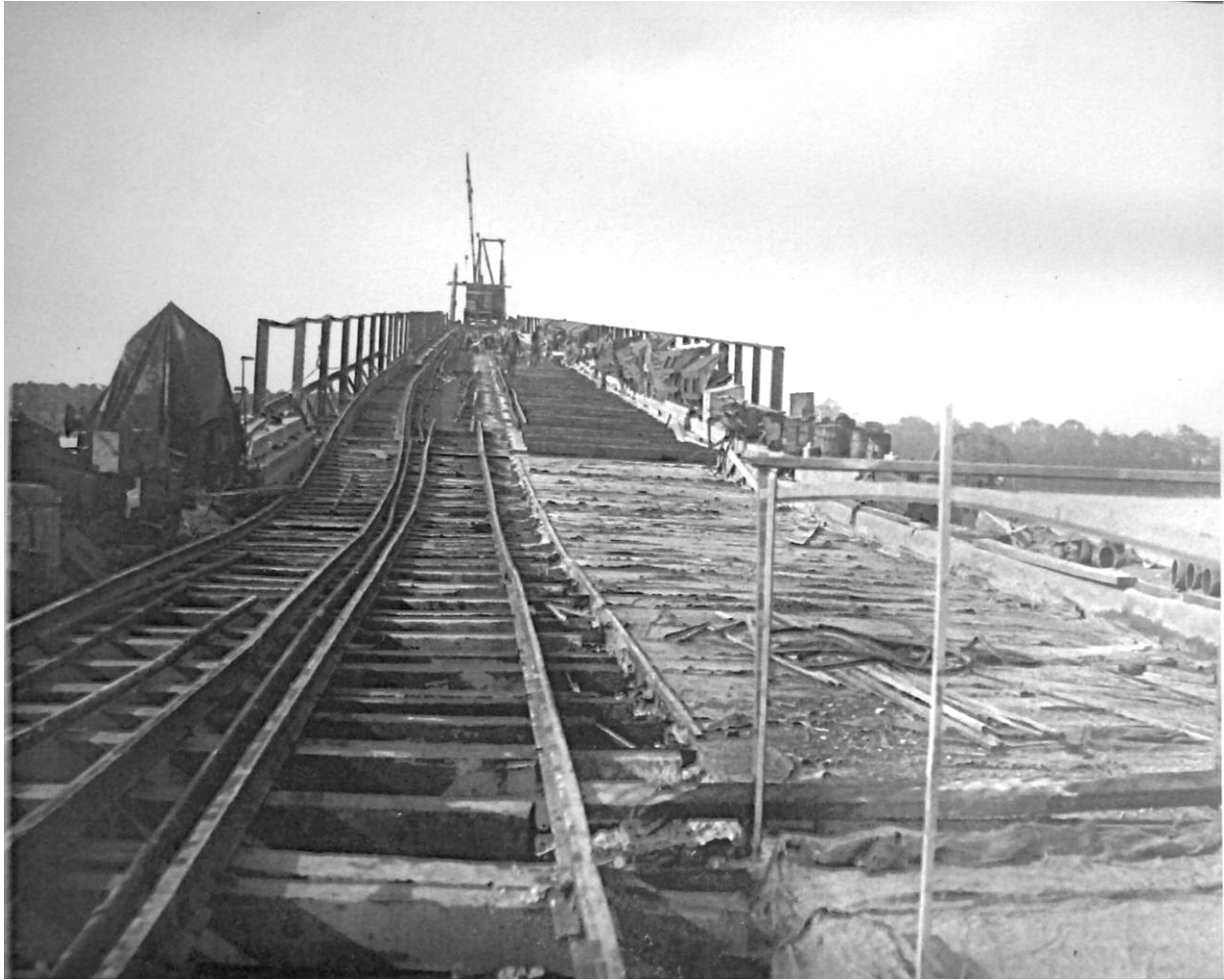
Figure 32. Concrete deck under construction on the New York end of the bridge, late April, 1929. The two sets of rails on the left side of the deck were used by Scott Brothers for their equipment and by American Bridge for their traveling derrick, which was still in use building Span 7. Image courtesy Bill Bodette.
