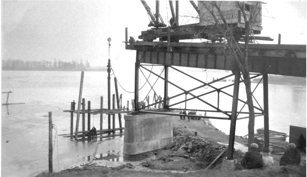
Figure 20. "American Bridge Company's traveling derrick at end of New York viaduct, Pier 3, driving piles for first temporary bent," December 28, 1928. Image courtesy Penfield Homestead Museum.
