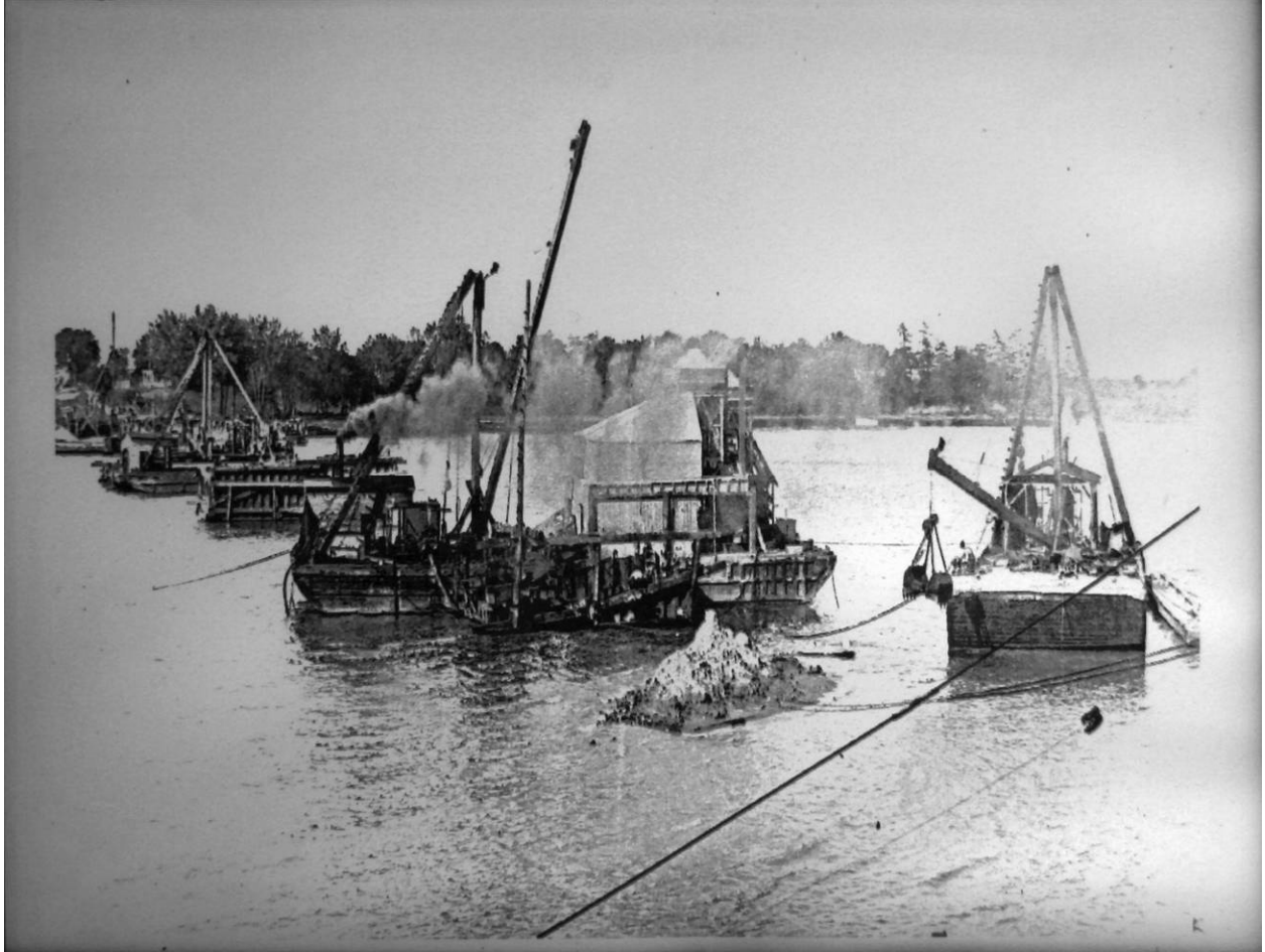
Figure 15. Pier construction by the Merritt-Chapman and Scott Corporation, summer 1928. Shows a derrick clamshell excavator and a floating cement plant on the nearest barges. Image courtesy Bill Bodette, Crown Point, New York.
