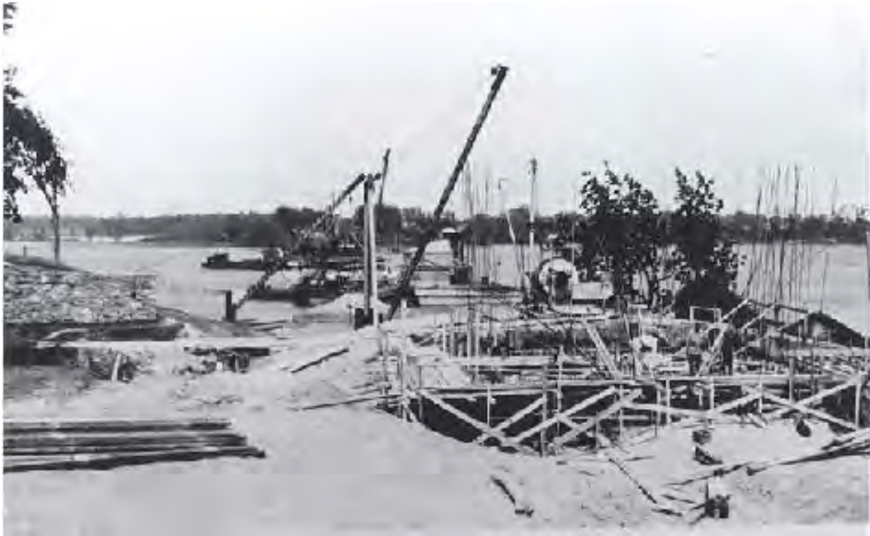
Figure 16. Construction of the New York abutment and piers by the Merritt-Chapman and Scott Corporation, showing proximity of the southeast bastion of Fort St. Frederic at left. Image courtesy Crown Point State Historic Site, Crown Point, New York.
