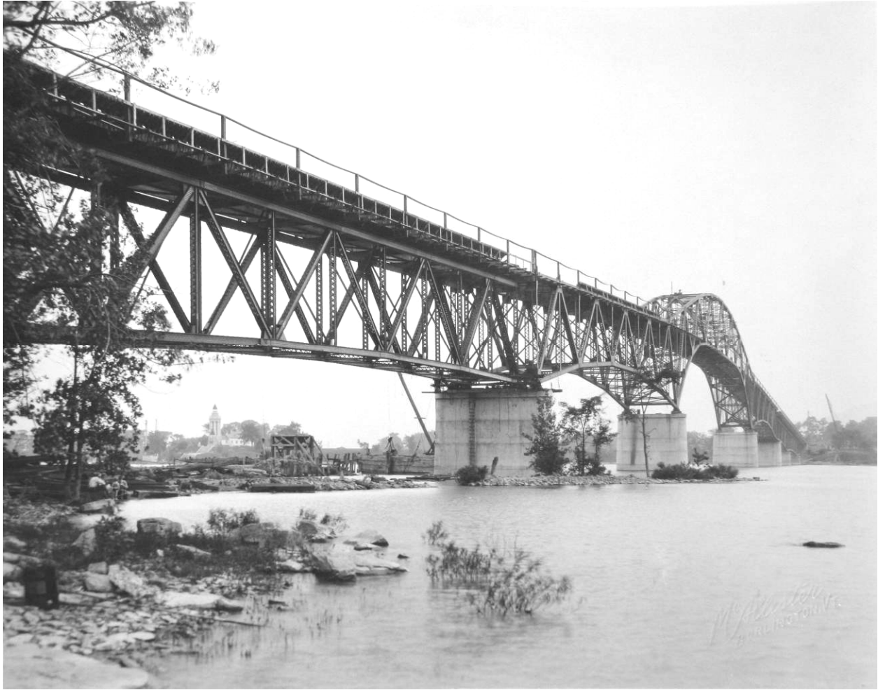
Figure 43. View of the almost completed bridge, west side, from Vermont, showing the temporary rail structure for the deck construction still in place, July 1929. The Champlain Memorial lighthouse is just visible in the distance at left. Image courtesy Vermont State Archives.
