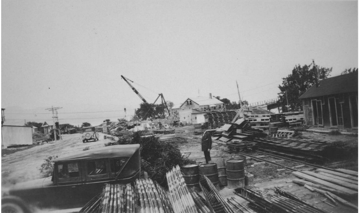
Figure 34. View of the staging area for the Scott Brothers Construction Company south of the bridge on the New York end. Shows the temporary rail line used to bring materials and scaffolding stacked in front of the company storehouse, at right. The bridge toll house is under construction in the distance. The road at left was the original entrance to the Crown Point Reservation. Image courtesy Vermont State Archives, Middlesex, Vermont.
