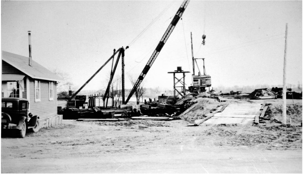
Figure 17. "General View of American Bridge Company's stiff leg 110' beam derrick and traveling erecting derrick just ready to go on first span of viaduct," December 21, 1928. Image courtesy Penfield Homestead Museum, Ironville, New York.
