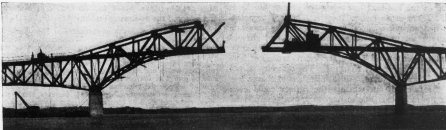
FIG. 8—ERECTION OF MAIN SPAN
