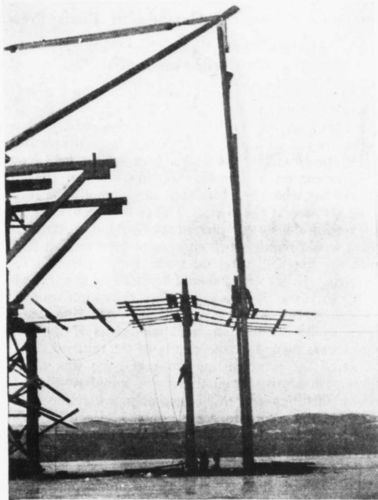
FIG. 7—DRIVING 140-FT. FALSEWORK PILING WITH
