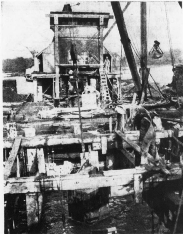
FIG. 3—POURING CONCRETE SEAL FOR DEEP COFFERDAMS WITH BOTTOM-DUMP BUCKET
