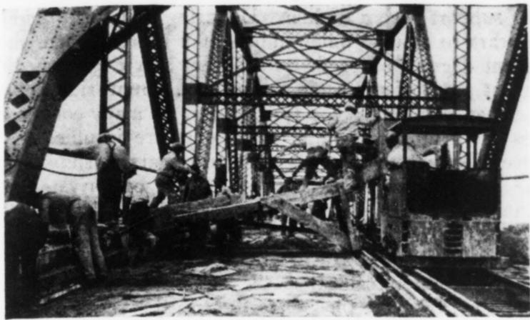
FIG. 6—POURING SIDEWALK AND CURB
