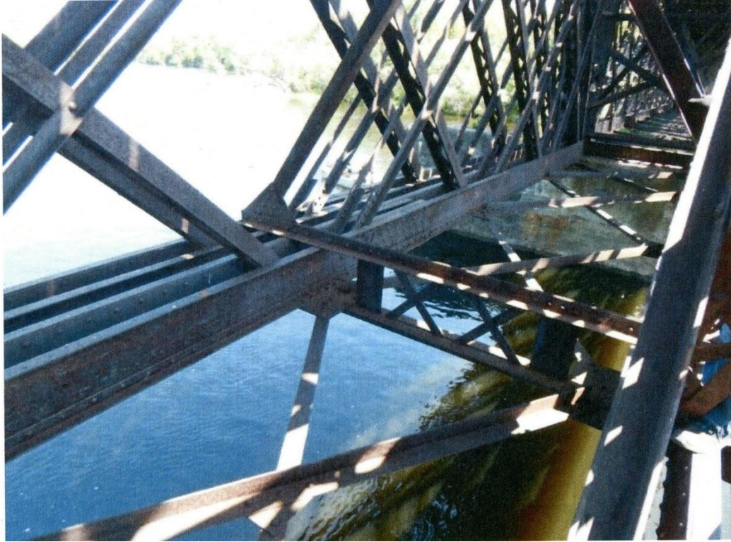
Photo 5. View of the NYOG Bridge No. 80, Span 2, showing the lower chords and laterals (Parsons 2015 Inspection Report, Photograph 31, page 39).
