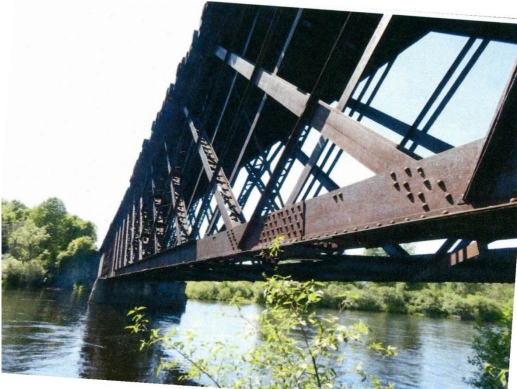
Photo 4. View of the NYOG Bridge No. 80 east (south) elevation, Span 3, showing the single truss. (Parsons 2015 Inspection Report, Photograph 28, page 38).
