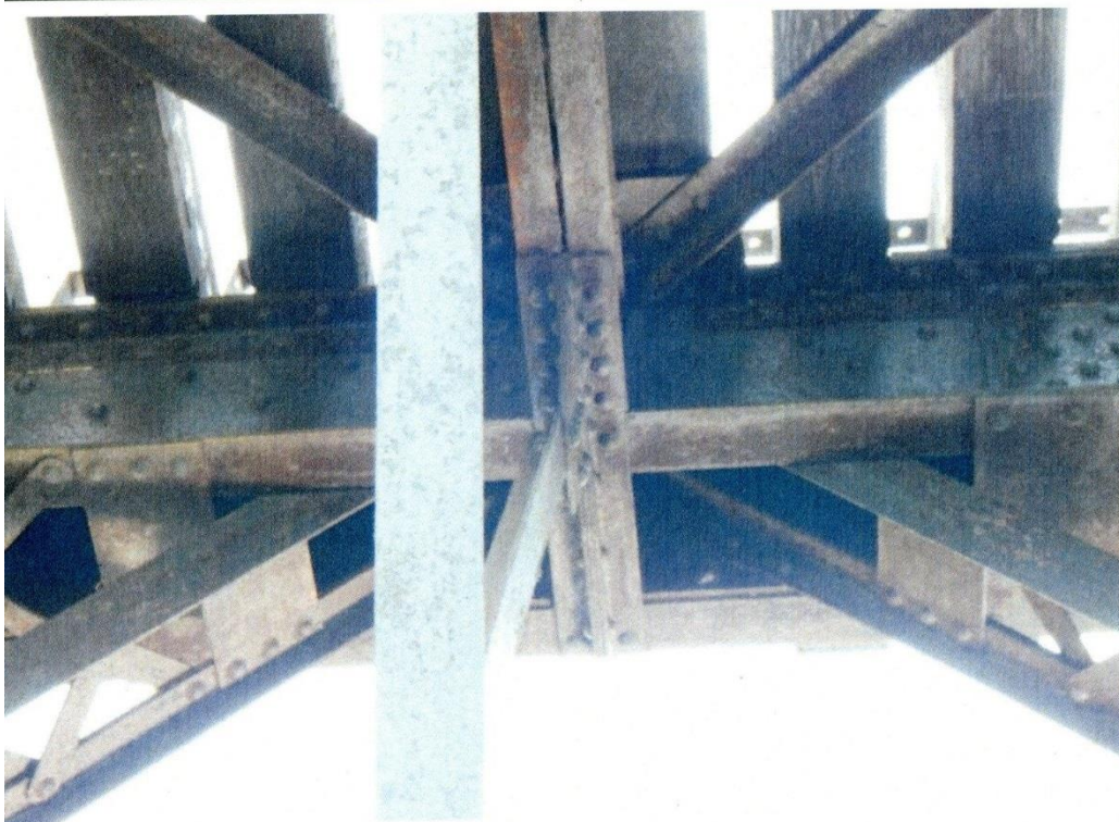
Photo 8. View of the NYOG Bridge No. 80, Span 3, showing the upper chord and laterals (Parsons 2015 Inspection Report, Photograph 30, page 39).
