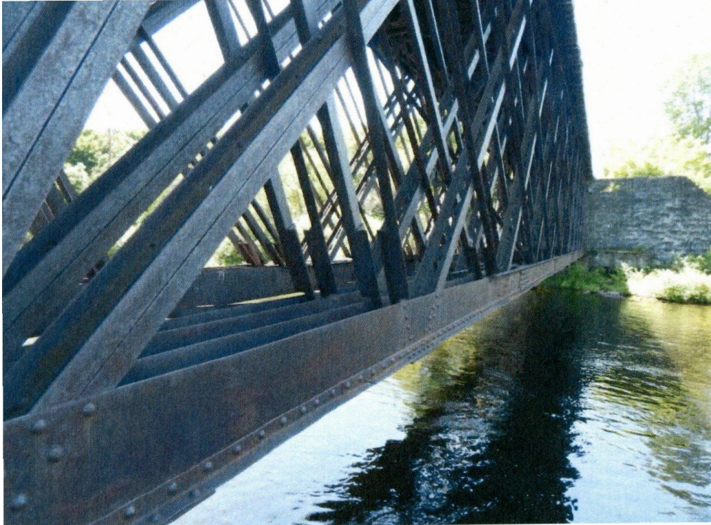
Photo 3. View of the NYOG Bridge No. 80 west (north) elevation, Span 2, showing the double truss. (Parsons 2015 Inspection Report, Photograph 28, page 38).
