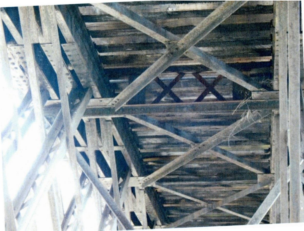
Photo 6. View of the NYOG Bridge No. 80, Span 2, showing the upper chords and laterals (Parsons 2015 Inspection Report, Photograph 34, page 41).
