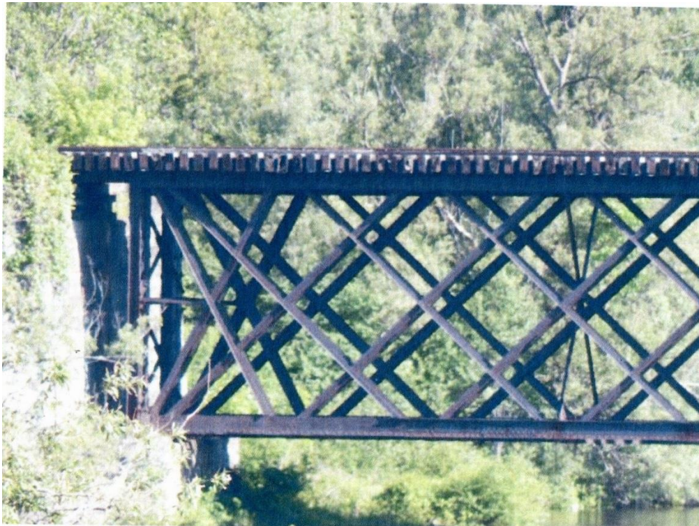
Photo 2. View of the NYOG Bridge No. 80 east (south) elevation, Span 2, at the south abutment. The bridge is a Hilton lattice truss, featuring quadruple intersection diagonals and end posts acting as tension hangers (Parsons 2015 Inspection Report, Photograph 3, page 24).
