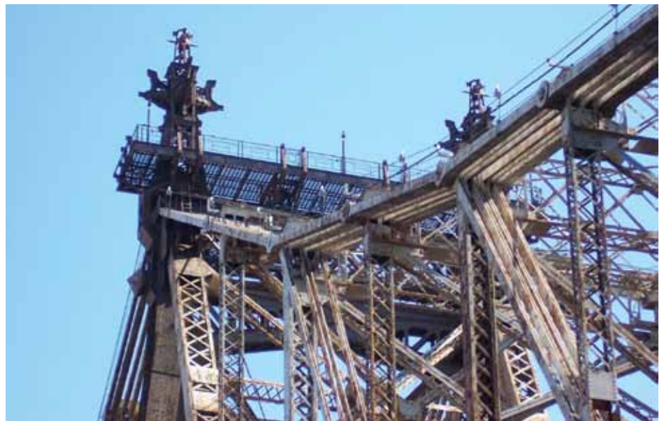
Queensboro Bridge looking to top of tower showing Links, Pinnacle, etc.
