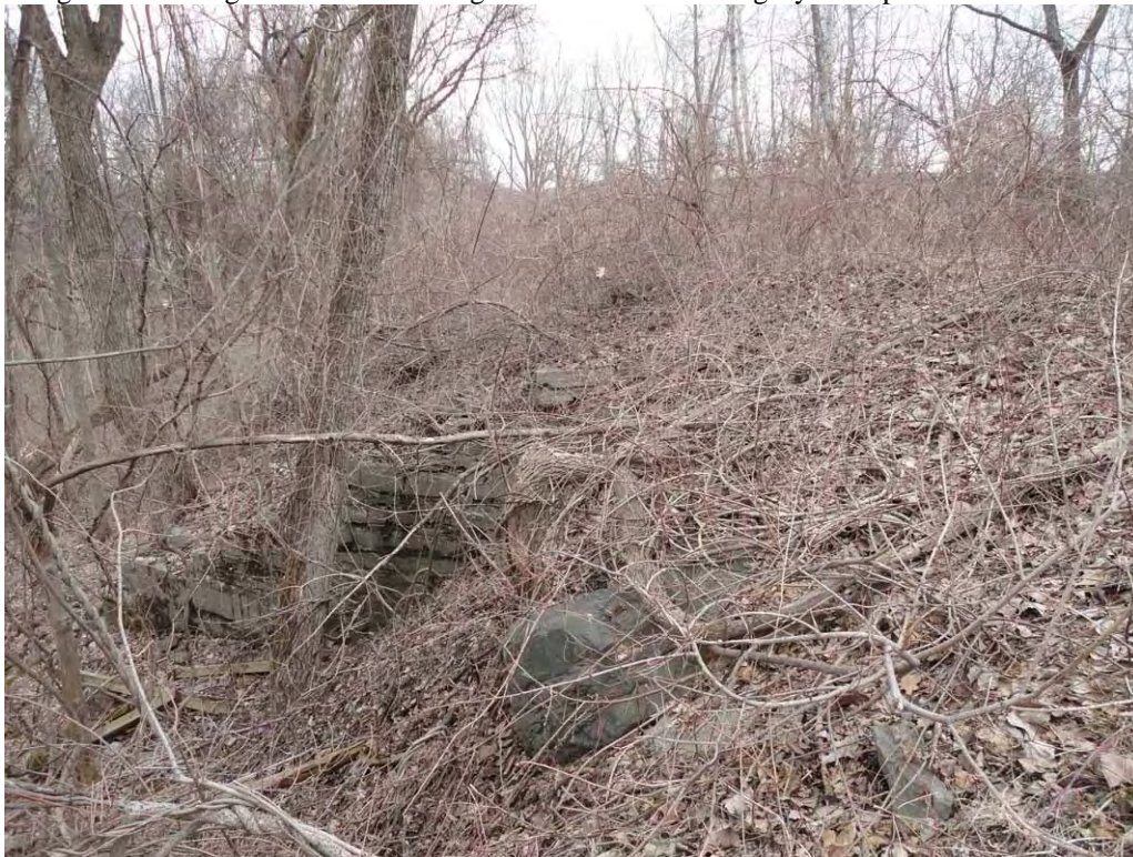
Photo 43. Structure 80, Blue stone head wall culvert, constructed c.1868, facing south. This structure was determined to be ineligible for listing on the National Register due to loss of integrity to its period of construction.
