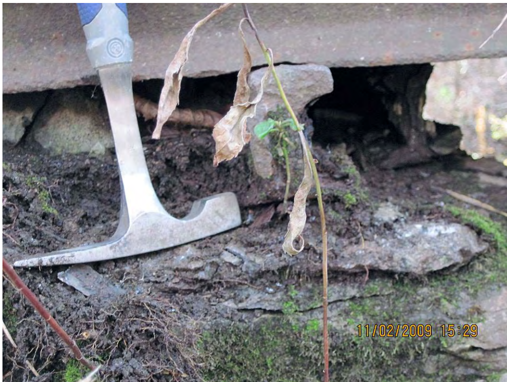
Photo 78. Detail showing section of rails used for decking.
