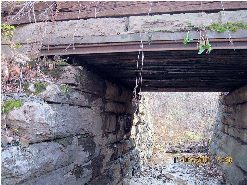
Photo 77. View north showing details of abutments and steel rail-supported deck.
