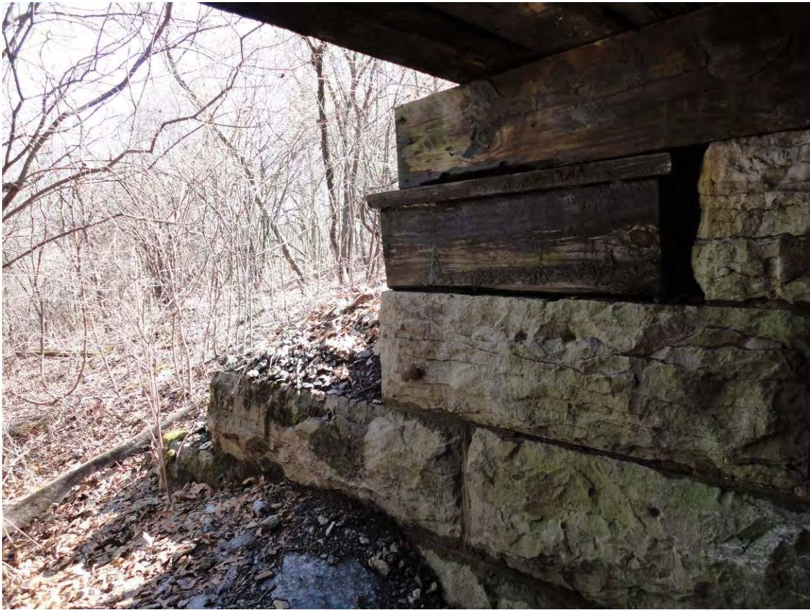
Photo 73. View northeast, showing typical timber and stone abutment detail.
