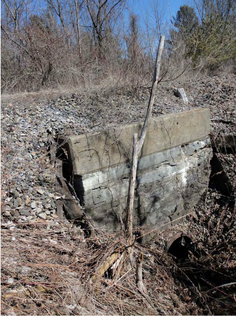
Photo 28. Structure 59, Limestone and concrete headwall with iron pipe, constructed c.1890, facing northeast. This structure was determined to be ineligible for listing on the National Register because it lacks distinguishing characteristics.
