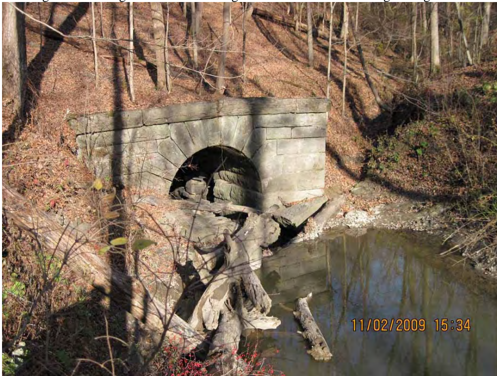
Photo 34. Structure 66, Stone headwall, constructed c.1868, facing northeast. This structure was determined to be ineligible for listing on the National Register. While this headwall is intact, the north headwall and approximately 20 feet of the brick arch culvert were recently destroyed during hurricane Irene. The structure no longer retains integrity to its period of construction.
