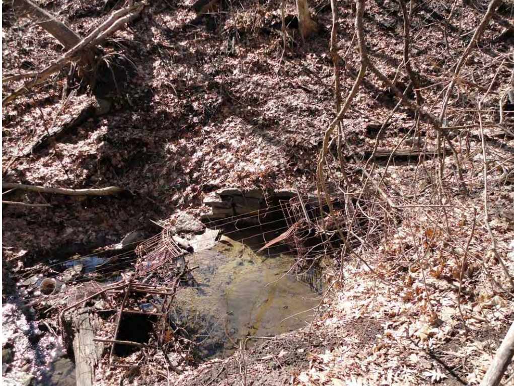
Photo 25. Structure 42, Blue stone head wall culvert, constructed c.1870, facing south. This structure was determined to be ineligible for listing on the National Register due to loss of integrity to its period of construction.
