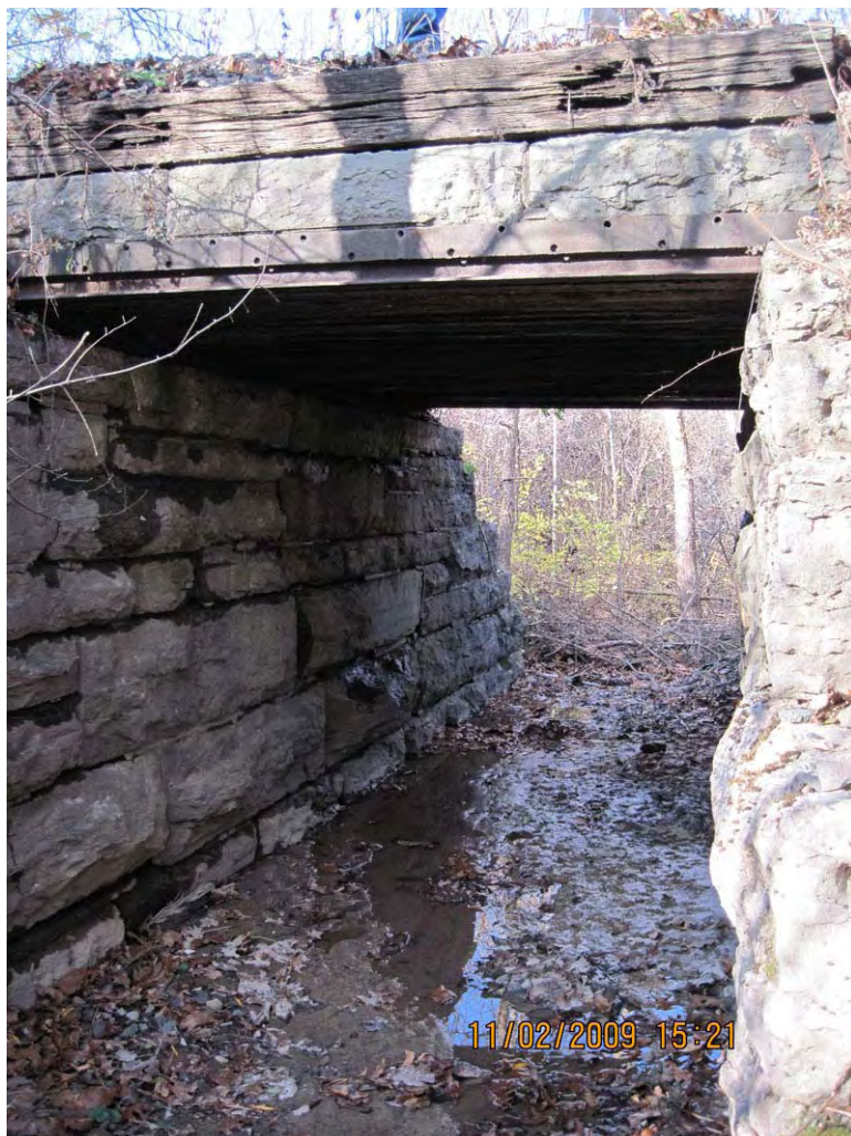
Photo 35. Structure 67, Culvert with stone walls, constructed c.1890, facing southeast. This structure was determined to be eligible for listing on the National Register under Criterion C.
