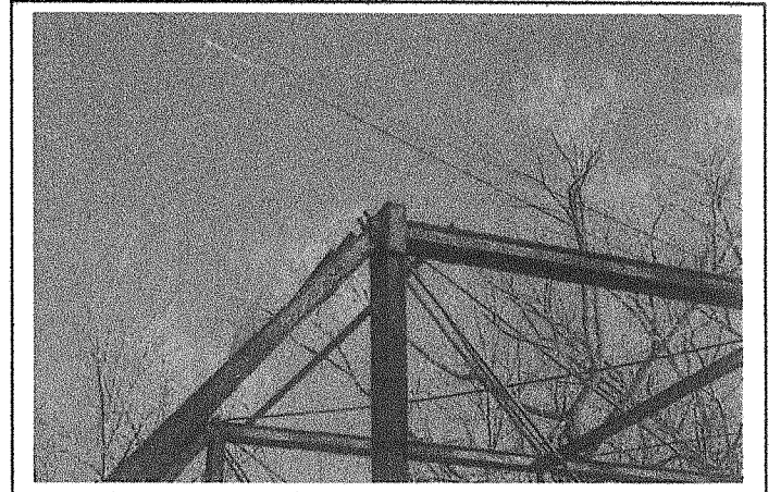
U5 South End post and upper chord detail
