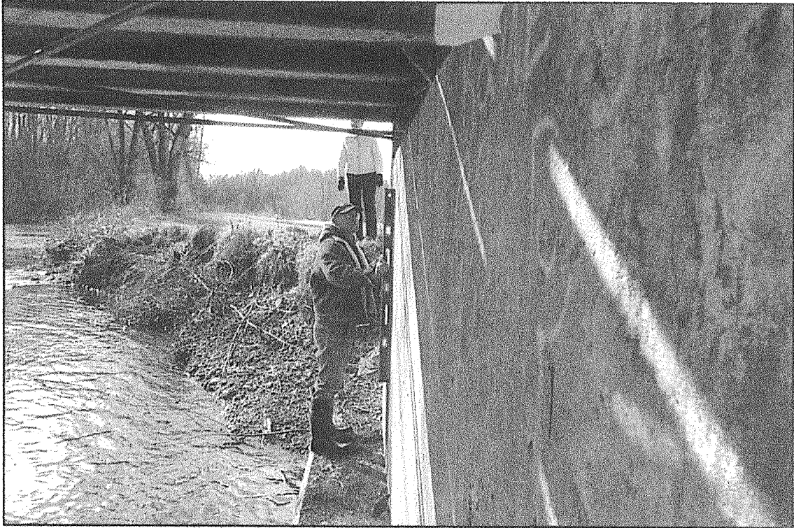
West Abutment looking southerly
