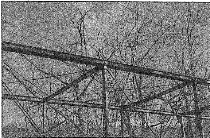
U4 Upper Chord Connection and cross bracing
