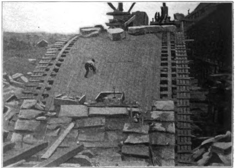
FIG. 4. CENTERING AT HOOSICK JUNCTION.
