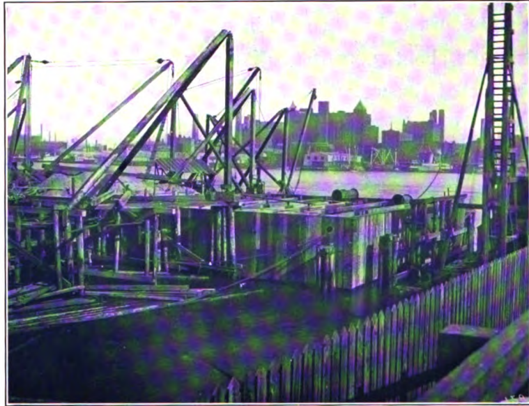
THE CAISSON ANCHORED AND READY TO SINK
