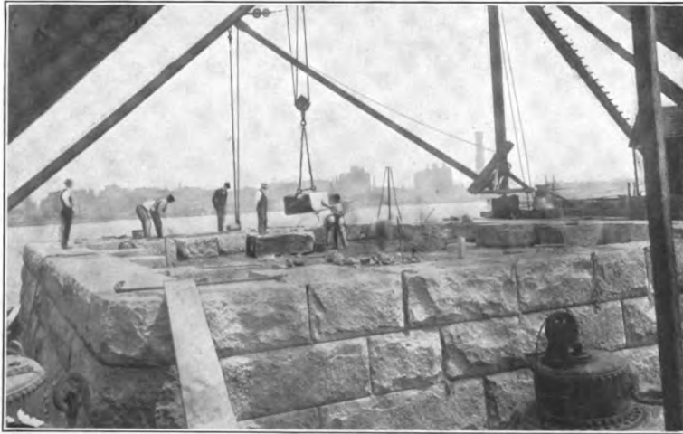
PLACING THE MASONRY ON A CAISSON
