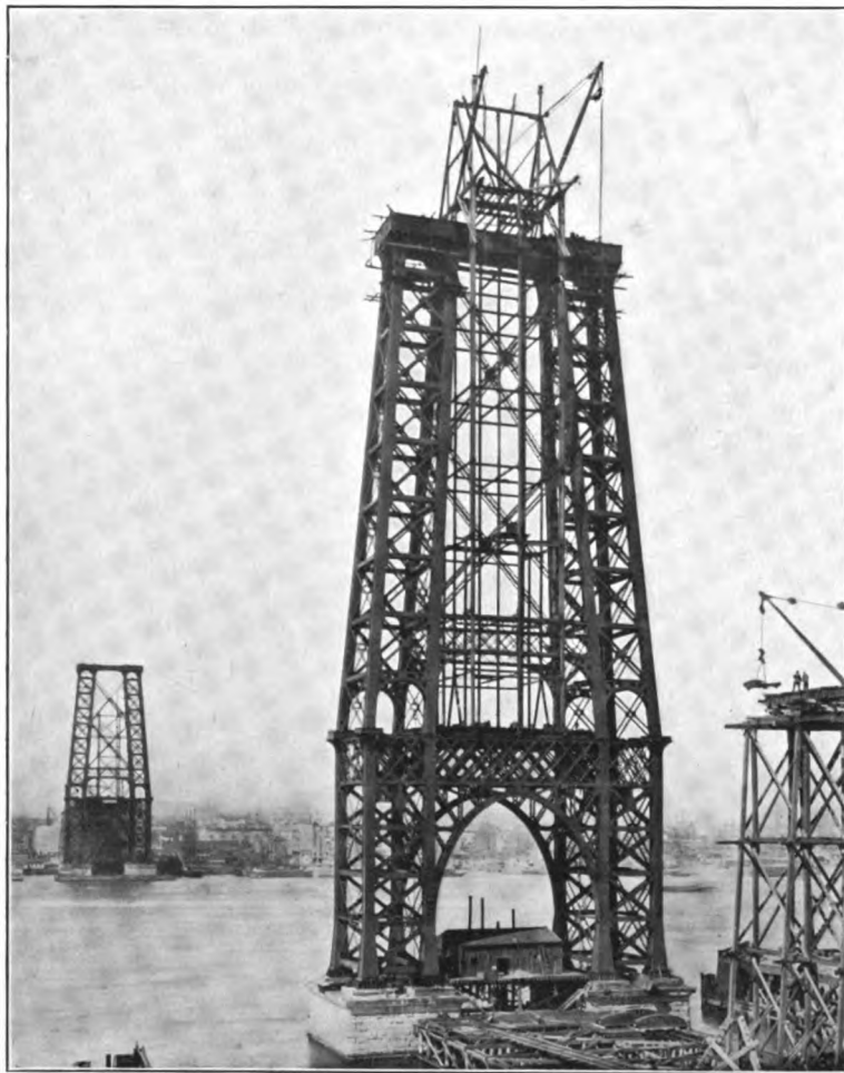
ALL IS THEN IN READINESS TO RECEIVE THE CABLES
