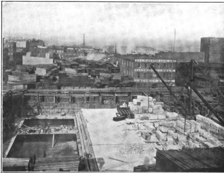
THE FOUNDATIONS FOR AN ANCHORAGE
