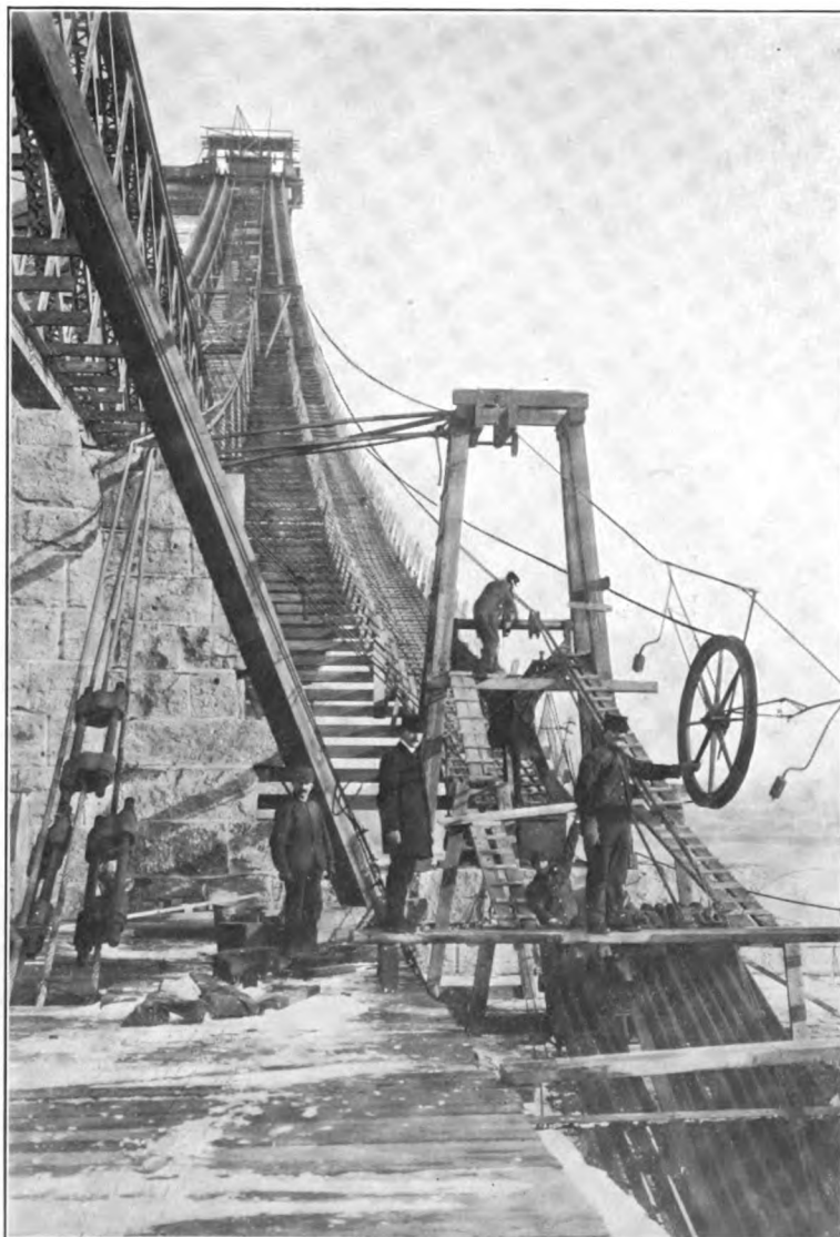
THE "TRAVELER" THAT SPINS THE CABLES
