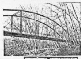
Elevation looking southwest-west end
