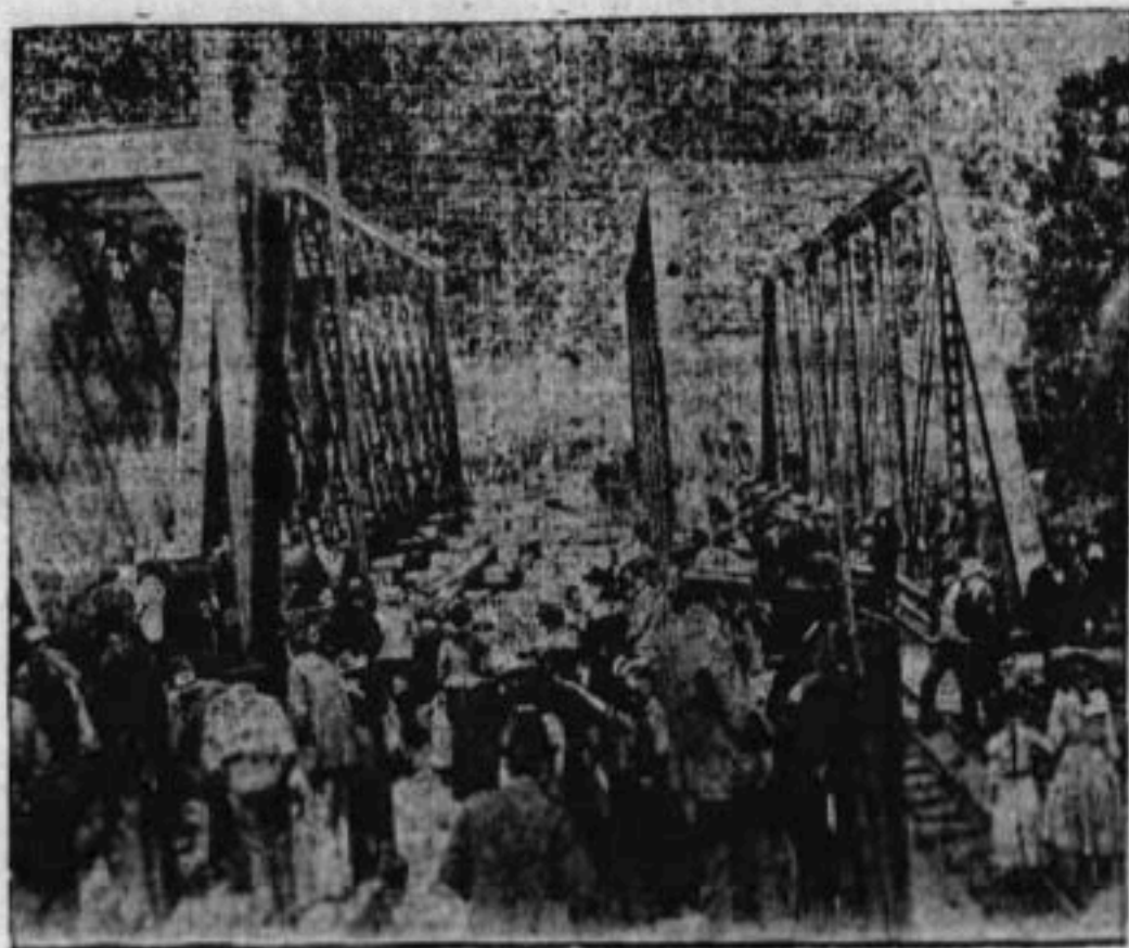
The bridge on the left is the new bridge ready for traffic.
