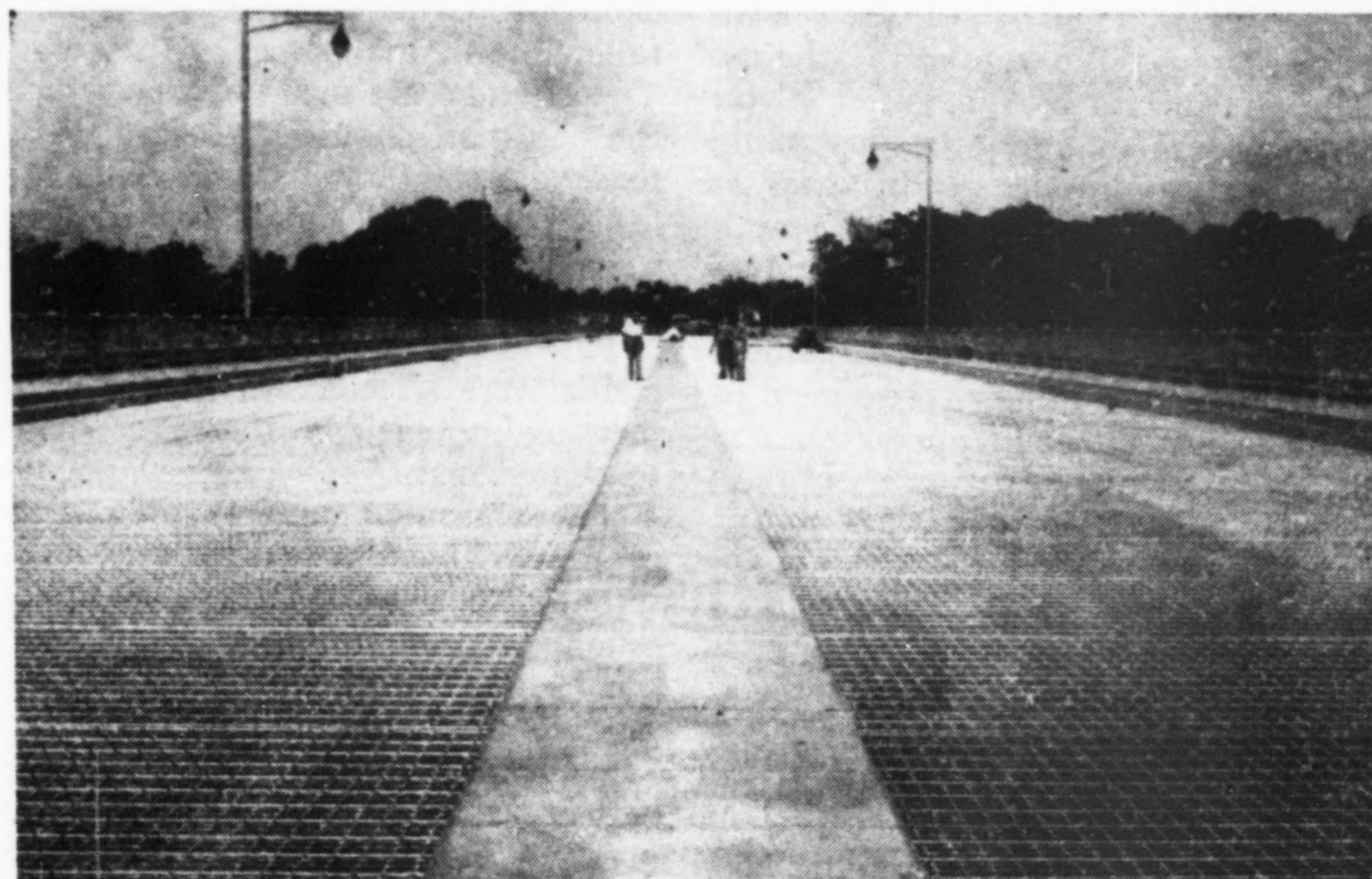
OPEN STEEL-GRID FLOORING for the two 26-ft. roadways—separated by a 4-ft. welded steel-plate—was adopted for its high strength-weight ratio, excellent drainage and low maintenance in the winter.
