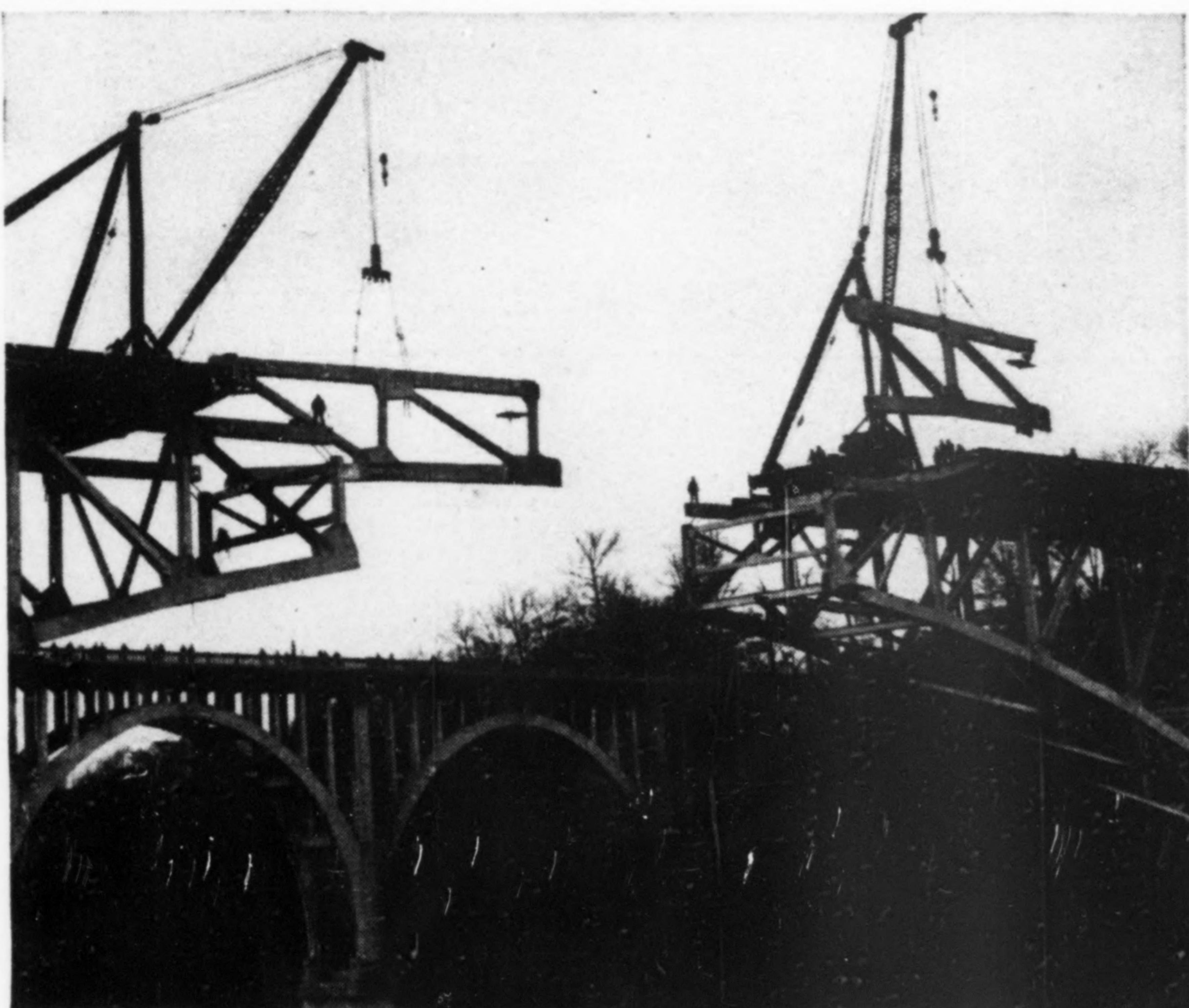
TRAVELLERS SWING 60-ft., 40,000-lb. sections of the suspended span into position (at top), for closure at the center of the middle span. Small gusset plates add beauty to the bridge by accentuating the constant-depth chords. (Akron Beacon-Journal photos)
