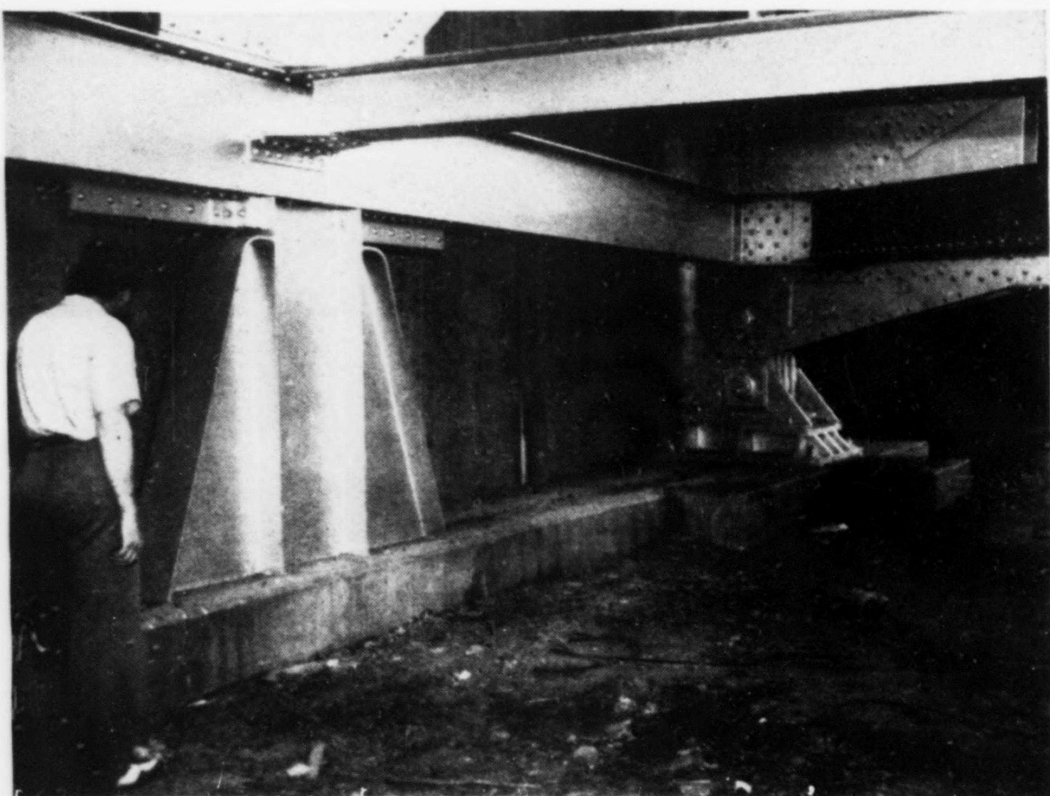
**WIND STRESSES** in the anchor spans are transmitted from the bottom chord lateral system to the abutments through a sliding support embedded in the center of the bridge seat. Truss anchorages, designed to permit expansion at both abutments are prestressed for a 500,000-lb. uplift.
