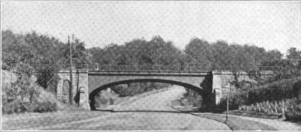
Fig. 1. Old East Boulevard Three-Hinged Steel Arch, Cleveland, O.
