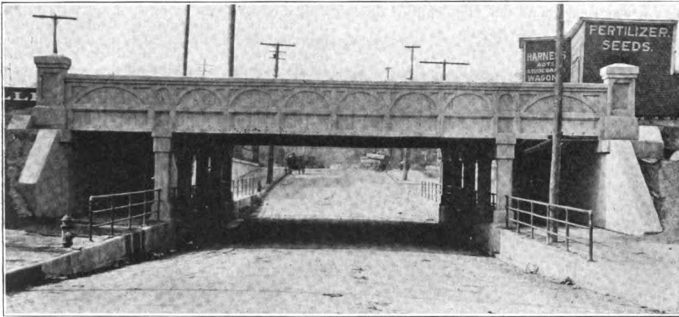
Fig. 7. Mayfield Road Bridge—Plate Girders Masked by Concrete.
