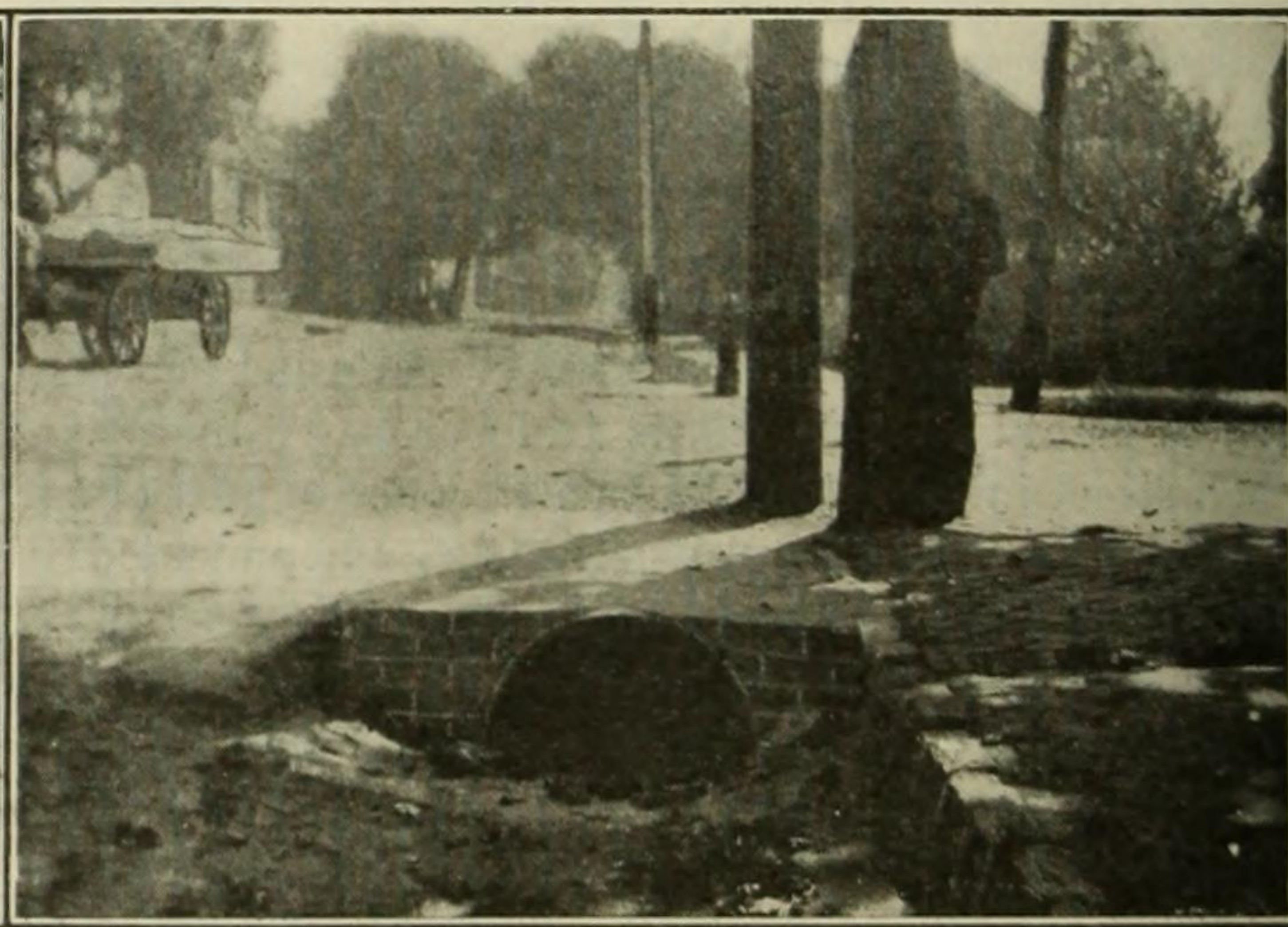
FIG. 2. NEW HALF-CIRCLE CORRUGATED CULVERT
