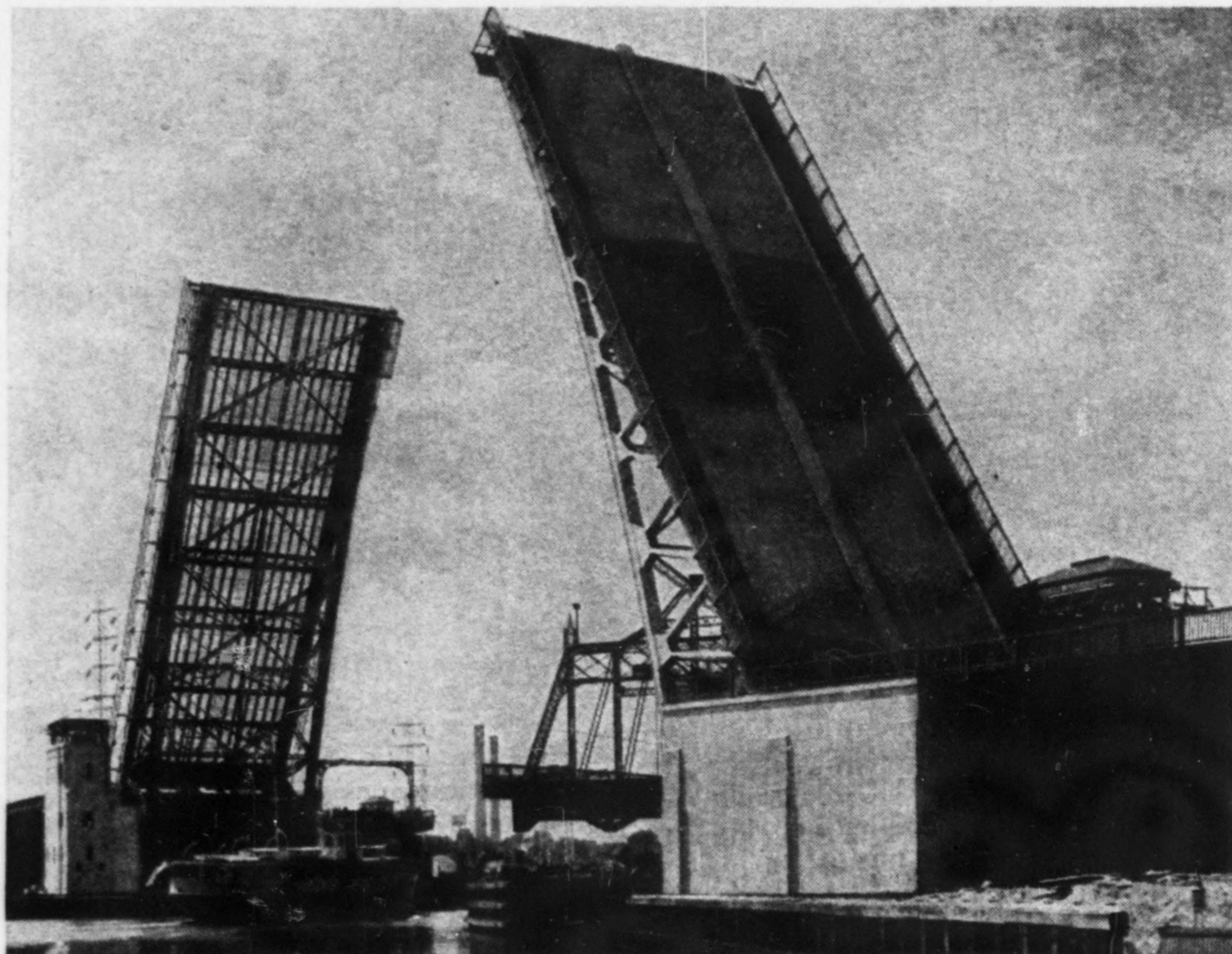
Fig. 4. How the long bascule with open-grid steel deck looked when completed. Old swing bridge adjacent is not being removed.
