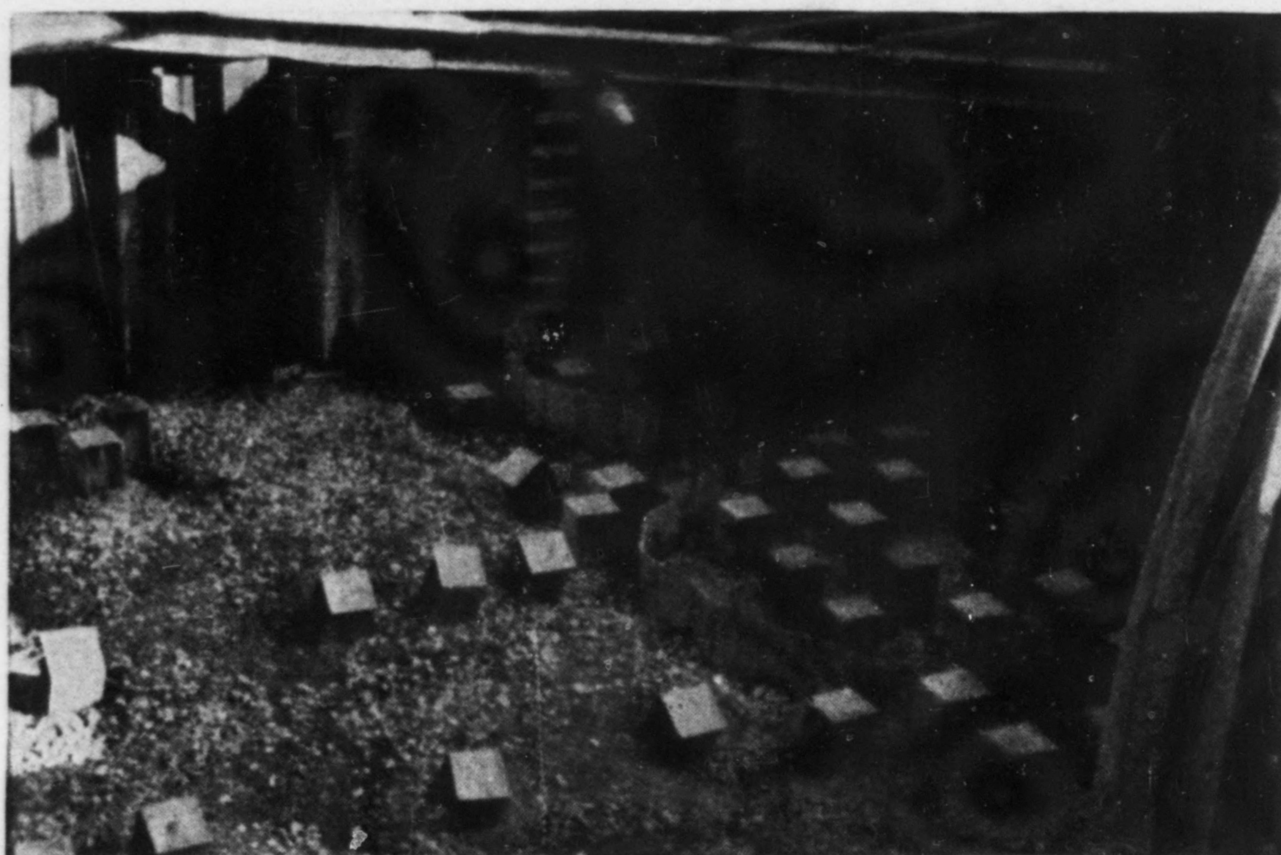
Fig. 3. H-beams driven to shale, and capped to distribute load on concrete support west pier after a circular sheetpile caisson scheme was abandoned.
