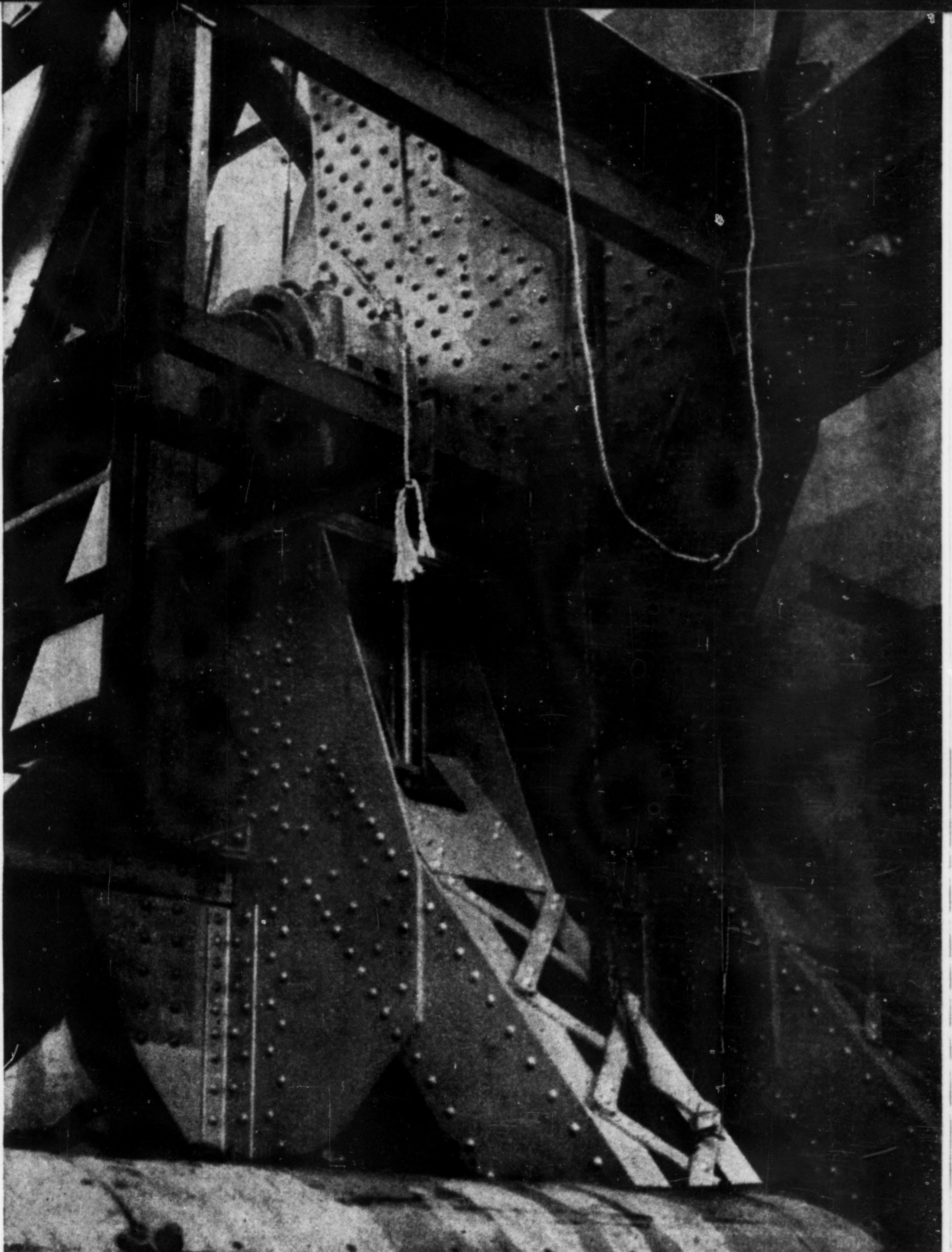
Fig. 2. Each 29-in. trunnion bearing carries 800-ton load of leaf and counter-weight. Chrome nickel steel is used for trunnion pinions and shafts, chrome vanadium for rack gears.
