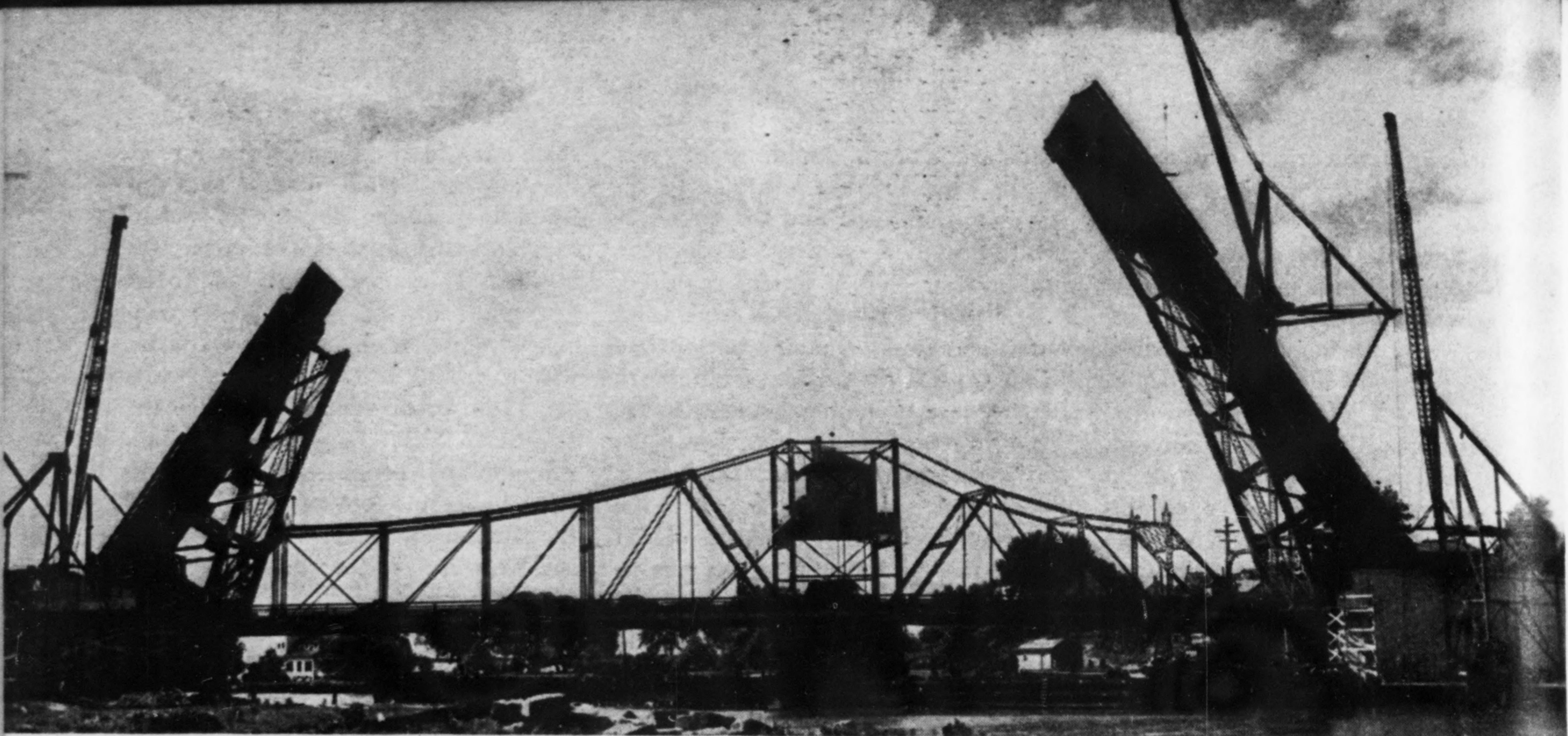
Fig. 1. At Lorain, Ohio, two derricks erect each bascule leaf to complete record 333-ft. highway span.
