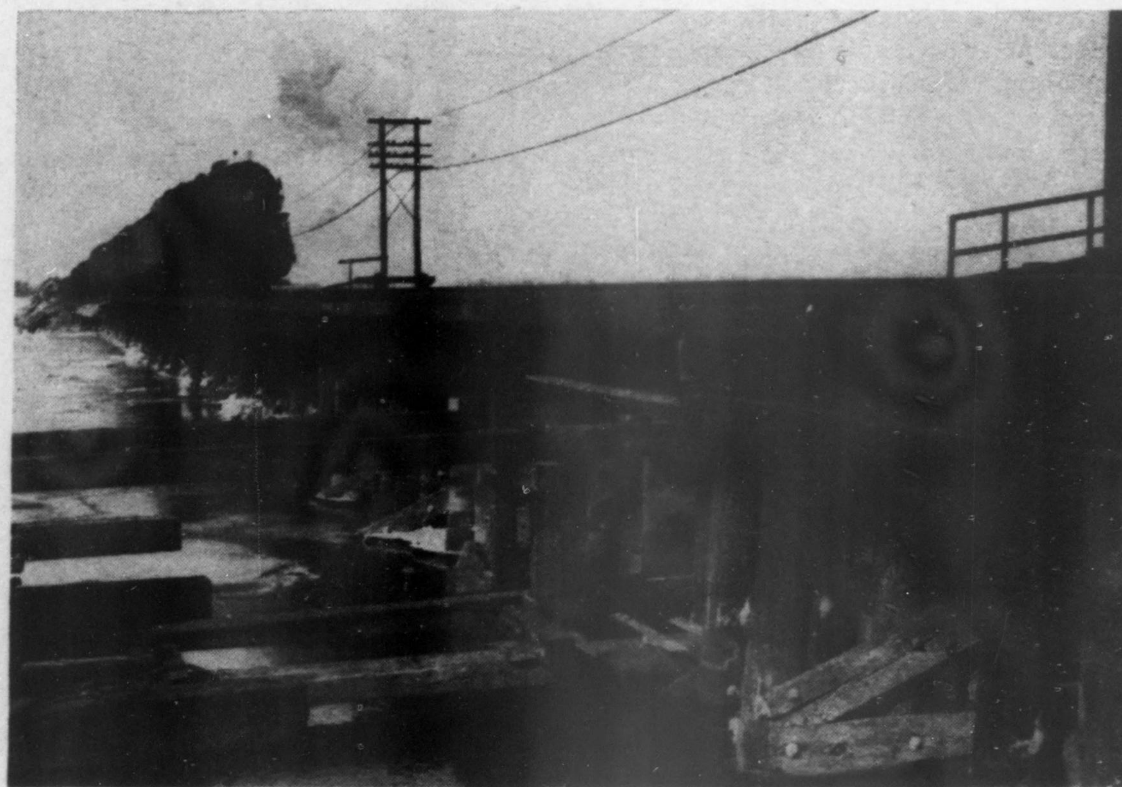
Bridge 68 before work was started in 1944, looking west
