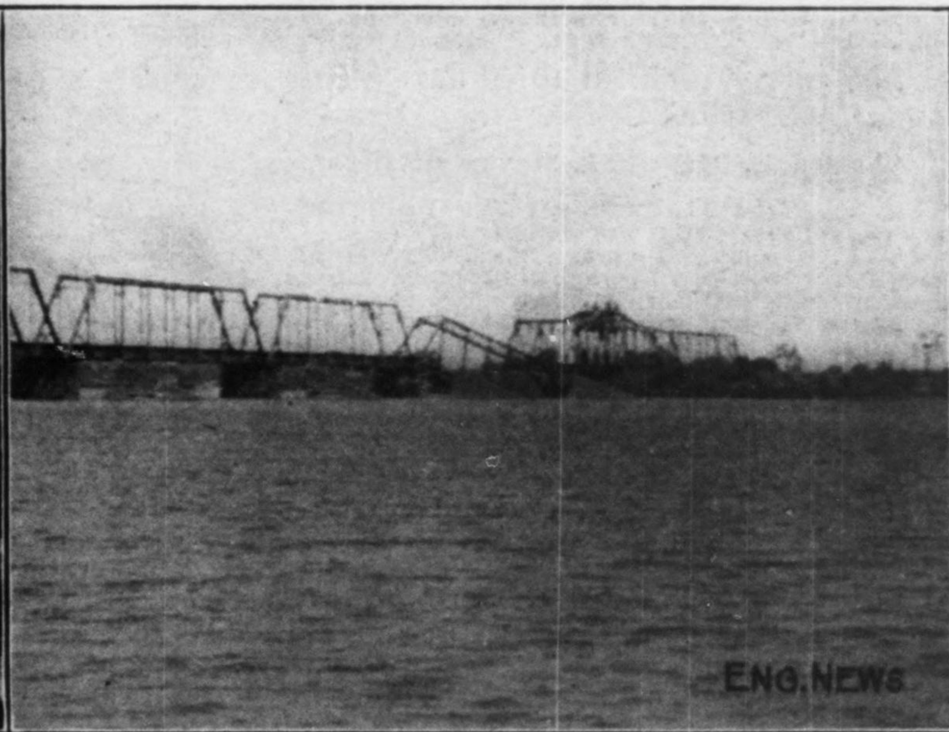
WHEELING & LAKE ERIE RY. BRIDGE AT TOLEDO; SPAN PUSHED OFF PIER BY COLLIDING BARGE
