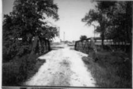
Portal view looking south
