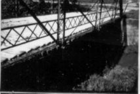
Lower chord connection (southwest)
