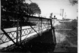
Counter crossing looking southwest
