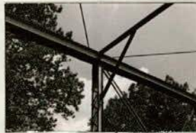
Detail view top joint @ vertical post - looking north
