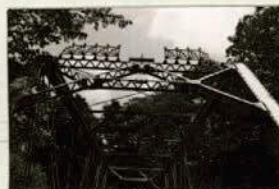
Detail view west portal frame looking east
