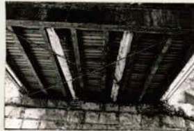
Underside view steel beams & sub- decking
