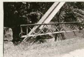
Detail view @ railing end
