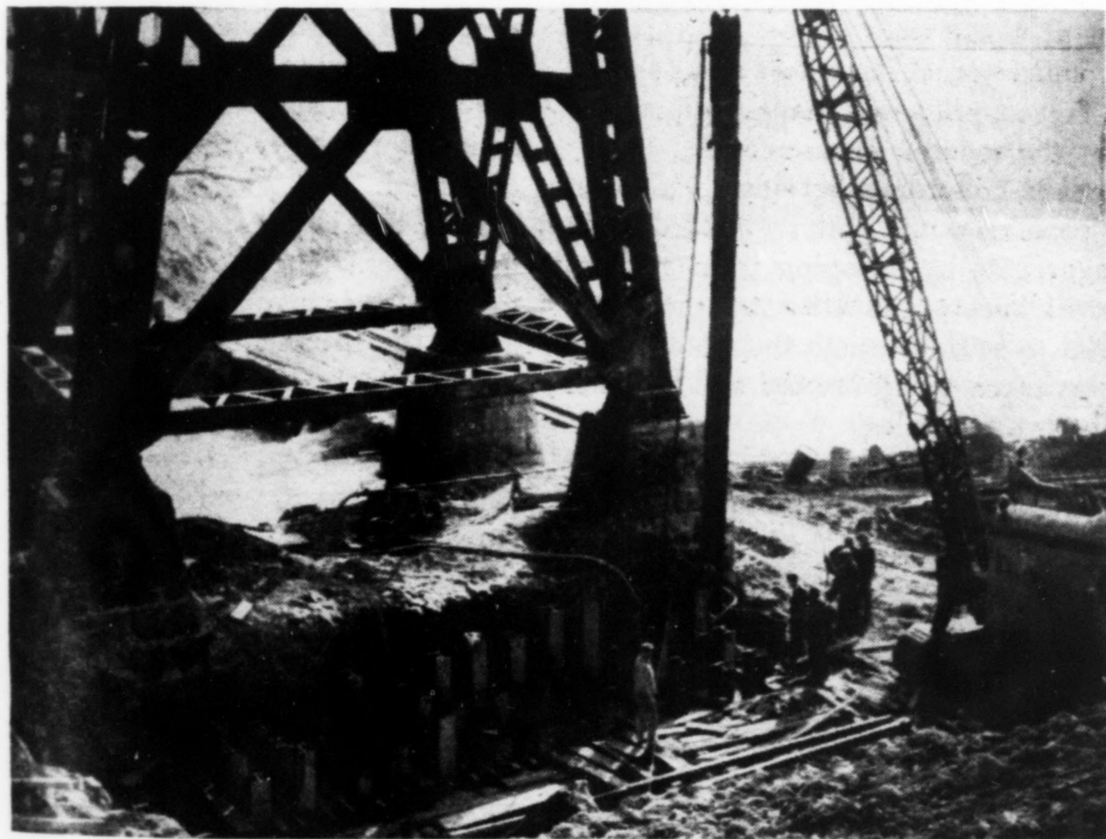
Fig. 6. Pier 3 was constructed immediately adjacent to existing footings by driving H-piles to bearing materials and extending them upward to near the bridge
