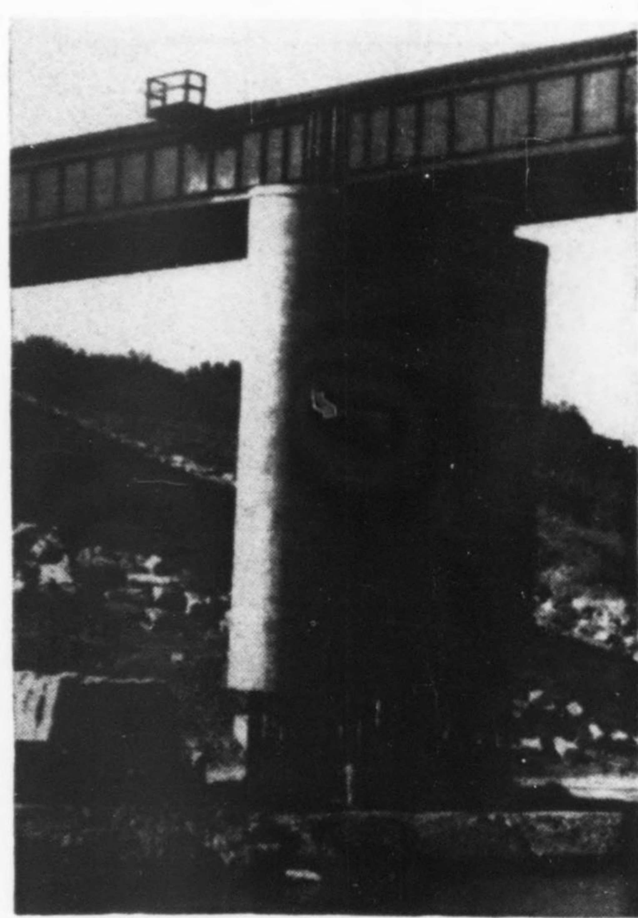
Fig. 10. Excavation below the ground line after the upper section was completed temporarily exposed the bearing piles of Pier 3, while under full load.
