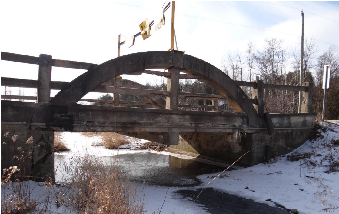
Figure 2: East elevation of the subject bridge, looking west
