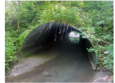
CSP Culvert: Jibb Road
