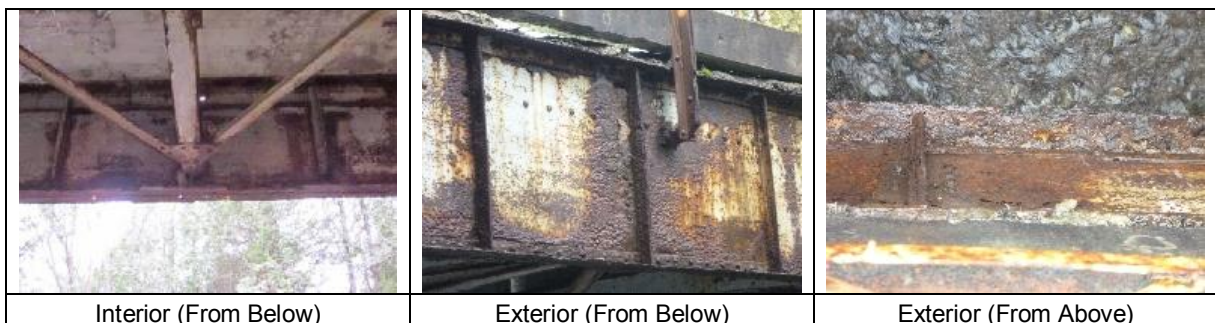
Figure 2 – Critical Location on South Girder
